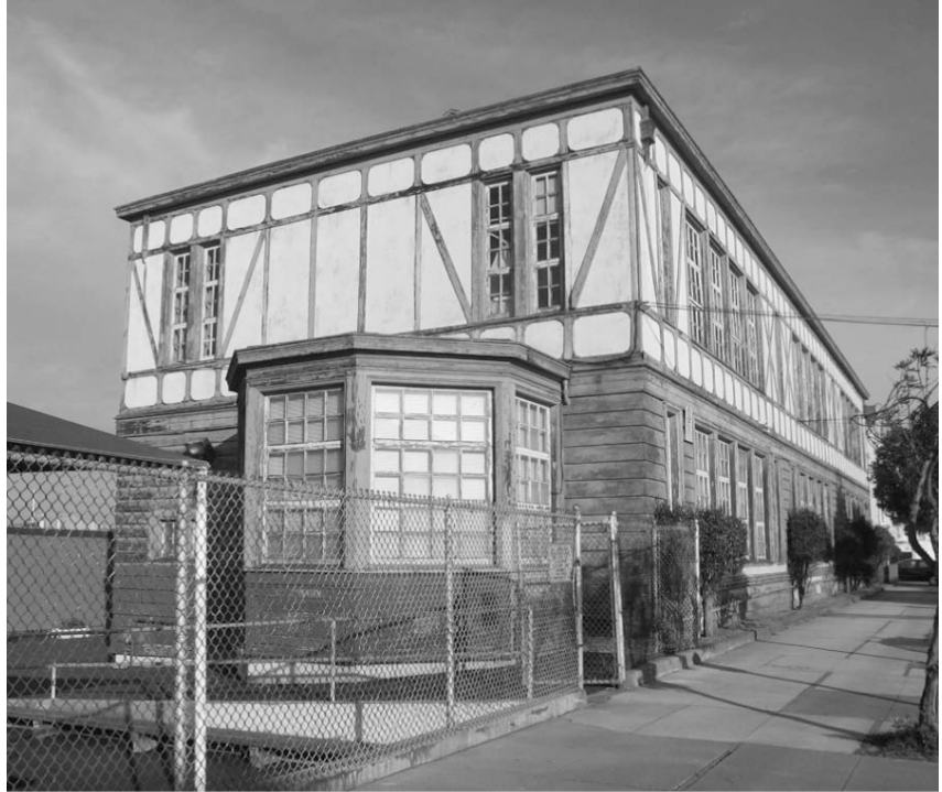
Francis Scott Key School Annex.
