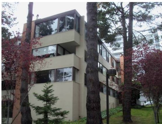
Left: 66 Cleary Court residential tower designed by Jones & Emmons (1964). Right: Across the street, at 85 Cleary Court, is a complex of six three-story, 12-unit buildings designed by Claude Oakland (1963). Common alterations include the enclosing and glazing of both the low-rise buildings and the tower. The middle-unit (right) retains its original open-air balcony. Photos: Aisha Rahimi; Mary Brown, San Francisco Planning Department
