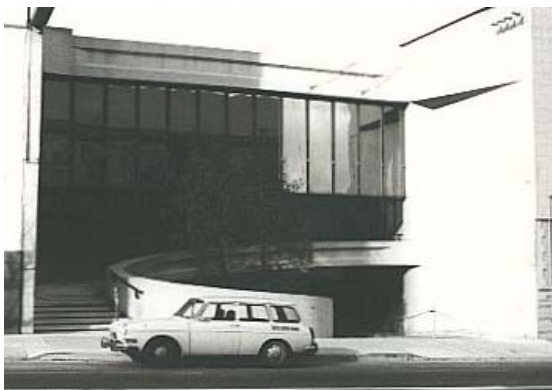
Left: Designed by Neill Smith Assoc., the Bank of America branch bank at 1660 California Street features a highly unusual circular stairway, an open deep set-back, concrete construction, floor-to-ceiling plate glass windows, and a parking garage. Although extant and retaining high physical integrity, the welcoming exterior space was subsequently fenced off. Source: 1976 Architectural Survey
