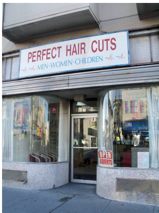
LEFT: The façade of this 1918 mixed-use building on Mission Street was fully remodeled in 1941. It features rare extant curved windows and bulkheads, topped with horizontal, extruded metal bands. The bulkhead tile work and front door were replaced in 1963. BELOW: Built in 1949, this free-standing Excelsior District commercial building, strongly reflects the nautical influences of the Streamline Moderne style. The flat roof and ribbon windows appear influenced by the International Style. The building is an early design by San Francisco-based Modern architect Mario Ciampi. Ciampi also designed several Midcentury Modern commercial and mixed-use buildings in the Excelsior District. Photos: Mary Brown, San Francisco Planning Department.
