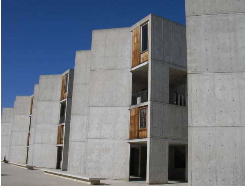
Top Left: Louis Kahn's Salk Institute, San Diego, California, built 1959-1965. Kahn's Brutalist masterwork features interstitial service floors, located between the working floors, to accommodate technological upgrades. The complex consists of two rows of low-rise concrete offices and laboratory spaces. Photo: Mary Brown, San Francisco Planning Department
