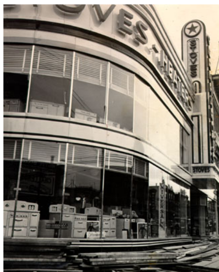
Left: The rectangular plan commercial building at 2205 Mission Street (extant), was completely remodeled in 1937-38 drawing from the Streamline Moderne idiom. The building’s corners were rounded, continuous corner windows installed, rustic wood cladding covered with smooth enamel iron panels, speed lines applied near the roofline, and the entrance renovated to include a recessed vestibule, terrazzo paving, and marquee/tower. Photo: San Francisco History Center, San Francisco Public Library
