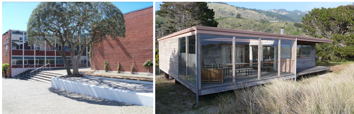
Electrician's Union, Local 6, 55 Fillmore Street, San Francisco Photo: Mary Brown, San Francisco Planning Department
