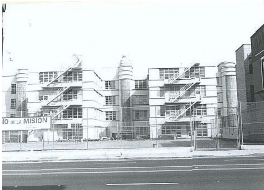
LEFT: The Mission campus of City College of San Francisco, constructed as a high school in 1939. The firm Masten & Hurd incorporated key features of the Streamline Moderne style including: rounded four-story stairwells, lined with glass blocks; projecting streamlined towers; horizontal bands that followed the profile of the bays; and ribbon windows. The design also reflects the austere influence of European International Style Modernism. Photo: 1976 Architectural Survey field form
