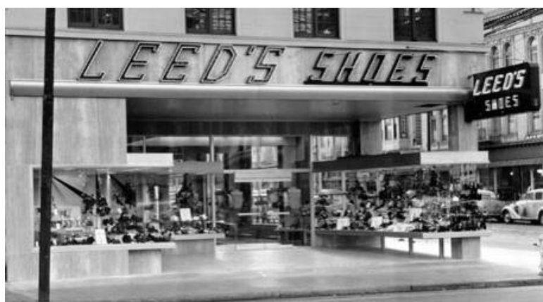
A 1948 remodel of the Mission District Leed's Shoes (above). The “Visual Front” storefront featured floating cantilevered display boxes, a large exterior foyer, cast freestanding letters and plate glass windows. The interior (left) featured “television wall show windows.” The storefront was demolished in the 1990s. (San Francisco History Center, San Francisco Public Library)
