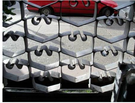
The flagship 1963 Bay View Federal Savings on Mission Street (left) features glass cladding, a barrel-vaulted roofline, a midlevel terrace, and, at the lower stories, metal sheathing. The anodized sheathing (above) mimics the shape of an eagle, the bank's corporate logo. The bank sits on squat structural supports, producing a floating effect at the ground level. It was designed by FTM Associates. Photo: San Francisco History Center, San Francisco Public Library; Mary Brown, San Francisco Planning Department
