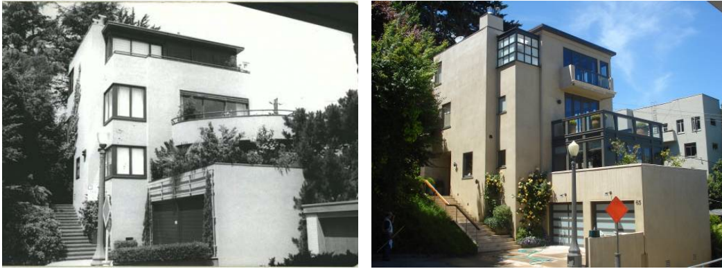
A view of 65 Montclair Terrace in Russian Hill neighborhood in 1976 and today. Unsympathetic alterations to this (1938) Gardner Dailey design, has diminished many of the building's original character-defining features. Photos: 1976 Architectural Survey field form; www.mapjack.com
