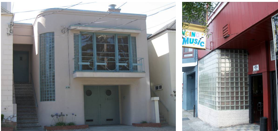
Left: Glass blocks were occasionally used as exterior walls as seen in the curved bi-level wall of this unusually intact tract house at 1547 37 th Avenue, constructed in 1939 by Sunset District tract builder Claude J. Lindsay. Glass blocks were commonly used to flank central windows in residential buildings, which evoked the appearance of shutters. Right: A remodeled storefront at 3247 Mission Street in the Excelsior District. Photos: Mary Brown, San Francisco Planning Department
