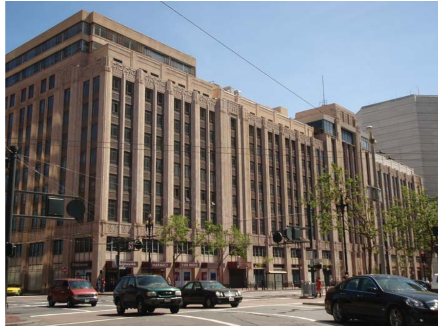
View of Market Street facade from Ninth Street
