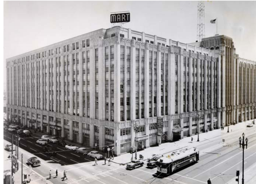
View southwest from corner of Ninth and Market Streets, 1955 [Note completed Ninth Street wing (1947), and wood-frame ninth floor additions (1941)] (SFPL, #AAC-5016)
