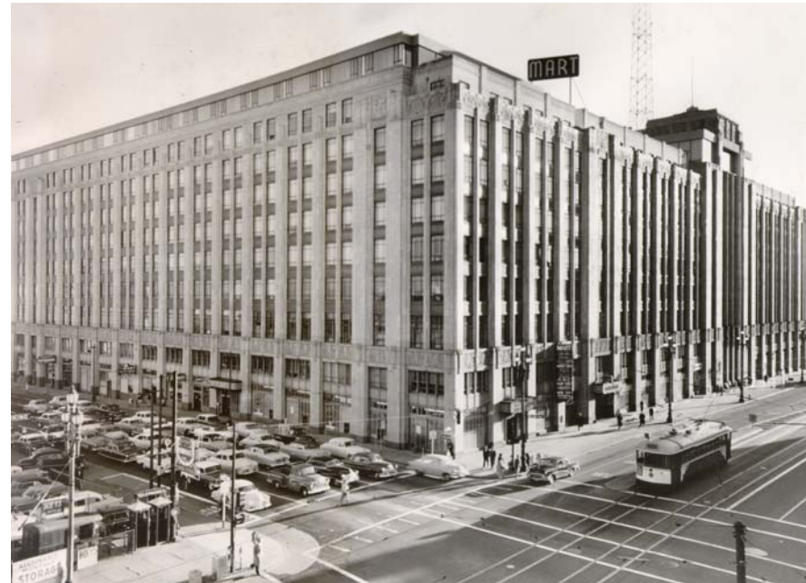
View southwest from corner of Ninth and Market Streets, 1961 [Note tenth floor addition and tower alterations (1958)] (SFPL, #AAC-5012)
