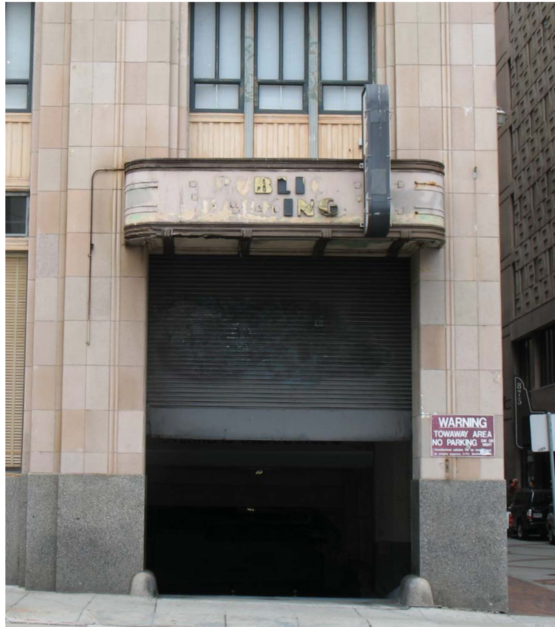
Existing entry to the garage at Tenth and Stevenson streets
