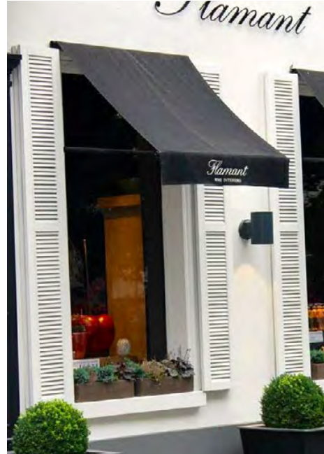
This awning fits well within existing opening.
