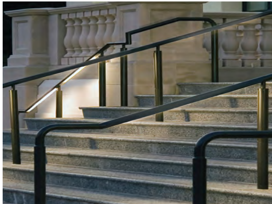
Example of an appropriate illuminated handrail
