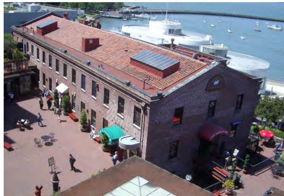
Woolen Mill: Aerial view, looking northwest
