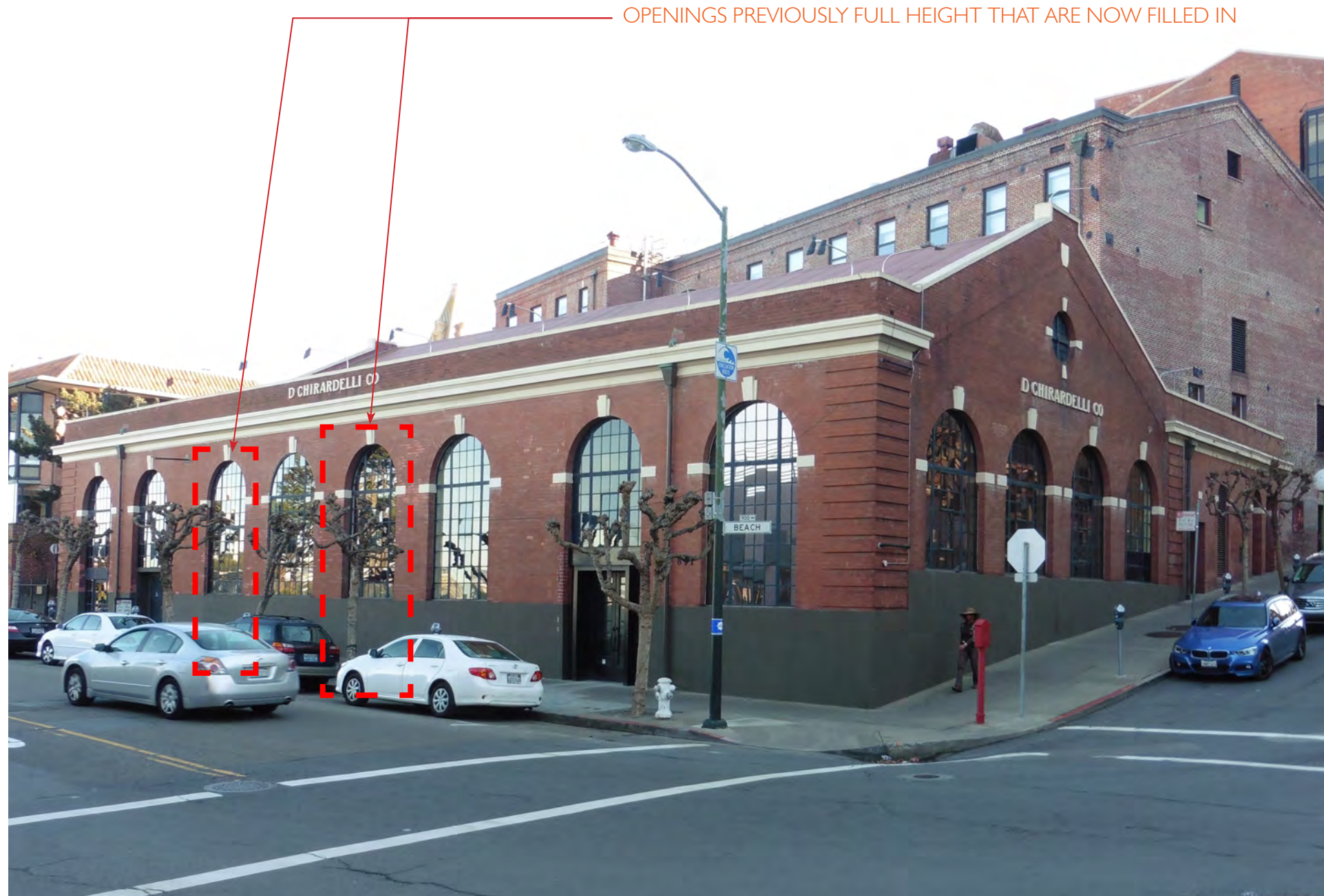
Power House - view from Larking and Beach streets. Note: there are currently three full height openings along Beach Street
