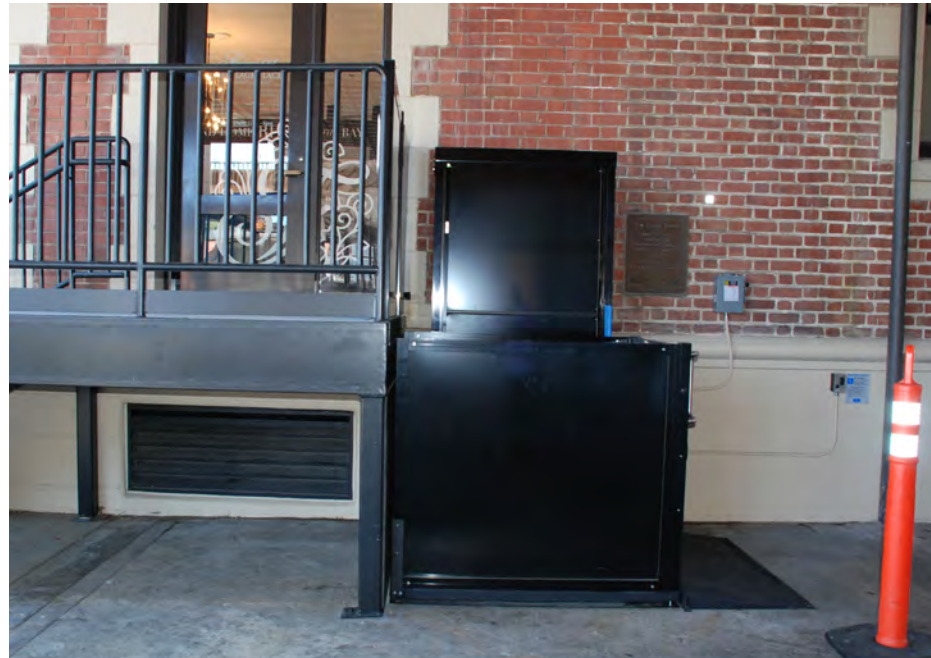
The wheelchair lift at Clock Tower is located in an unobtrusive location. The metal is painted black, compatible with the adjacent landing and guardrail.
