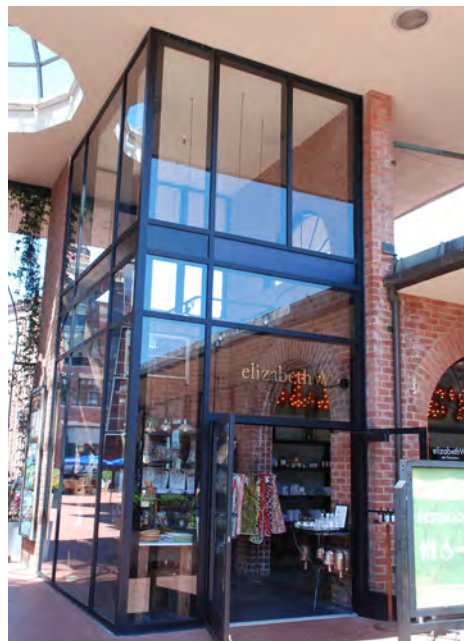
Appropriate storefront replacement at the Gateway Shops
