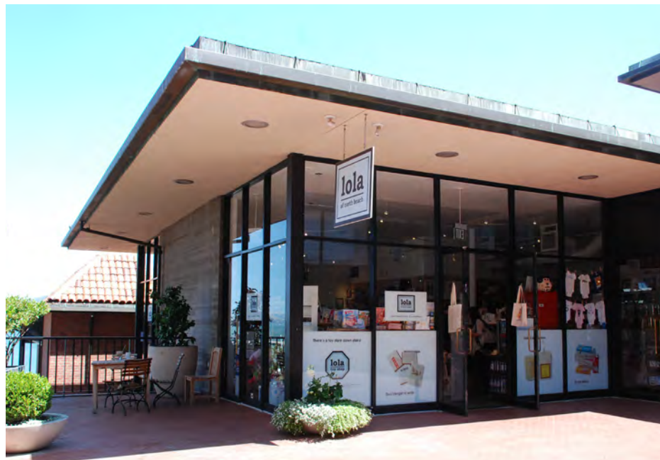
The sign hanging from this 1960s pavilion uses compatible materials and has an appropriate scale.
