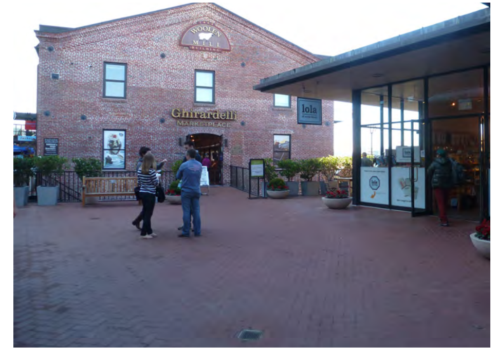
West Plaza, view looking west
