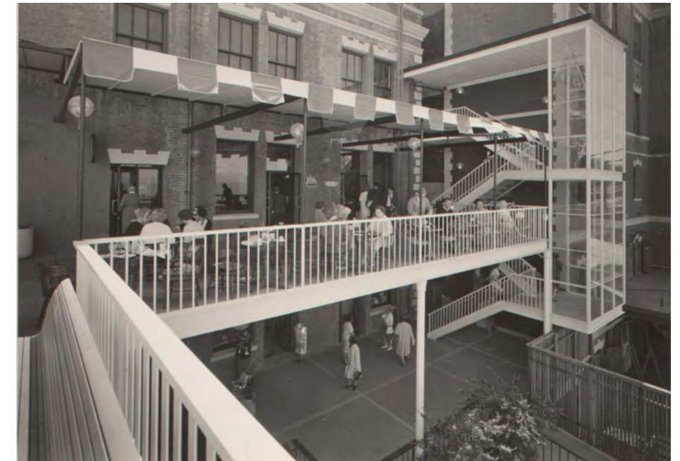
Glass Stair Enclosure at the Cocoa and Chocolate Buildings
