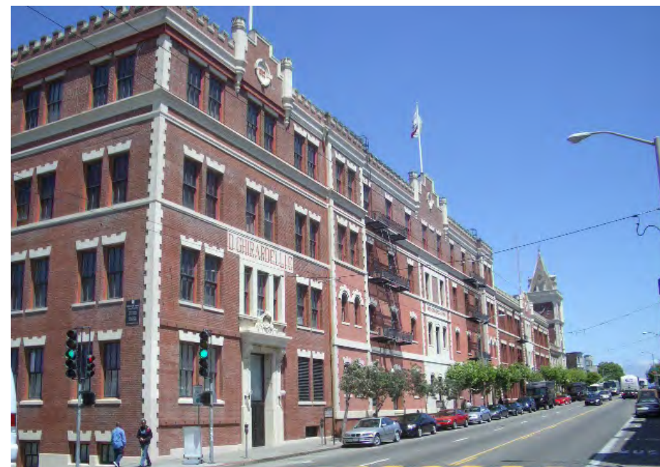
The Chocolate (in foreground), Cocoa, and Mustard Buildings retain original signage from the date of construction.
