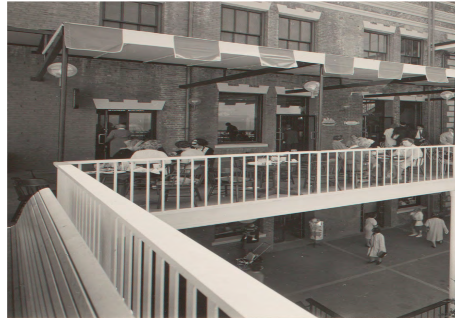
Canopy at the upper level of the north facade of the Chocolate Building, 1960s.
