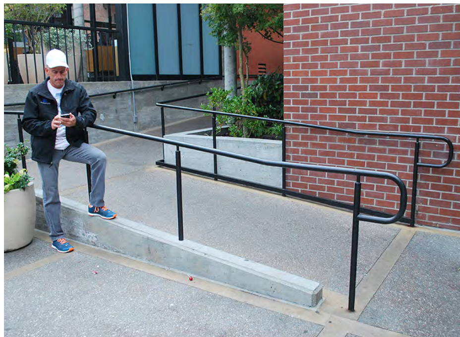
Appropriate - a slope within the Square's interior meets ADA standards using suitable materials.
