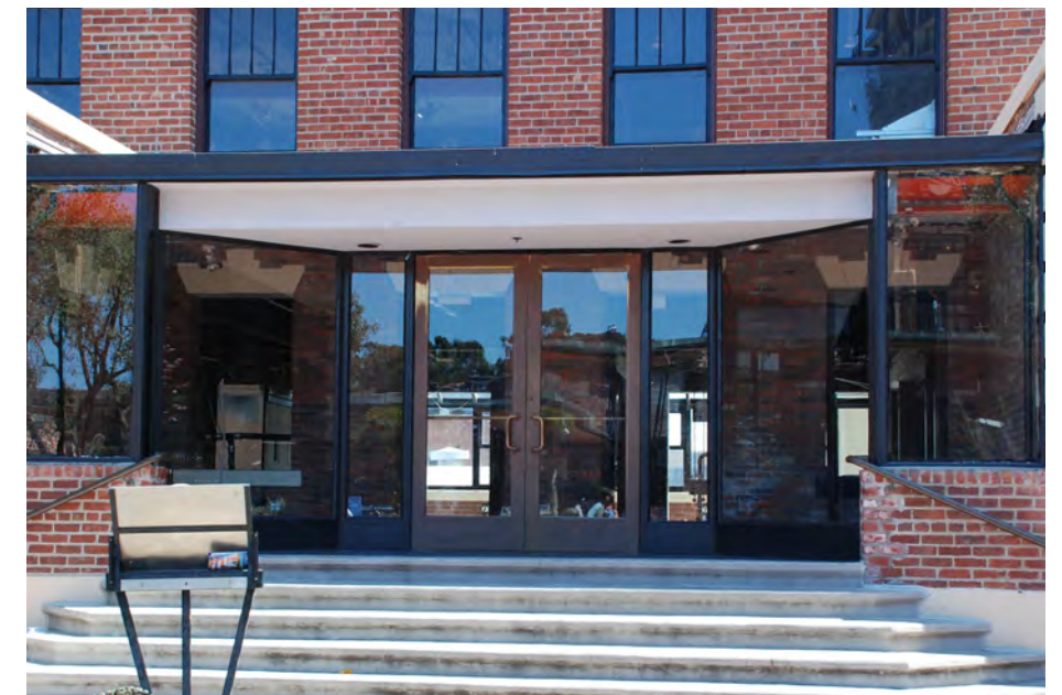
These entrance doors do not match the character of the rest of the storefront. They are lighter in tone and have wider stiles and rails compared to the storefront.
