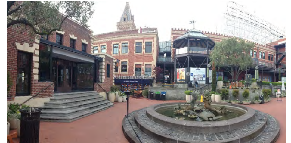
Existing conditions at Apartment House and Mermaid Fountain
