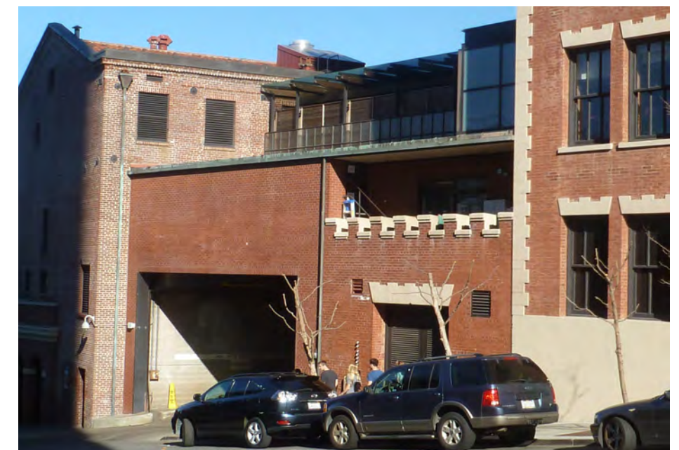
View of Polk Street facade, looking northeast
