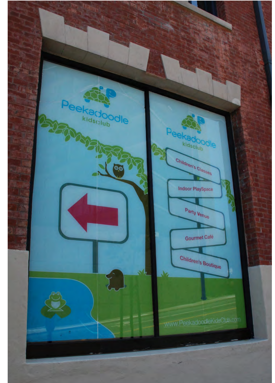
Inappropriate Replacement: Though part of the 1960s work, the replacement of a pair of original windows with a single window is not appropriate.
