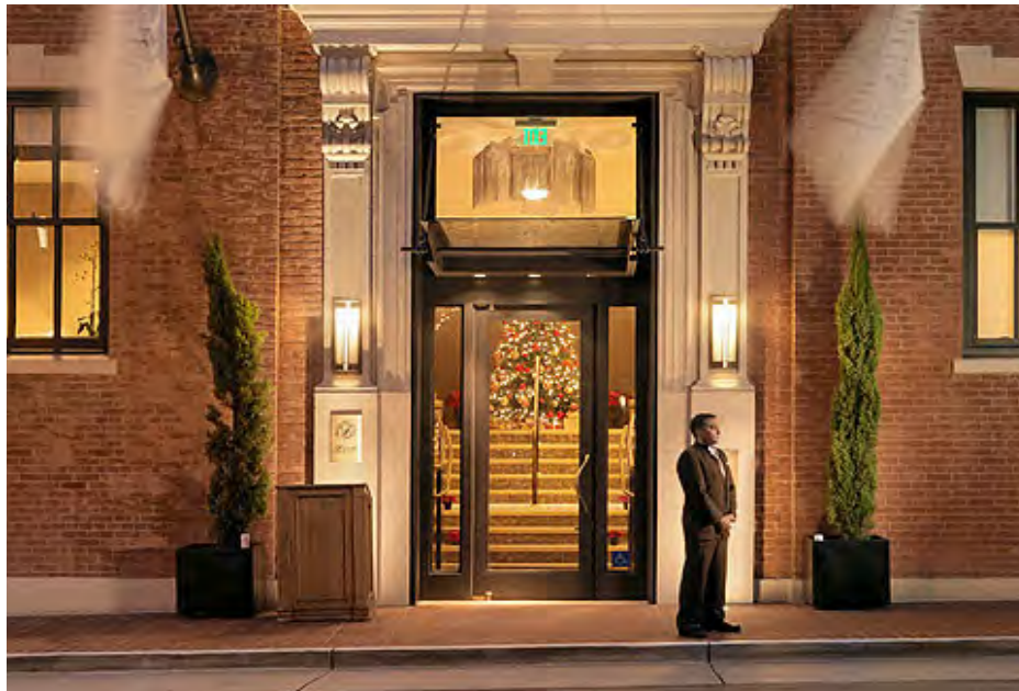
The contemporary entry door at the Chocolate Building entrance is well proportioned and uses materials compatible with the building.
