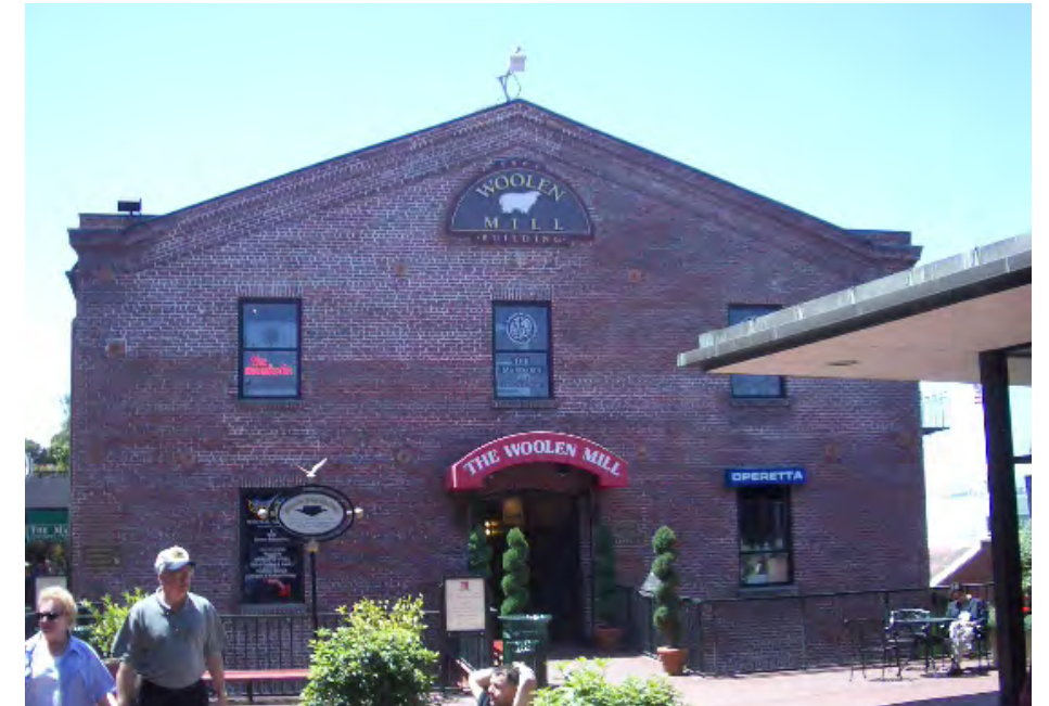
Woolen Mill: East facade
