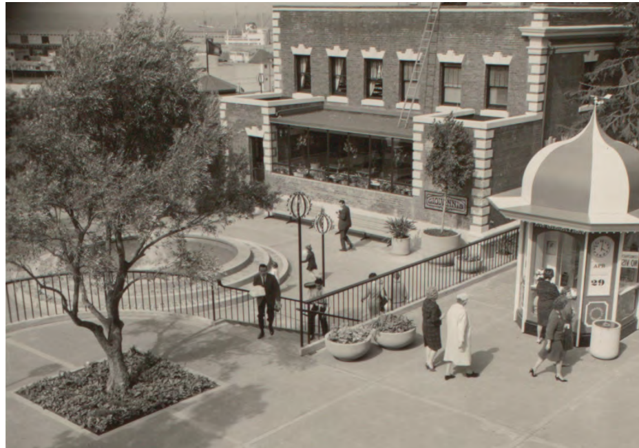
Apartment Building: Note that the steps at the existing west facade were not part of the 1960s rehabilitation (Environmental Design Archives, 1960s).
