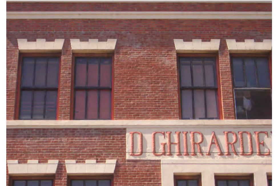
Several of the original Ghirardelli Buildings have double-hung steel windows.
