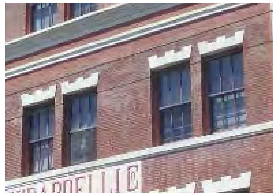
Chocolate Building: Original steel double-hung windows
