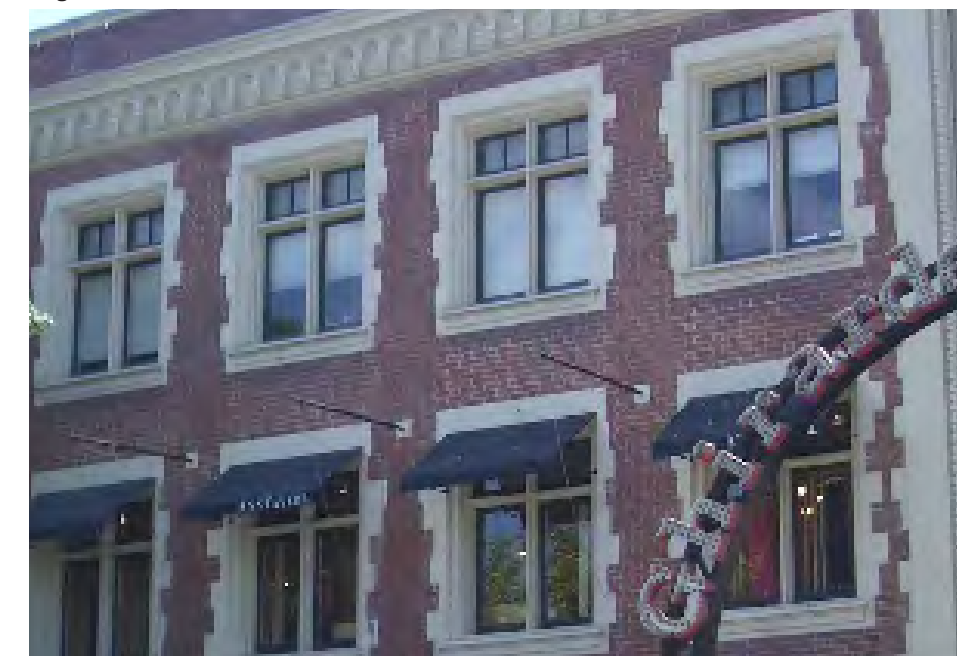
Clock Tower: Original steel casement windows.
