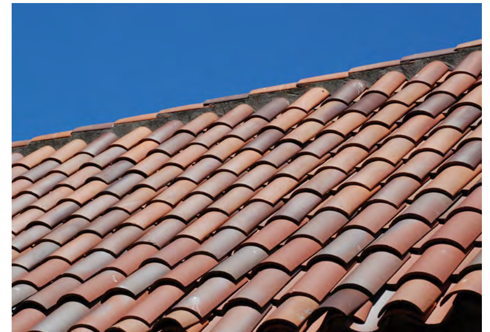
The clay tile roof of the Wurster Building is a prominent feature of the Square and an appropriate exterior material .
