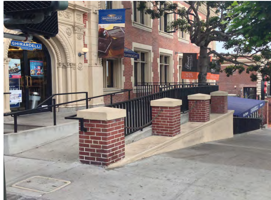
Appropriate - an exterior slope meets ADA standards using suitable materials.
