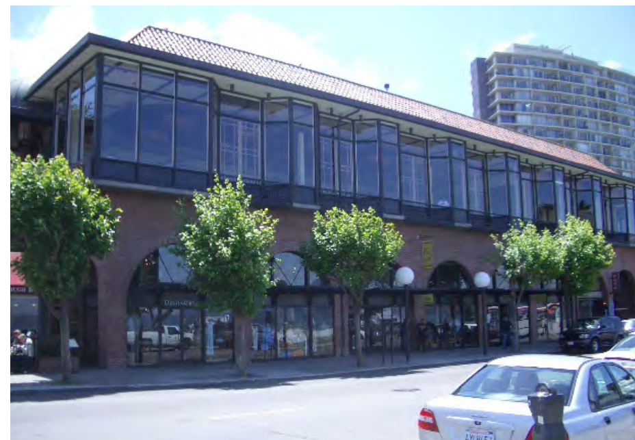
Wurster Building: North facade, view looking southwest
