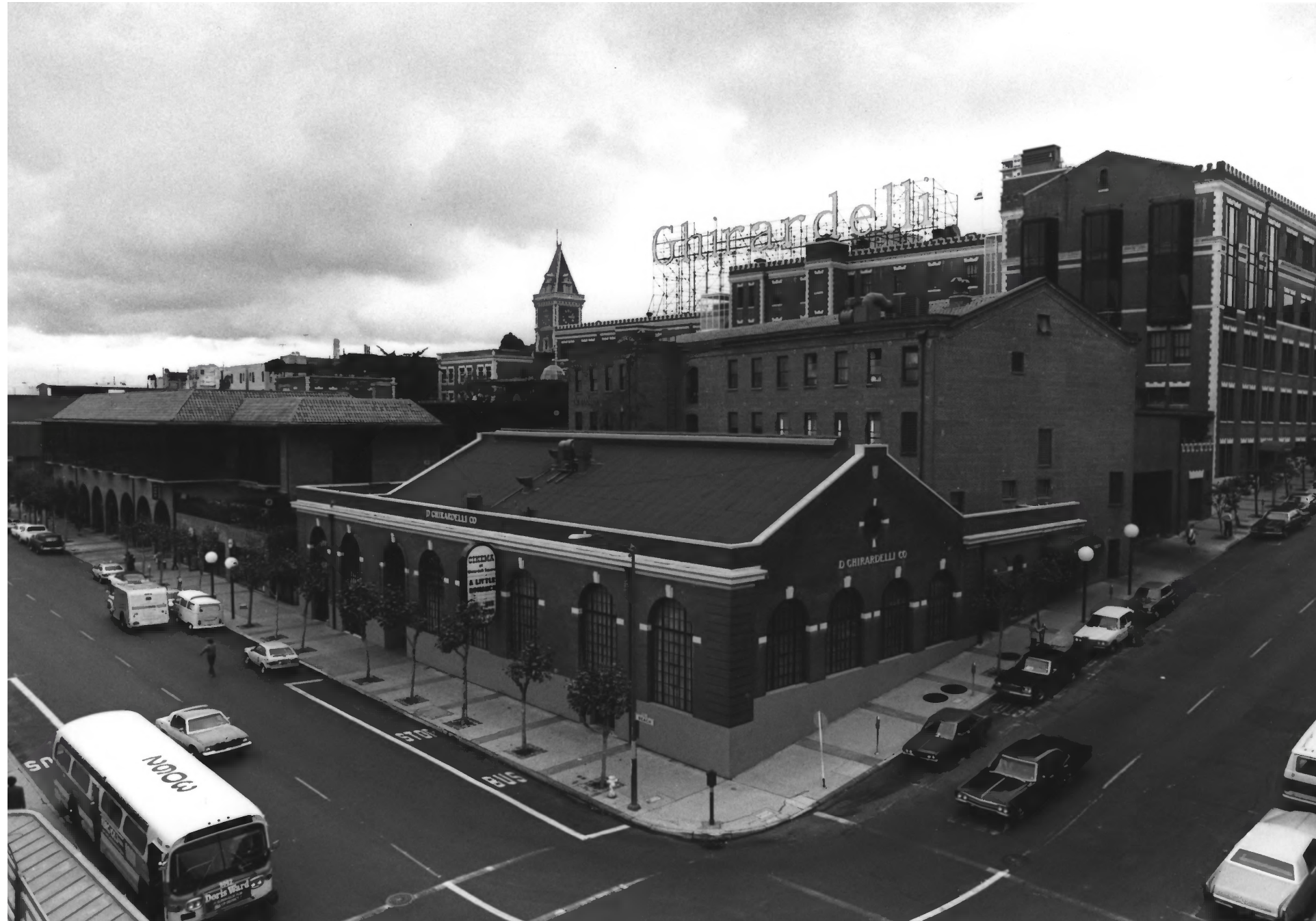
View of Ghirardelli Square with Power House at the forefront: ca 1975, Photograph by John Griffith. National Register Nomination
