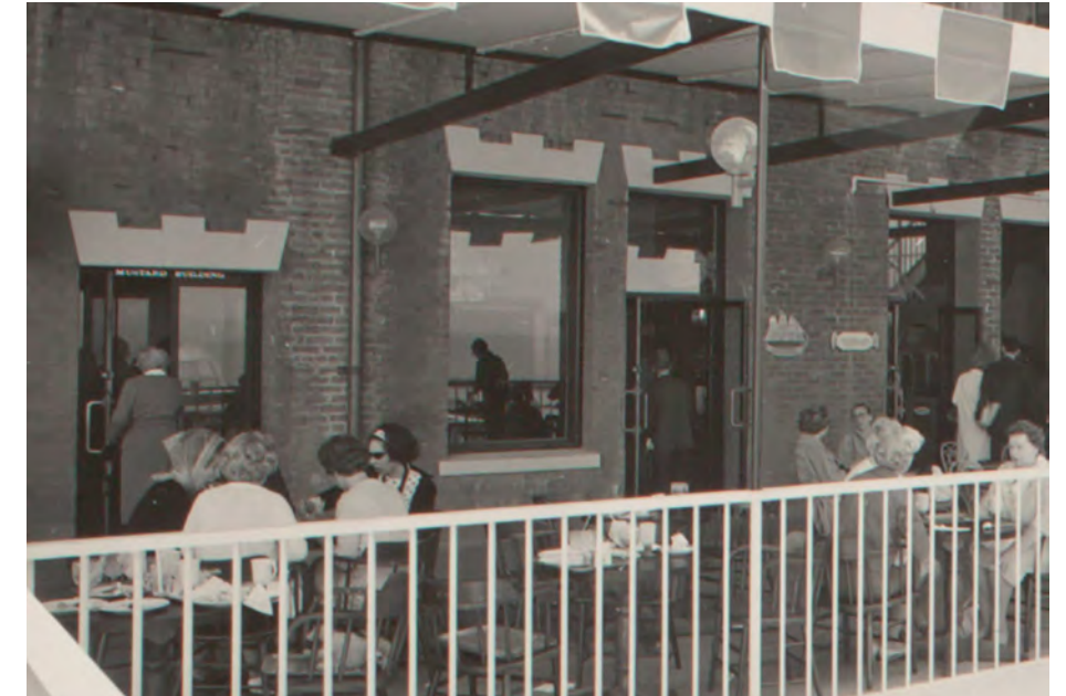
Mustard Building: Entry door was replaced on the north facade with a storefront door (Environmental Design Archives)
