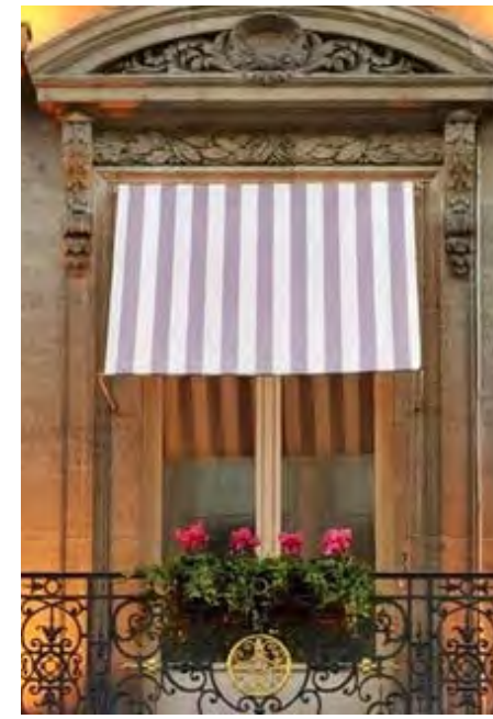
The pattern of this awning does not overpower the architectural features.
