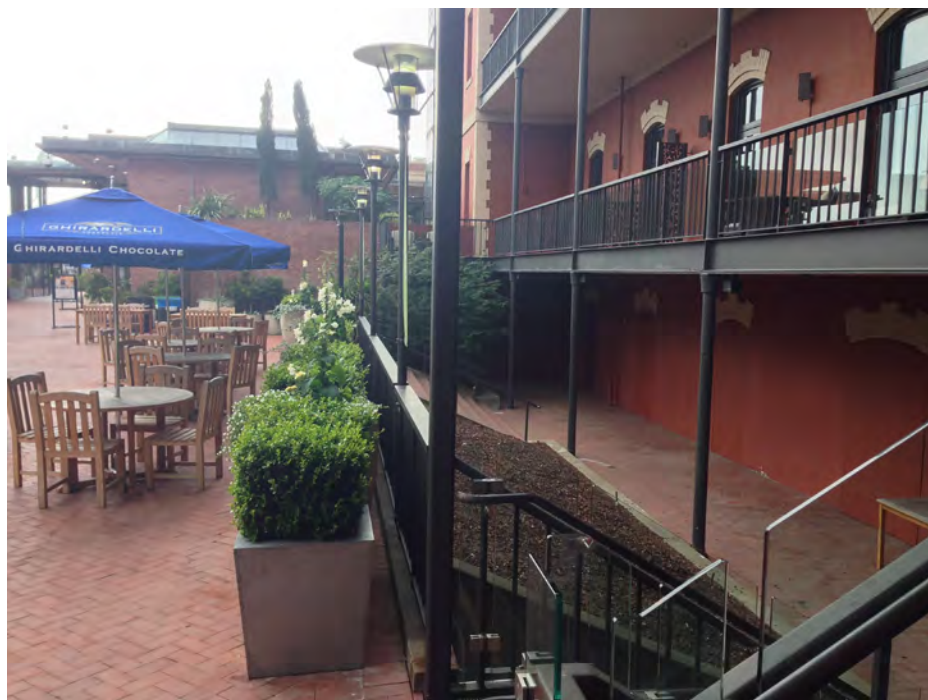
Photo 6 - Existing empty planter at Cocoa Bldg. basement
