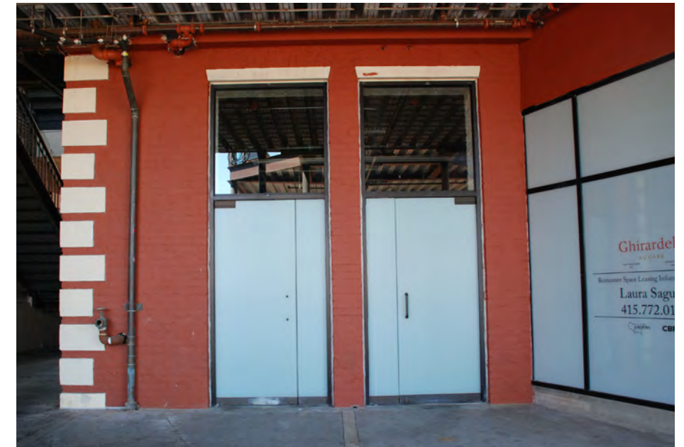
Frameless doors at the Mustard Building.
