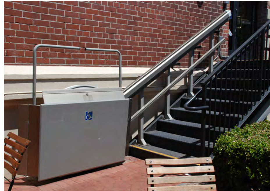
This wheelchair lift at Apartment House is located on a secondary facade. A darker tone of grey would make the lift less obtrusive.
