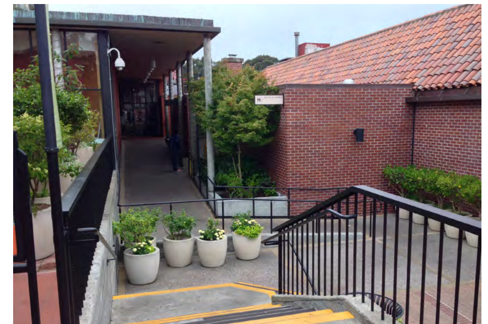
Promenade Level: Existing condition photo, view looking west
