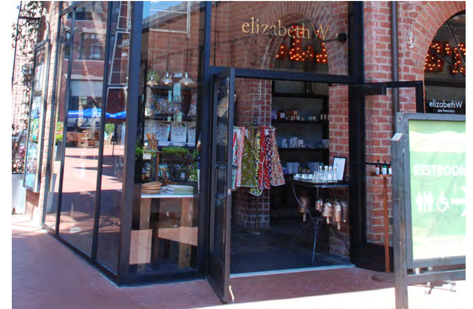
Gateway Shop: Entrance doors have fairly narrow stiles and rails. Their dark color is consistent with the storefront color.
