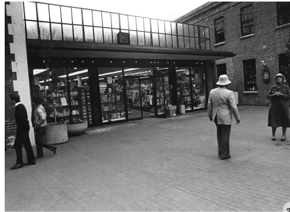
View of Coagulation Building with West Plaza in the foreground. (Allen Nomura, 1982)
