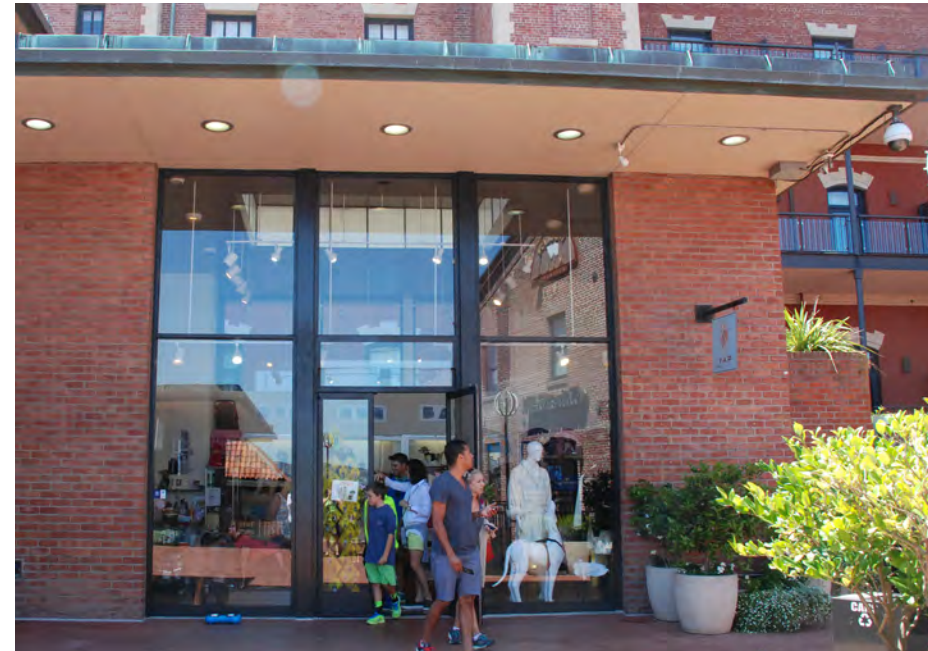
Building materials used in the 1960s additions include sand mold brick, metal, and cement plaster storefronts. These continue to be appropriate materials today..
