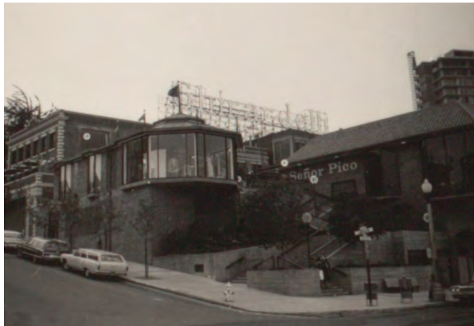
Apartment Building: Note that the existing green house on the east elevation had not yet been constructed (Environmental Design Archives, 1960s).
