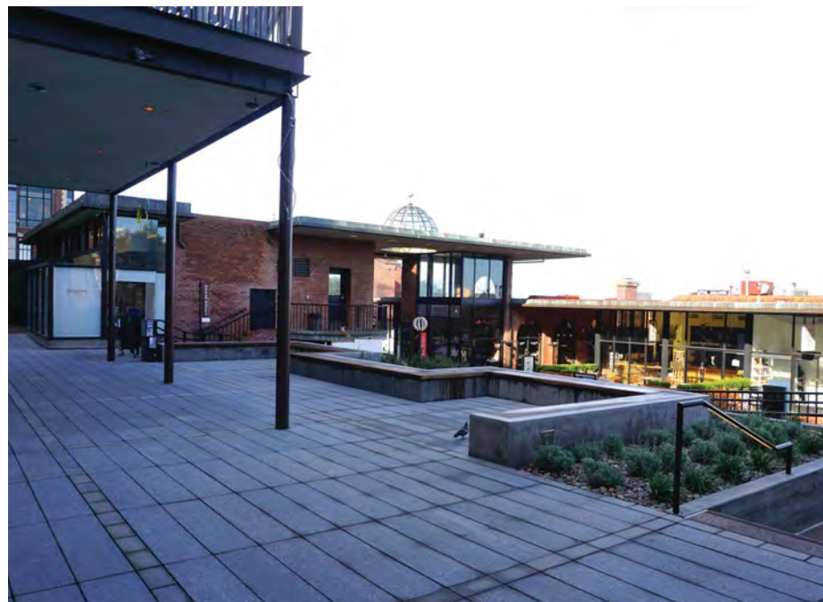
View of renovated Upper Terrace, looking northwest
