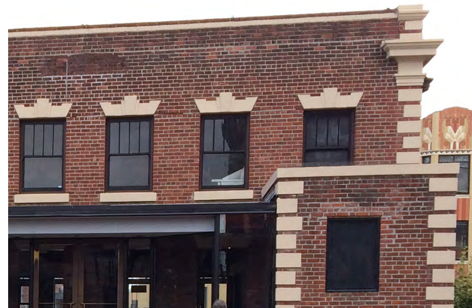
Apartment Building has wood windows.
