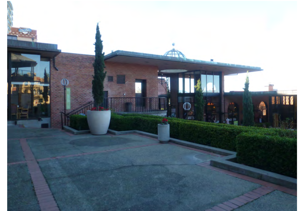
West Plaza, view looking west, 2015
