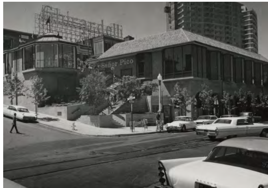
Carousel Building and Wurster Building both have glazed storefront walls that face the Bay
