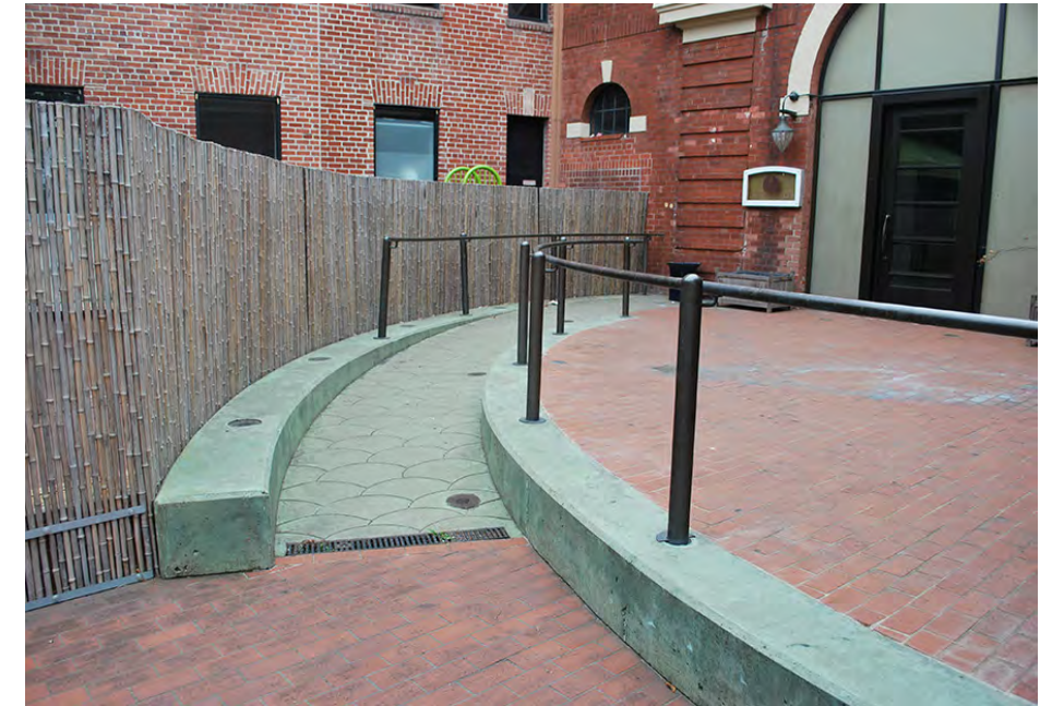
Inappropriate - paving materials and style should be in keeping with the character of Ghirardelli Square.
