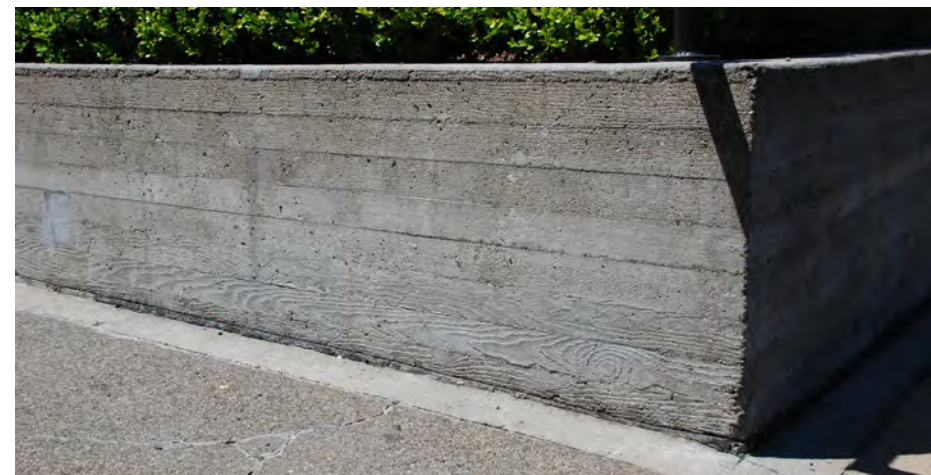
Appropriate existing paving and walls at Ghirardelli Square includes seeded concrete and board formed concrete.
