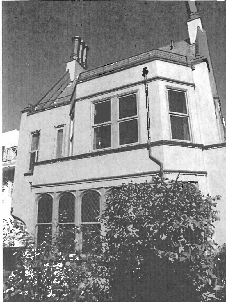
South elevation. Carey &amp; Co., Inc.
