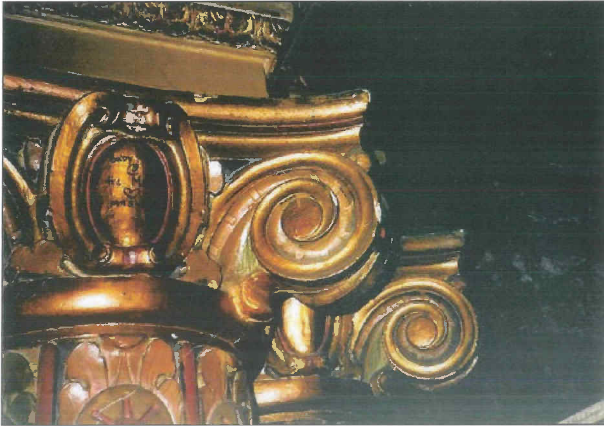
Detail view of capital in auditorium prior to 1998 renovation. (Source: Gary Parks, 1998, http://www.flickr.com/photos/howardbhaas/285871917/ ).
