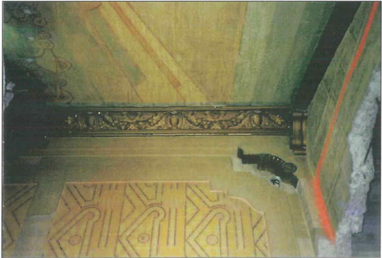
Detail of finishes at ceiling and wall of lobby prior to 1998 renovation. (Source: Gary Parks, 1998, http://www.flickr.com/photos/howardbhaas/285871917/ ).
