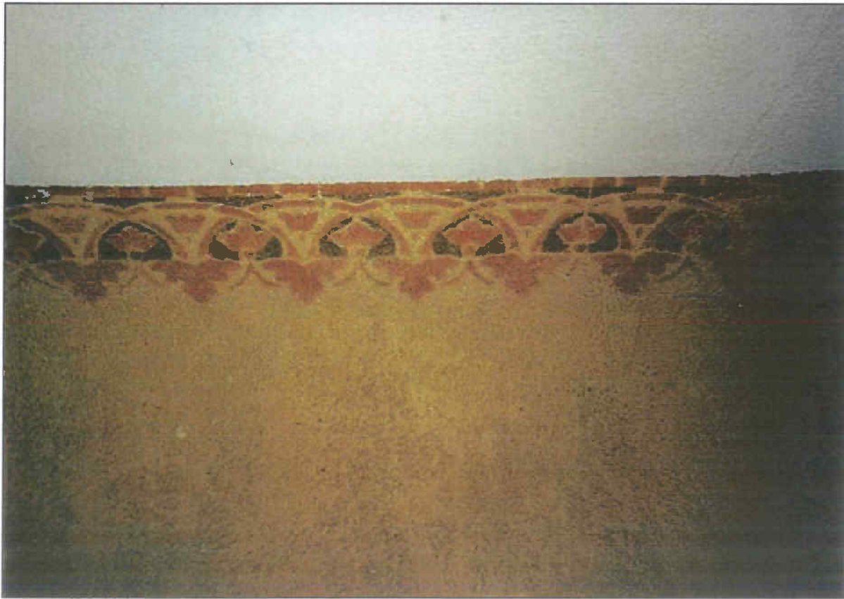
Detail view of finishes at ceiling of mezzanine prior to 1998 renovation. (Source: Gary Parks, 1998, http://www.flickr.com/photos/howardbhaas/285871917/ ).
