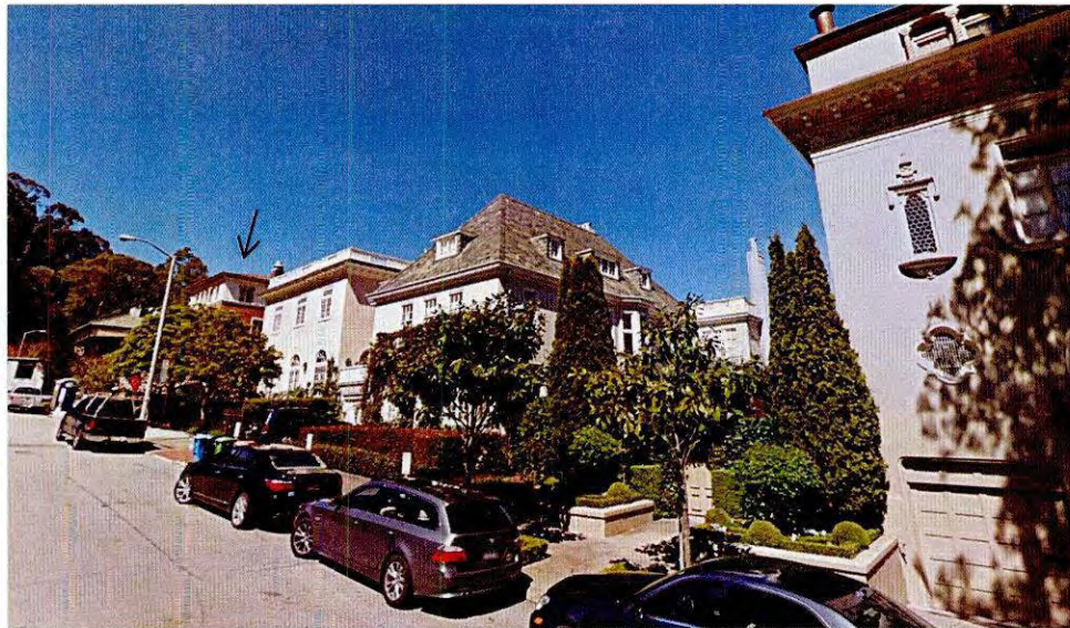
Contextual view of 2950 Vallejo Street relative to the adjacent block face (Google Maps)
