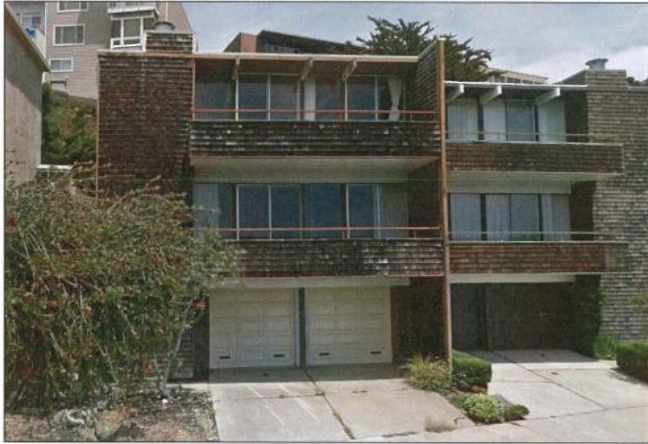
261 Amber Drive, view N of primary façade (south elevation), prior to unpermitted exterior alterations that took place between July 2015 and June 2016, (Google street view)
