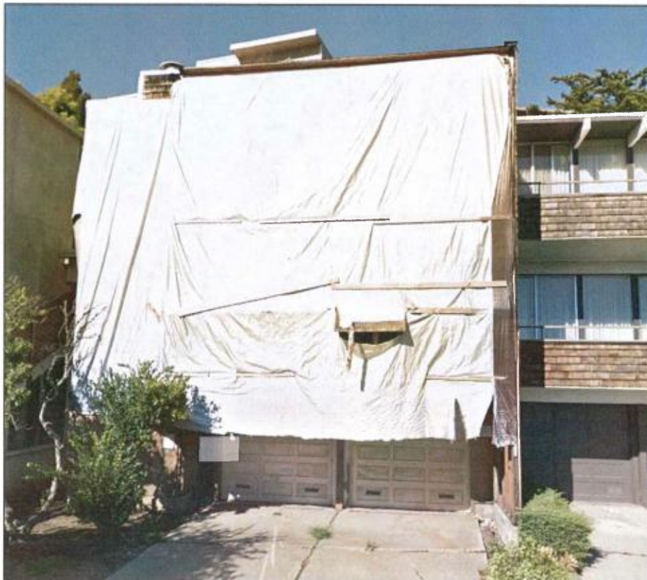
261 Amber Drive, view N of primary façade (south elevation), at is appears today, (Google maps)
