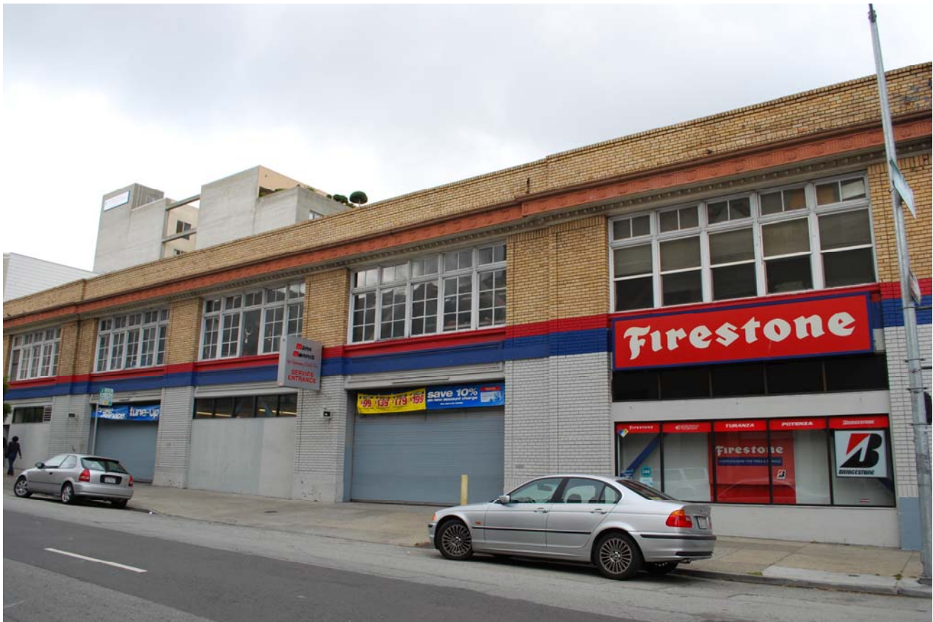
View looking NE at the Larkin Street side of the building
