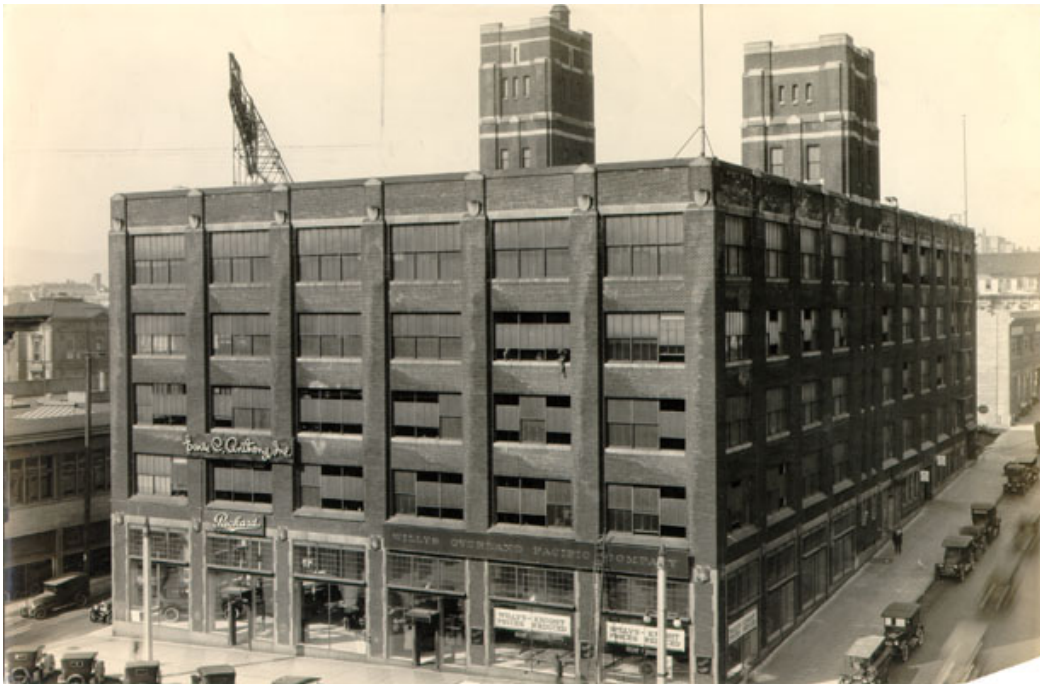
Photo from 1921-1923. Earle C. Anthony's Packard showroom occupies the bays to the south, and Willys Overland's showroom is in the bays to the right. San Francisco History Center, Main Library. Photo AAD-4662.
