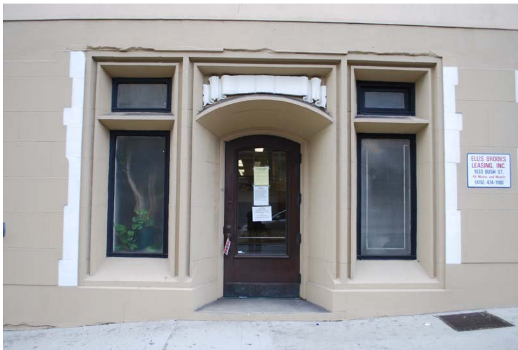
Top photo: Main entrance, Van Ness Avenue. Bottom photo: Entrance on Bush Street. Their decorative treatments indicate they may date to the original construction of 1916.
