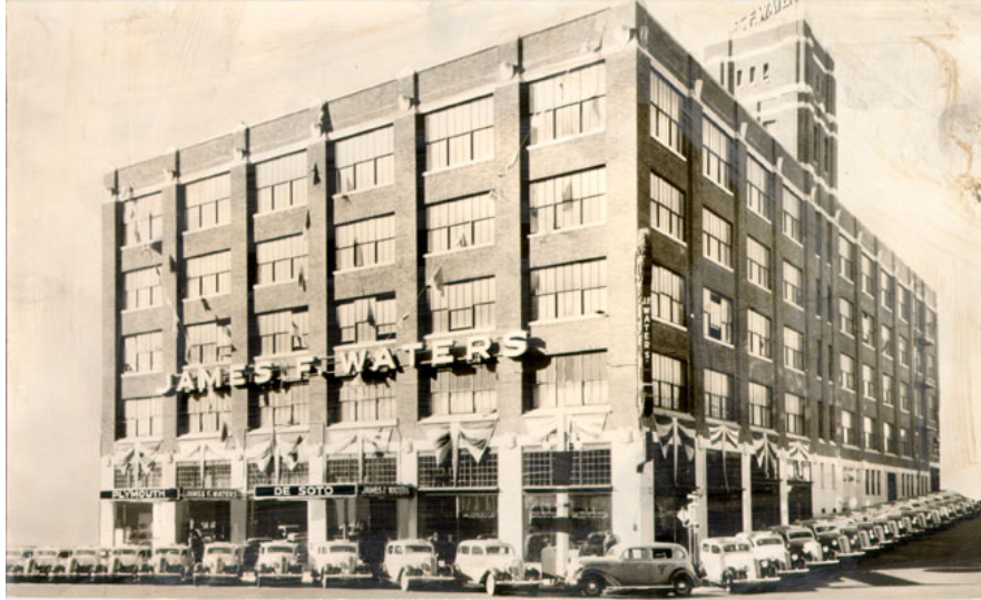
Photo dated November 1935, the same year James F. Waters occupied this building. The autos parked in front are DeSotos, destined to become part of Yellow Cab's fleet of 300 autos. San Francisco History Center, Main Library. Photo AAD-4674.
