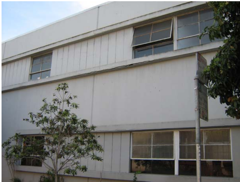
Detail of windows on primary façade
