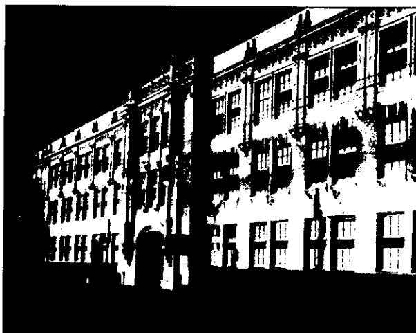
Image 38, above: High School of Commerce, built 1926, located at 135 Van Ness Avenue, date not known. Source: San Francisco History Center, San Francisco Public Library.
