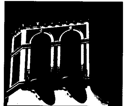
Image 18, upper right: The cupola tower, Aug. 2006. View west.
