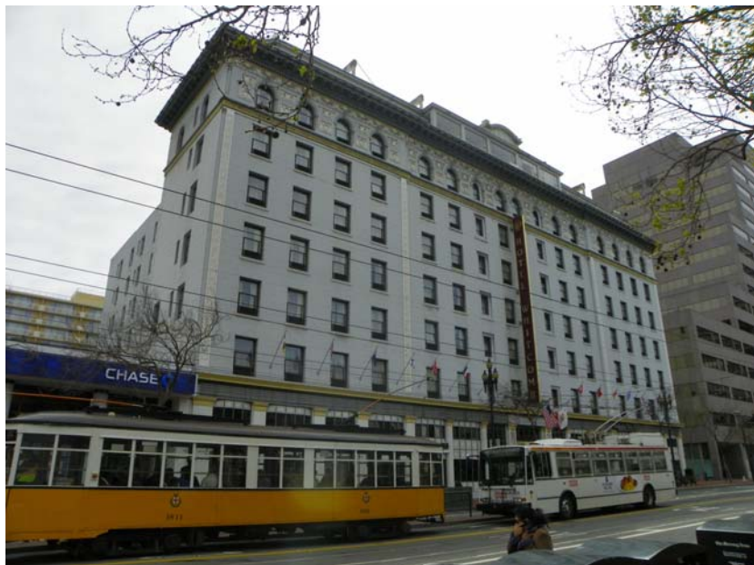
View of northwest facade. 103_3963.JPG 3/7/2011
