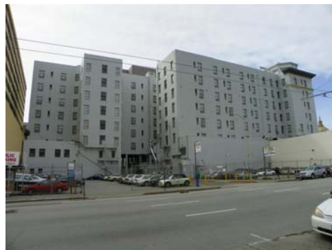
View of northeast facade. 103_3960.JPG 3/7/2011
