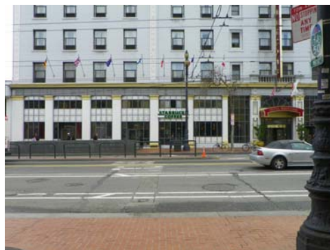
Detail of first story storefronts. 3/7/2011. 103_3965.JPG
