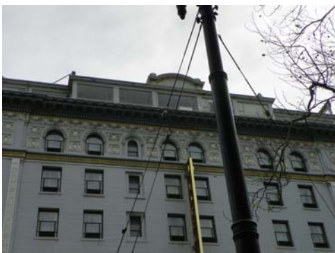
Detail of upper primary facade. 3/7/2011. 103_3964.JPG
