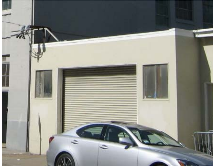
East section of primary façade. Source: Page and Turnbull
