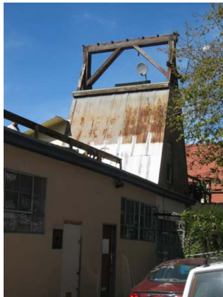
View of secondary façade and mechanical enclosure. Source: Page and Turnbull
