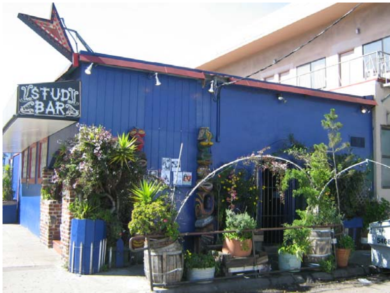
View of rear (east) façade. Source: Page and Turnbull
