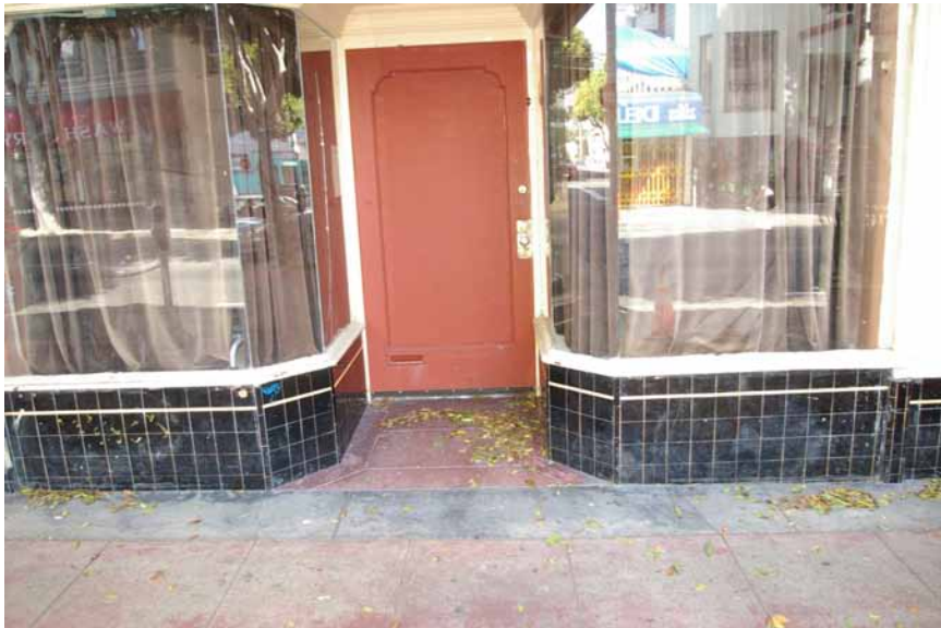
View looking south at an original storefront. Source: San Francisco Planning Department
