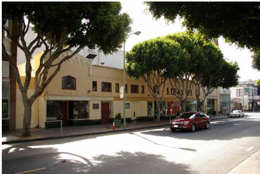
View looking southwest at the primary façade. Source: San Francisco Planning Department
