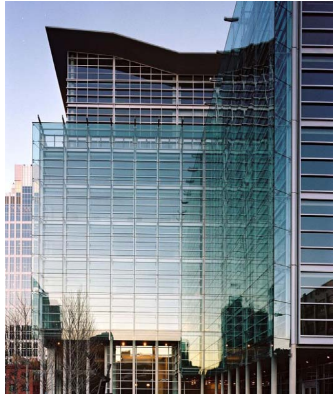
TOP: SoMa's Foundry Square presents a full façade of highly reflective glass. While all glass can be reflective, glass manufacturers label glass with standards "reflectivity" ratings.
