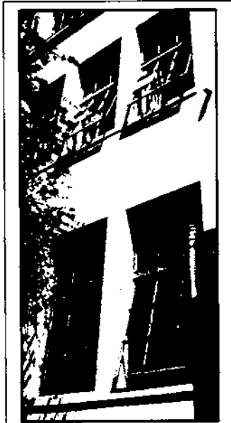
Stacked awning windows in academic classrooms. Source: SF Planning Department.
