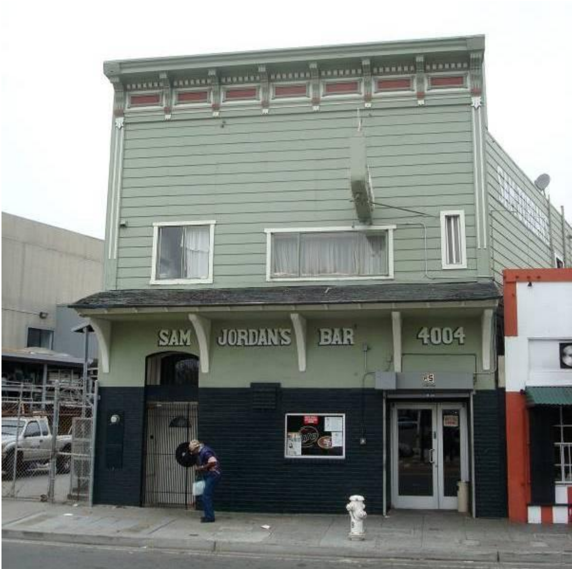
4004-4006 Third Street, Sam Jordan's Bar, primary facade.
