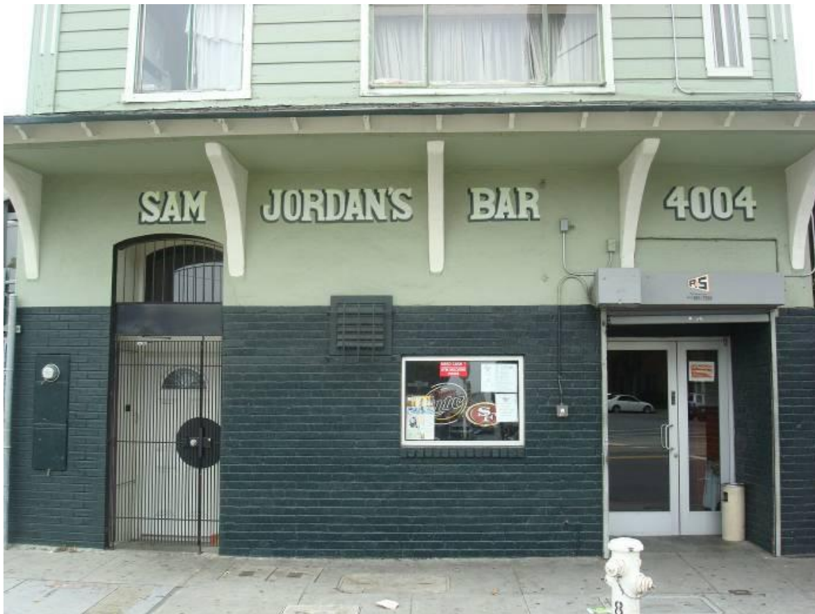
First story, primary facade.
