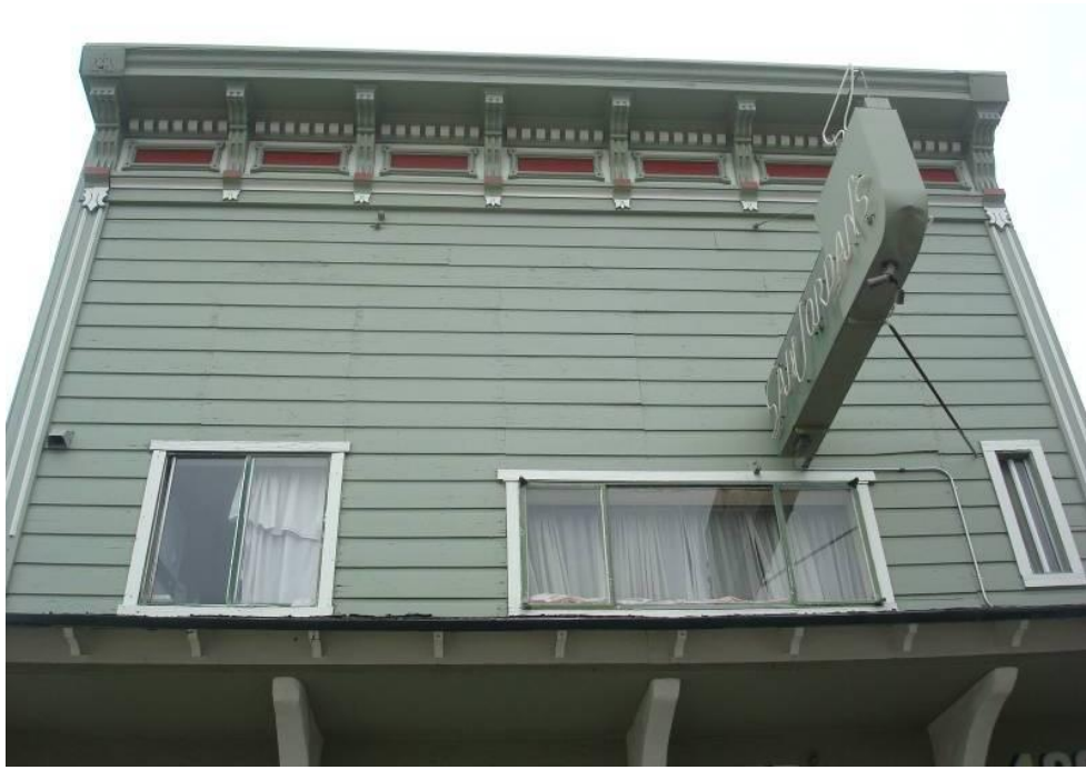
Second story, primary facade.
