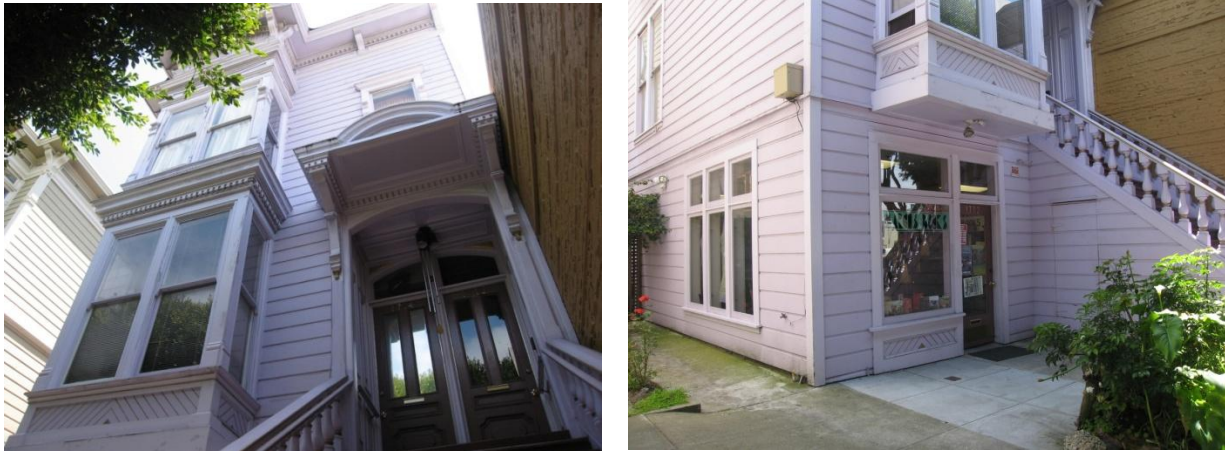
Figure 2: Left: View looking east at upper stories of the primary façade. Right: View looking southeast at storefront space.
