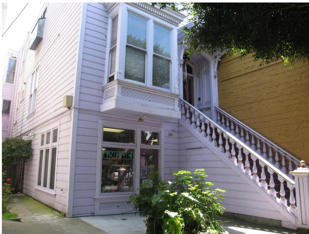
Figure 1: 1712-1716 Fillmore Street, view looking southeast
