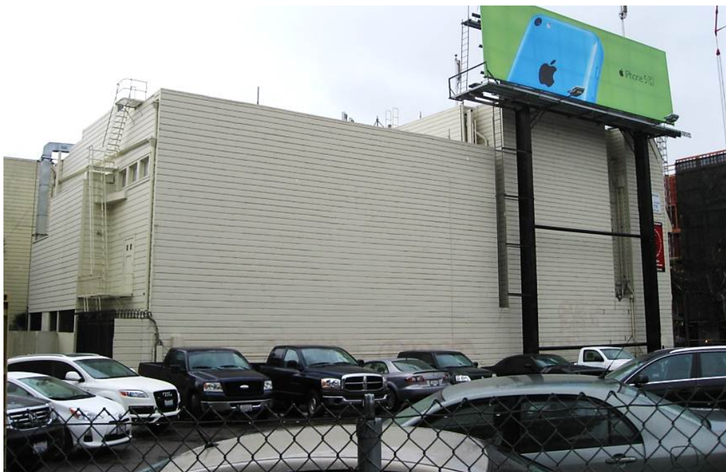
View of the west and rear (north) facades
