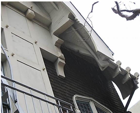
Detail of trim work on the upper facade
