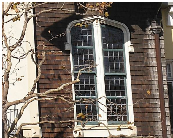
Detail of arched window
