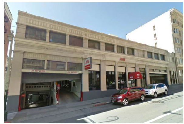
Cristobal Apartments at 750 O'Farrell Street (1913) at top; Parking garage at 675 Post Street (1919) at bottom.
