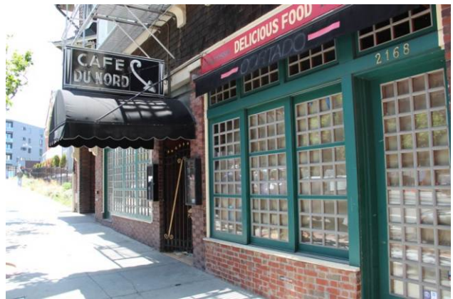
View of the storefronts. Note the non-historic brick cladding beneath the storefront window at right
