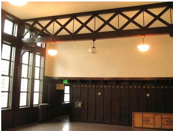
Second floor lodge room, view to west wall
