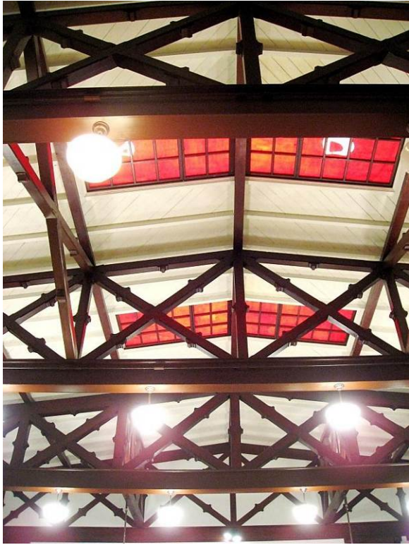
Detail of skylights
