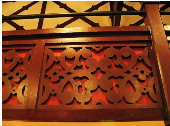
Detail of balcony fretwork
