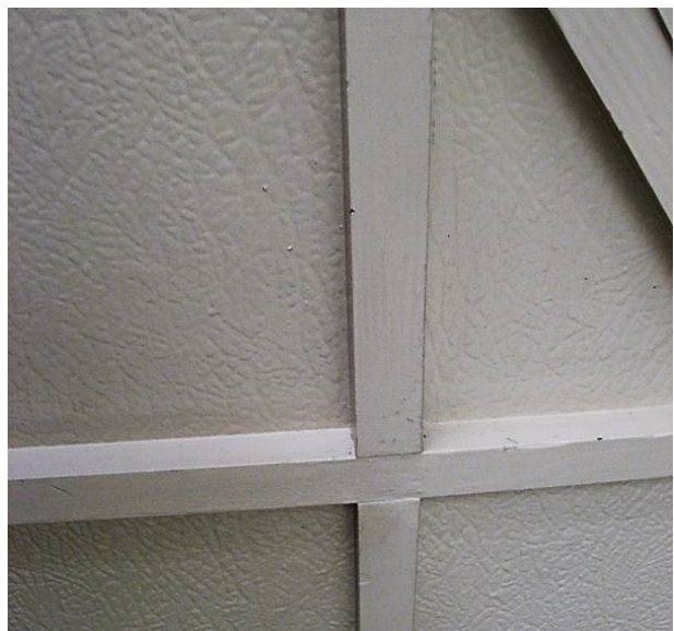
Detail of the leather paper wall cladding
