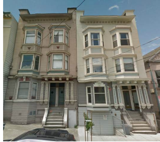
Flats at 847-851 and 853-857 Cole Street designed by August Nordin and completed ca. 1904. 23 (Google Maps)
