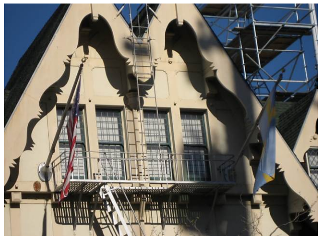
Detail of the barge boards and shadow lines
