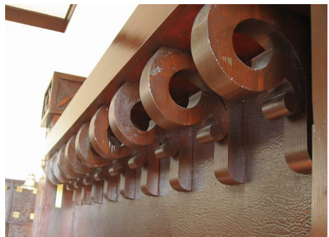
Detail of scrolled brackets beneath the east wall mantle
