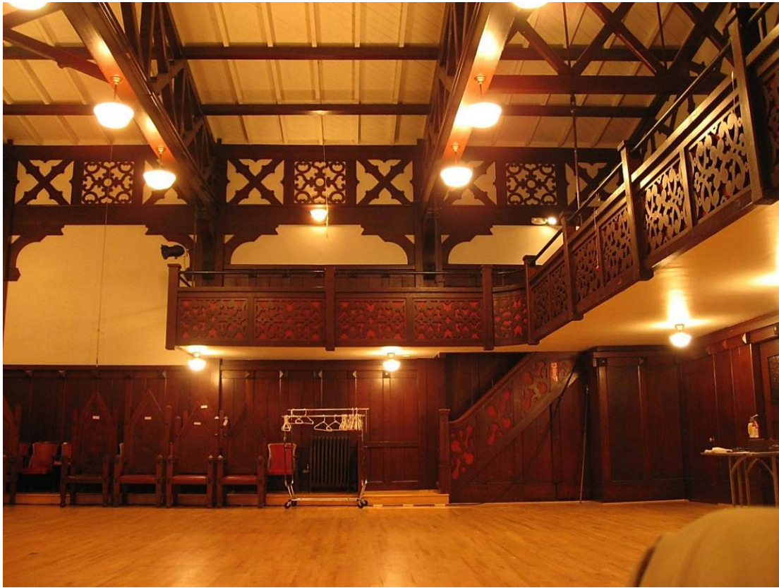
View east across Freja Hall showing trusses and trim work. Note the staircase leading to the balcony level at lower right.
