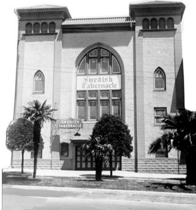
1930 view of the Swedish Tabernacle at 455 Dolores Street, constructed in 1908. (San Francisco Public Library Historical Photo Collection)
