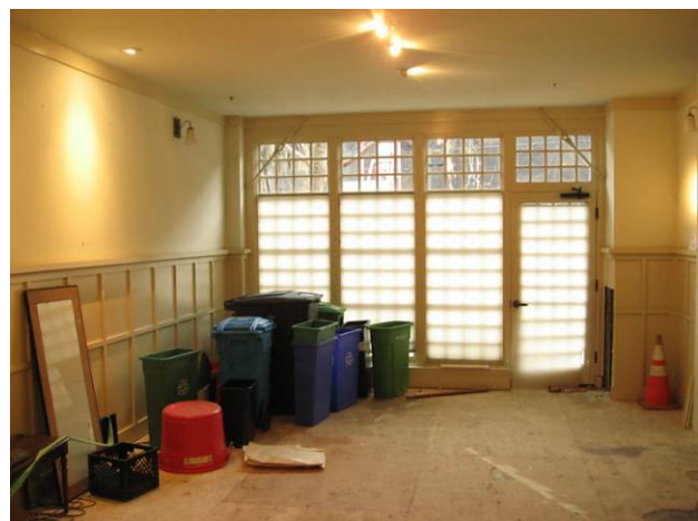
View north of the reception area, formerly used as a store at 2172 Market Street.
