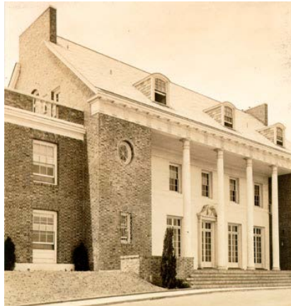
University Mound Old Ladies' Home shortly after construction (San Francisco Public Library, June 16, 1932)
