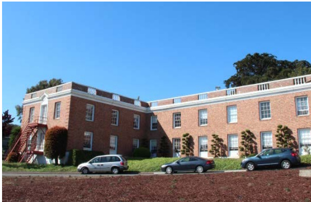
Primary (east) façade of south wing, April 2015
