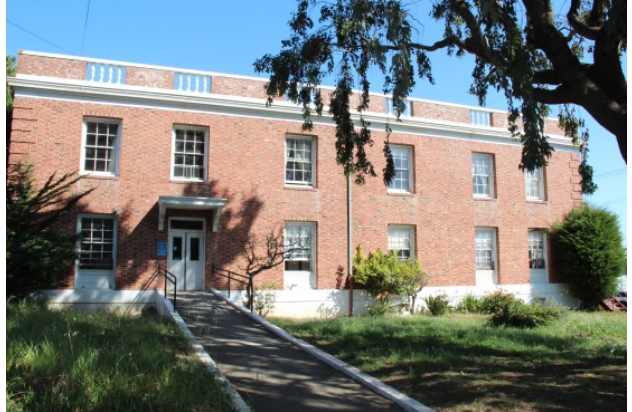
South elevation of south wing, April 2015
