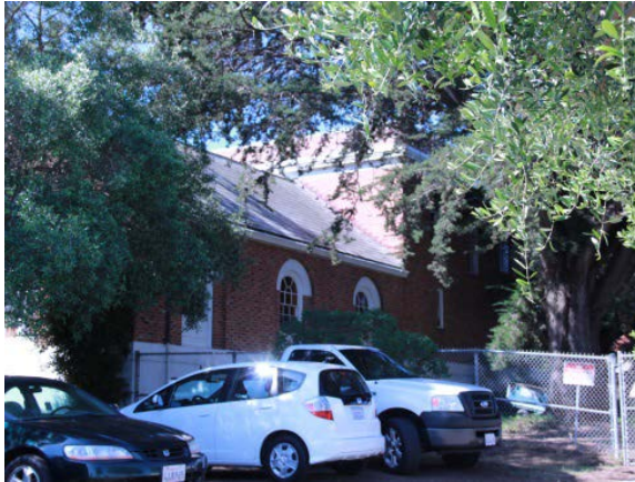
North elevation of chapel, April 2015
