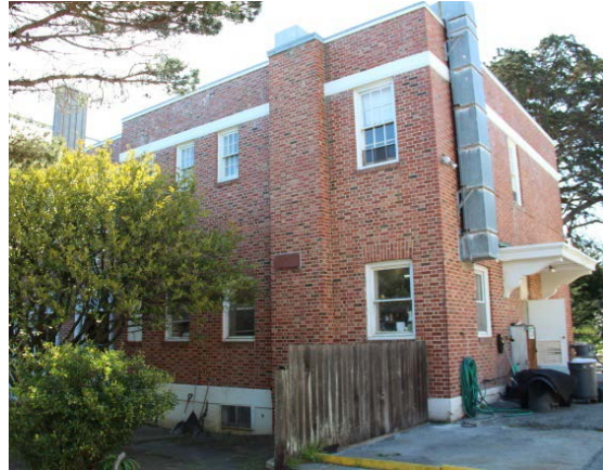
North elevation of service wing, April 2015
