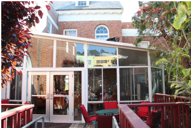
Sunroom alteration at west elevation of south wing, April 2015
