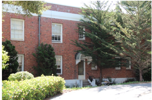
West elevation of south wing, April 2015
