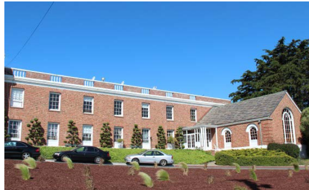
Primary (east) façade of north wing, April 2015
