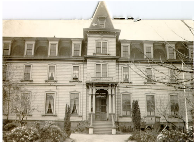
Original building of the University Mound Old Ladies' Home (San Francisco Public Library, March 6, 1930)
