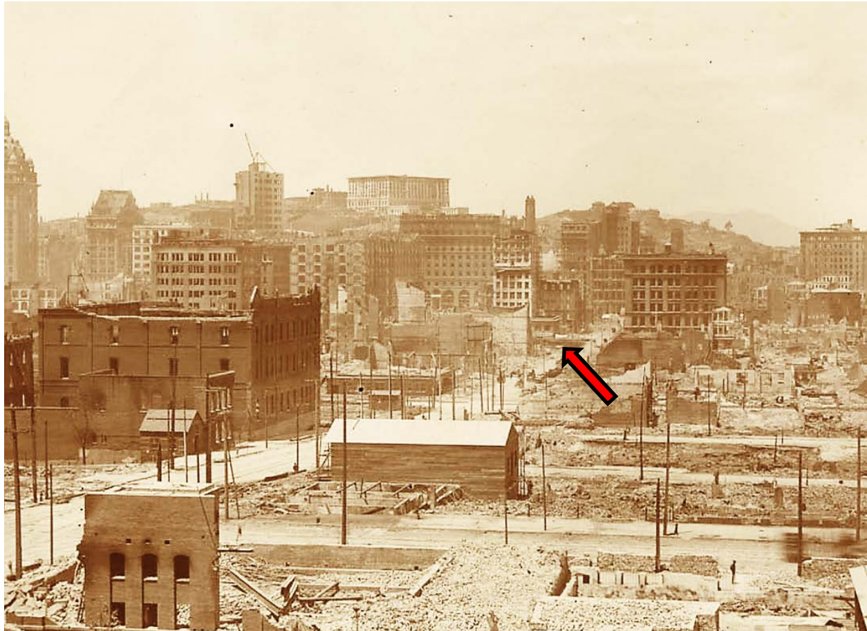
View north from Folsom Street near Second Street, circa May 1906. Arrow added by author to show the Bourdette Building. (California Historical Society)
