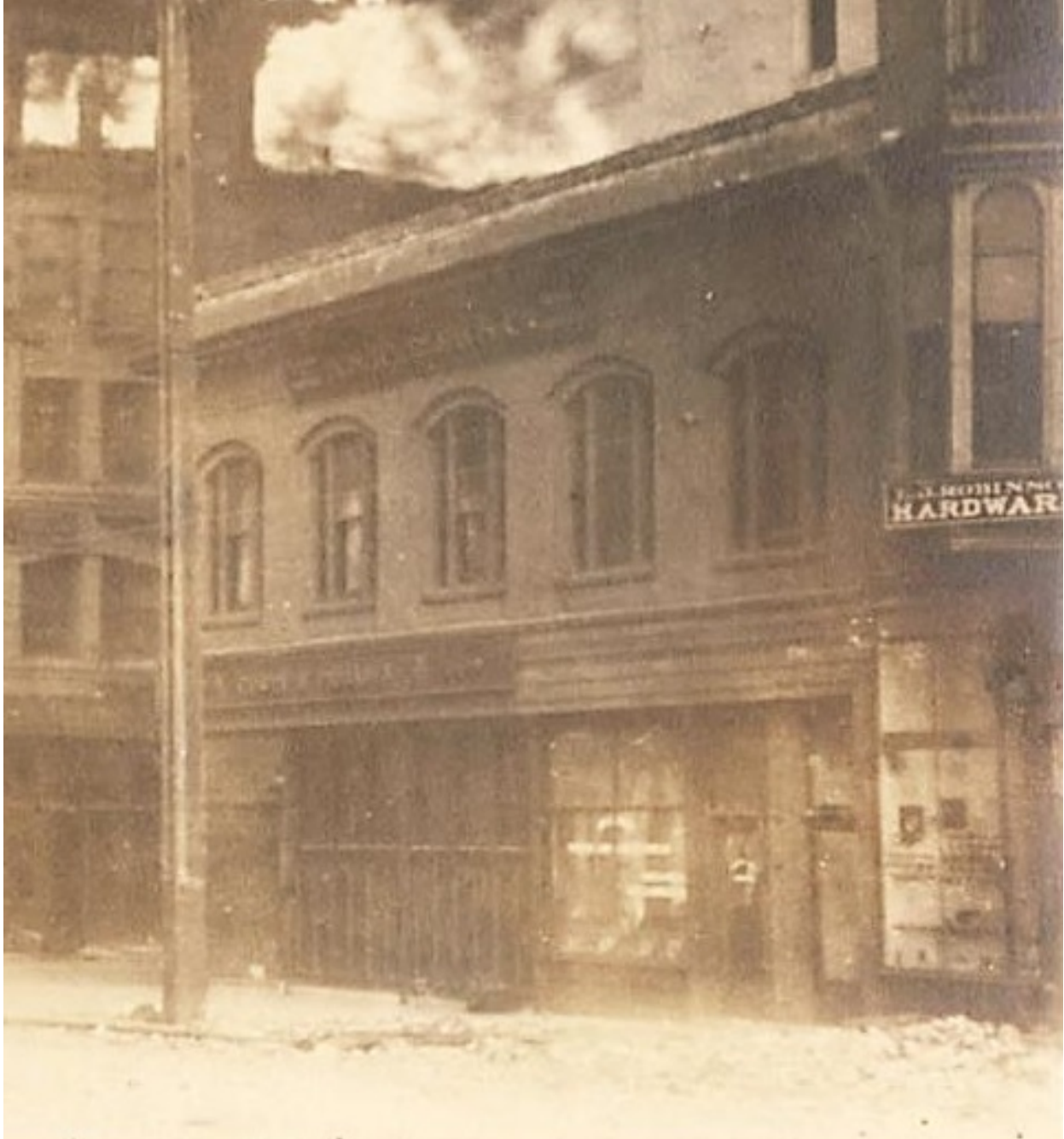
Detail view from the image on the previous page. This is the best photo available showing the original configuration of the Second Street storefront systems.
