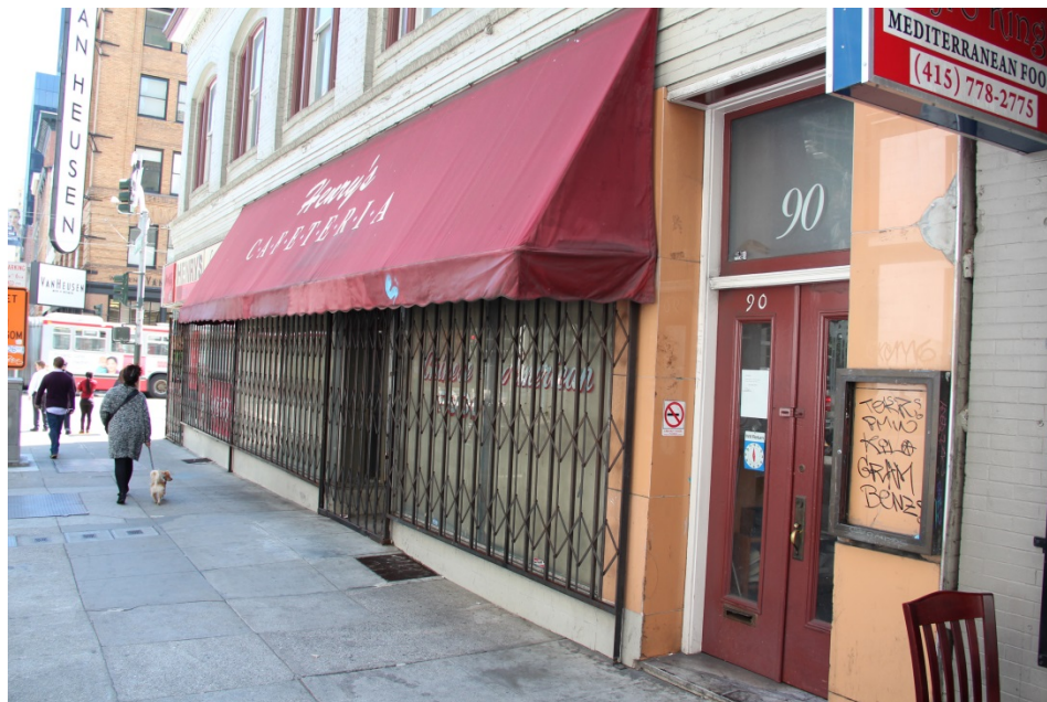
View toward Mission Street along the Second Street facade.
