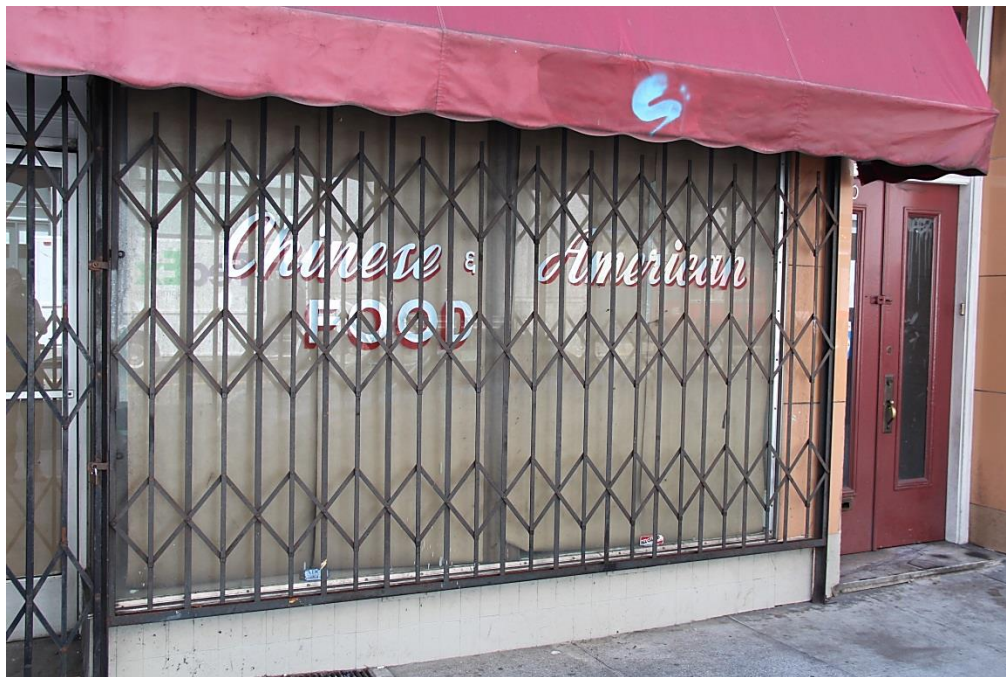
Detail of painted sign on the northern portion of the storefront at 92 Second Street. Note the stacked tile veneer on the bulkhead.
