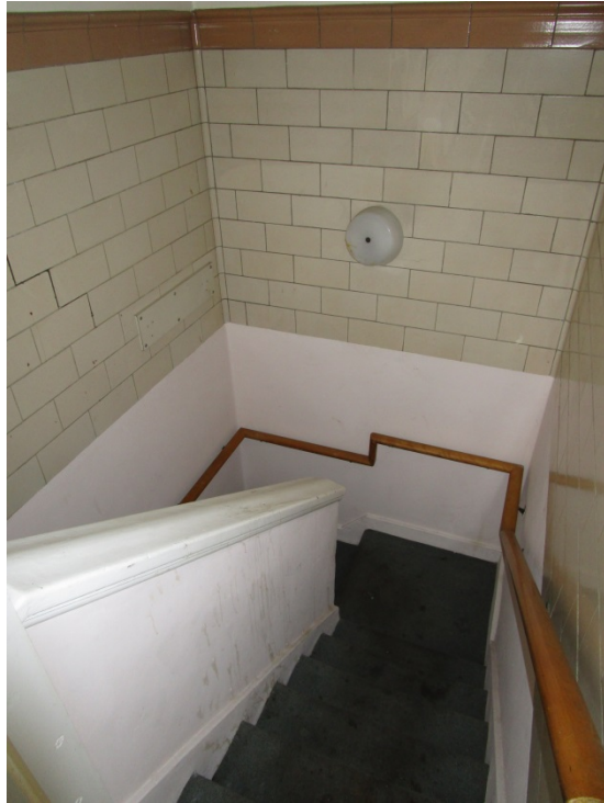
Detail of stair; note cream-colored tile with tan-colored border.
