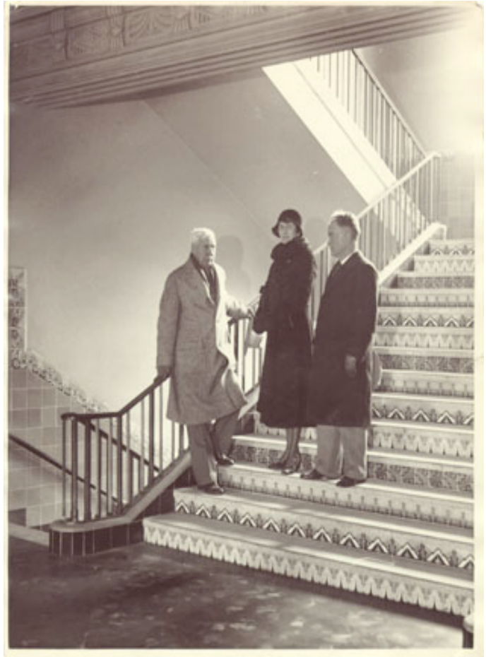
City architect presenting James Lick Junior High School to President and Commissioner of Board of Education, 1932 [AAD-4537] San Francisco History Center, San Francisco Public Library.
