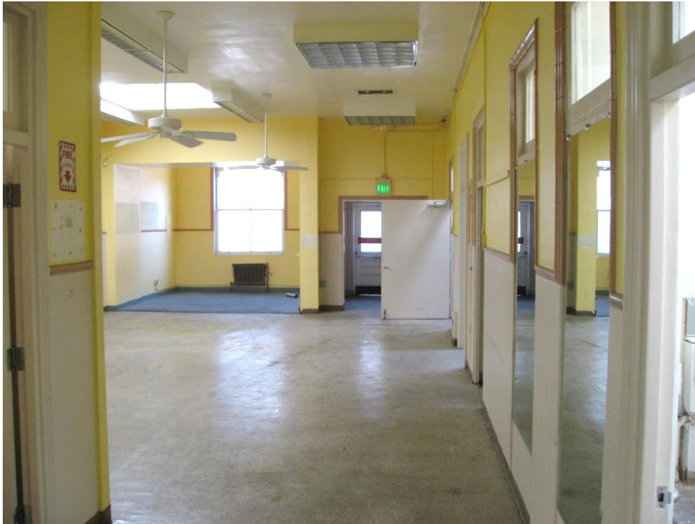
Former ward room, view northwest; note cream-colored tile with tan-colored tile borders.
