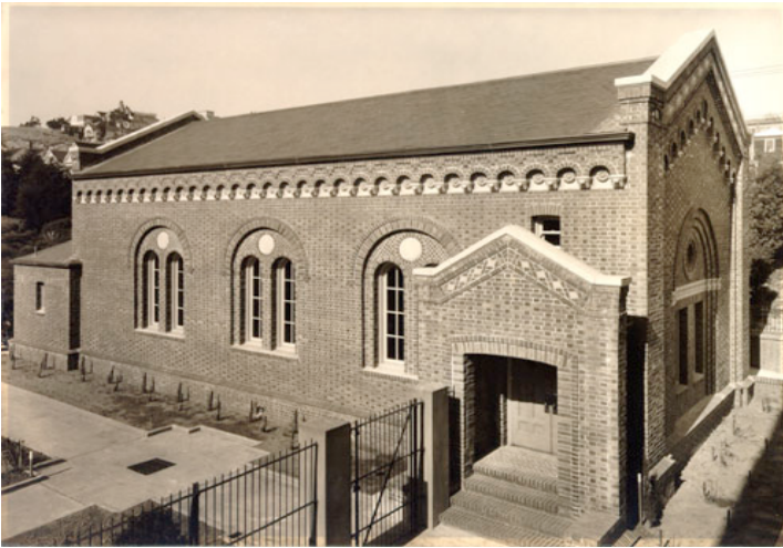
The Chapel at SF General Hospital, Charles H. Sawyer, City Architect. [AAD-0445] San Francisco History Center, San Francisco Public Library.
