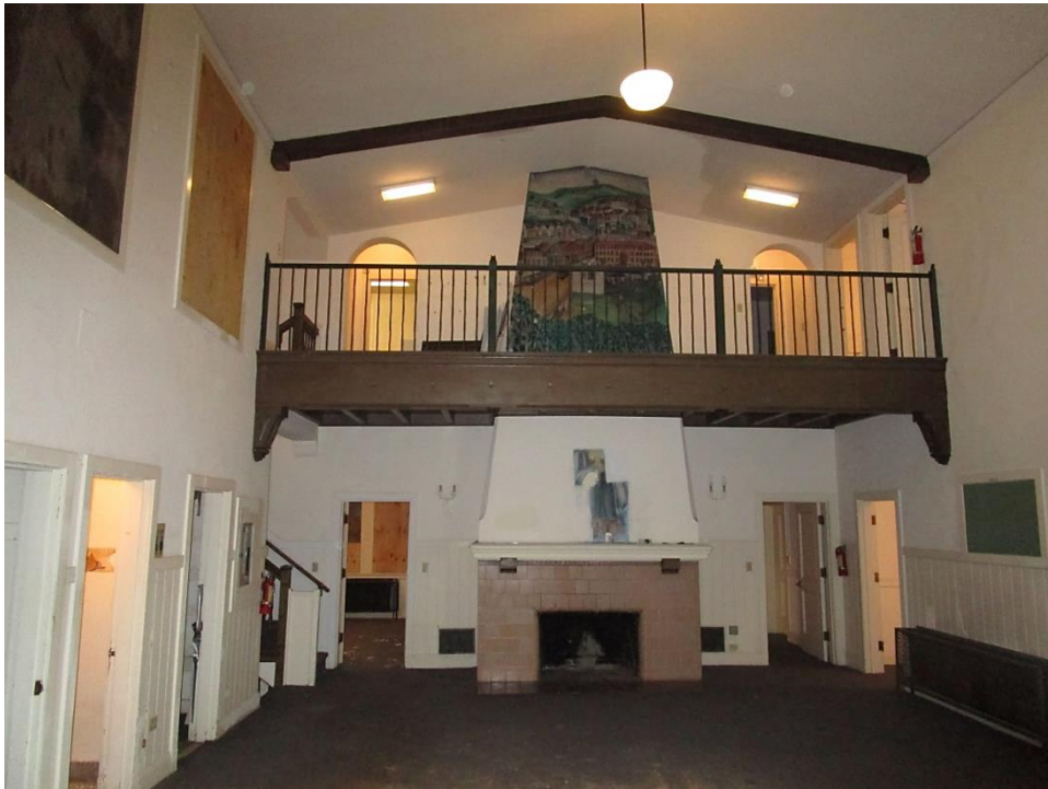
Lobby, view south; note double height volume, gable ceiling with wood beams, balcony, central fireplace with tapered chimney, metal candle scones and openings flanking fireplace and chimney, and vertical board wainscot with flat board trim throughout
