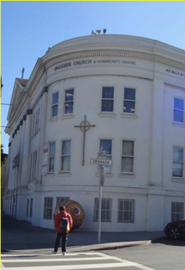
View of the building's curved northwest corner.
