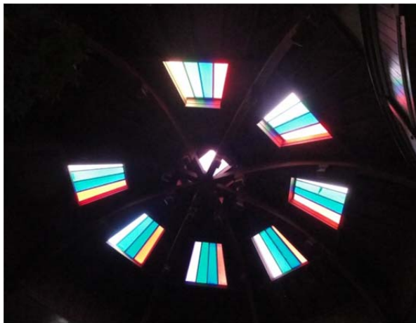
Detail of the dome's skylights.
