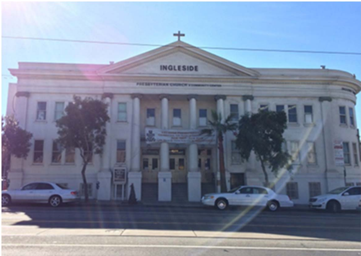
View of the primary façade along Ocean Avenue.
