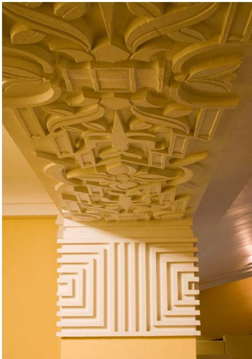
Figure 19. Detail of plasterwork in the lobby.
