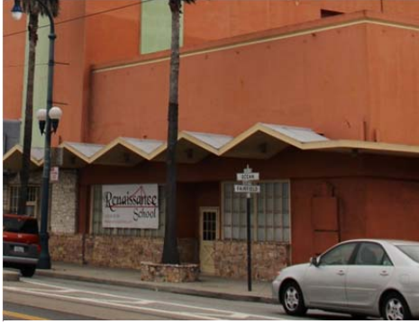
Figure 11. East retail wing, looking west.
