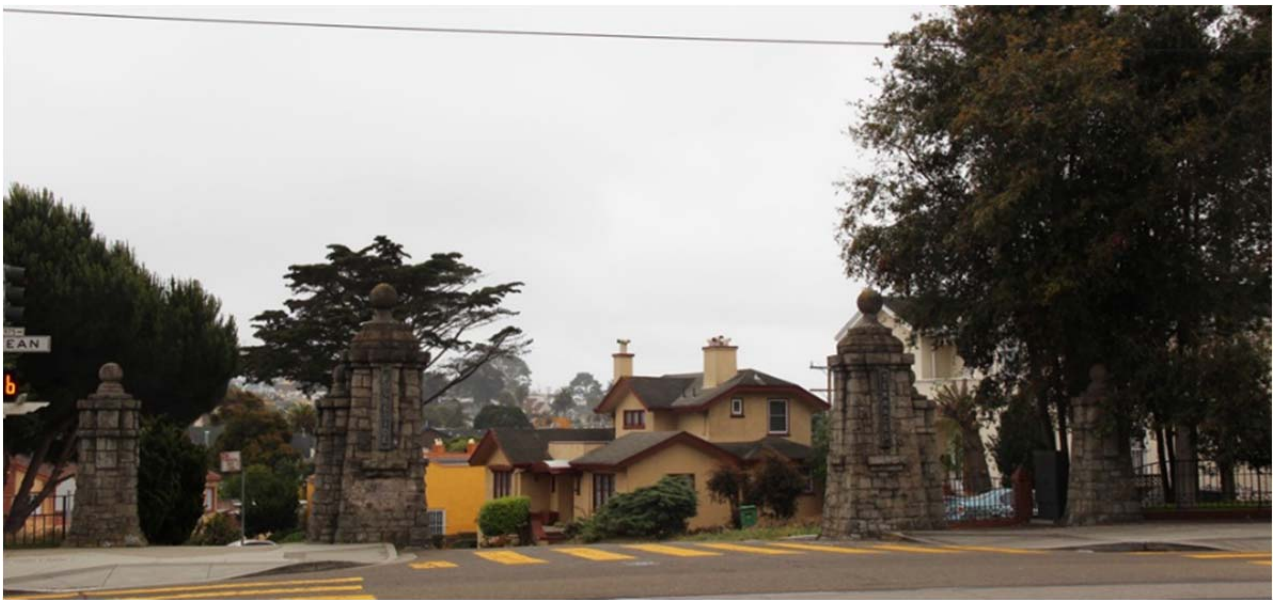
Figure 4. Victoria Street entrance to Ingleside Terraces, looking south.
