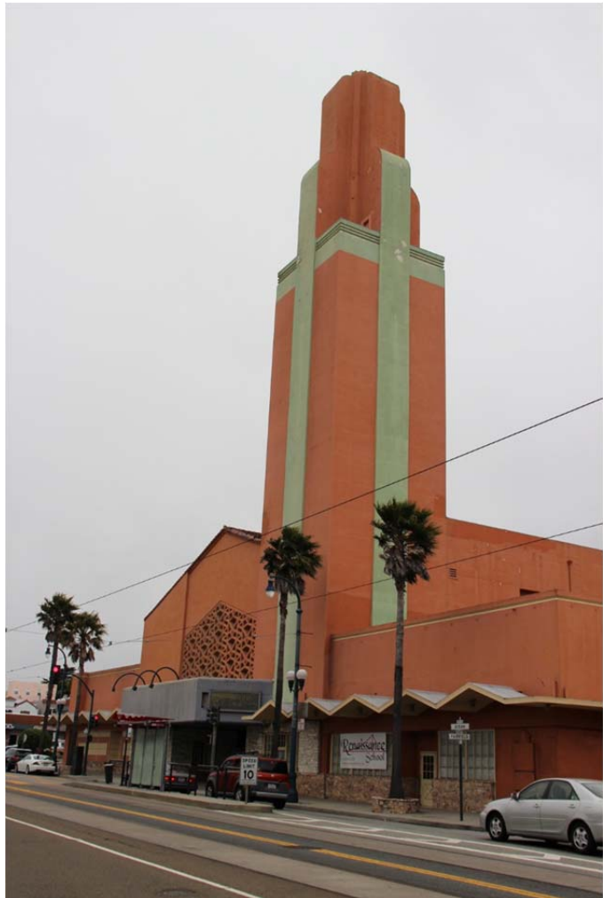
Figure 6. Primary façade of El Rey Theater, looking west.
