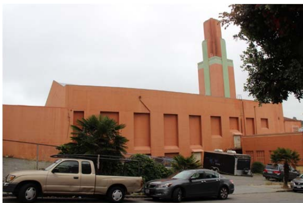
Figure 16. West wall of auditorium, looking southeast.
