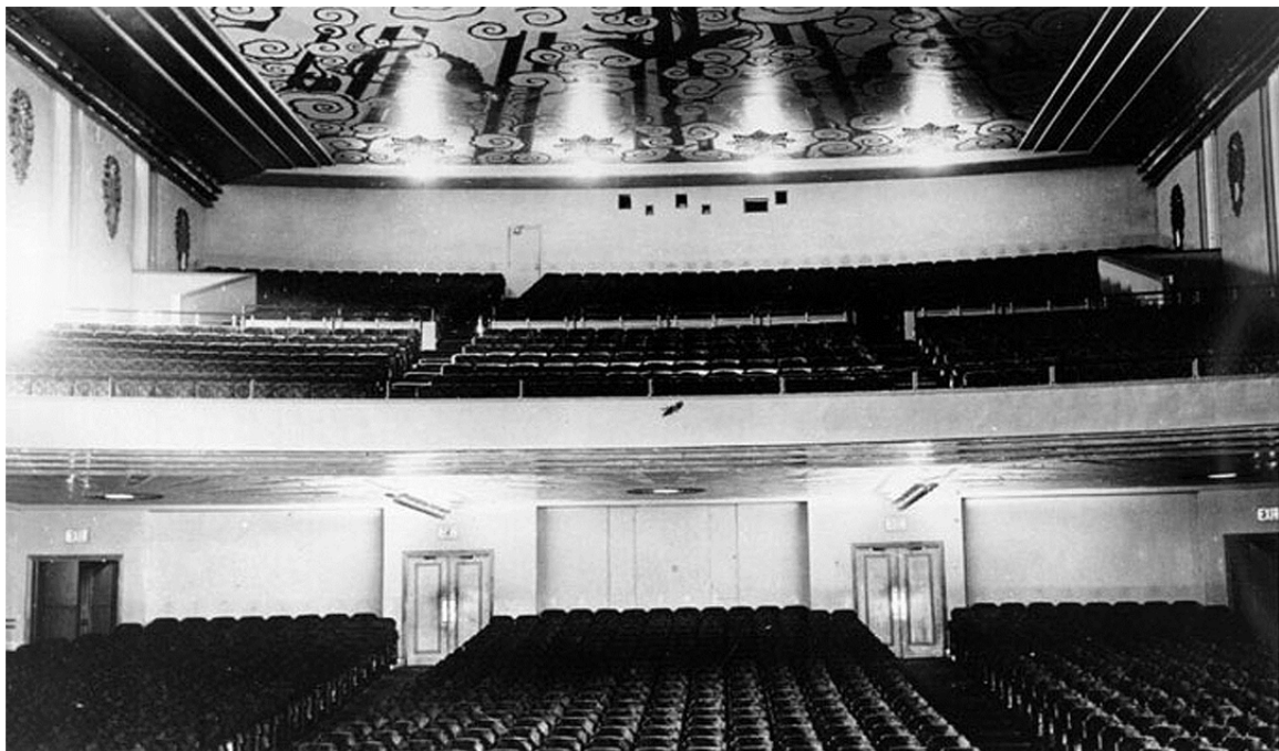
Figure 32. El Rey Theater Auditorium, looking south, 1942.
