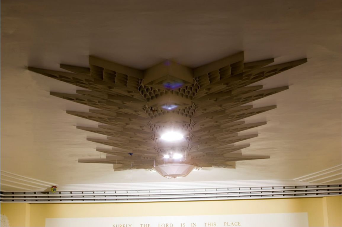
Figure 24. Sheet metal light fixture on ceiling of auditorium, looking north.
