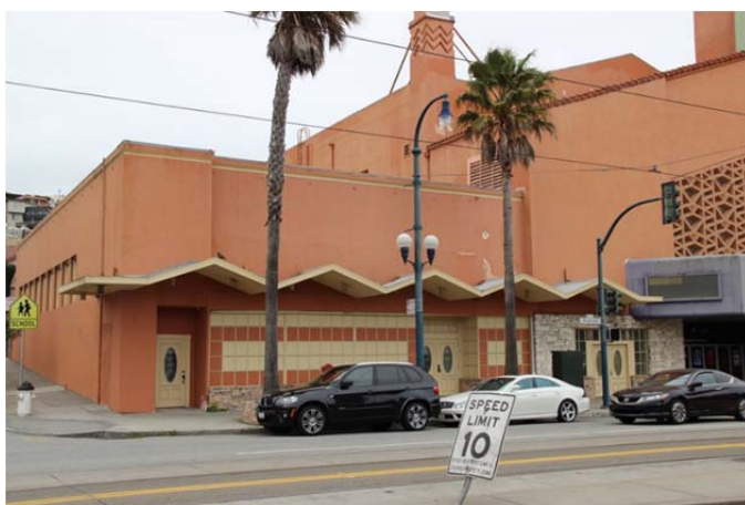
Figure 7. South wall of west retail wing, looking north.
