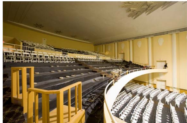
Figure 23. Balcony, looking southwest.
