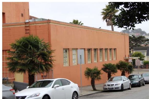
Figure 17. West wall of west retail wing, looking south.
