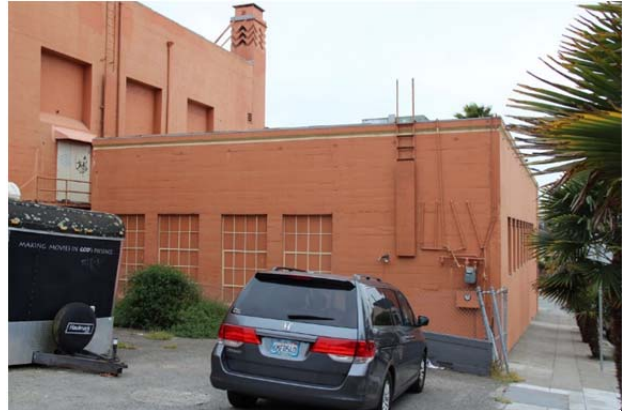
Figure 15. North wall of west retail wing, looking south.
