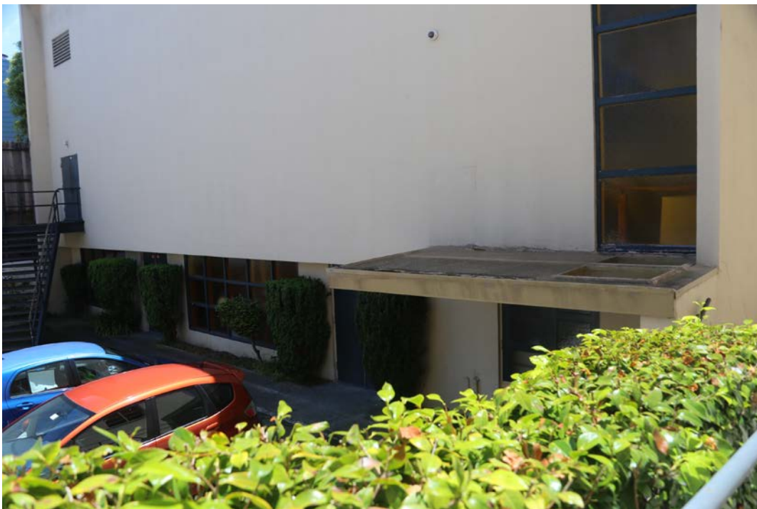
North elevation, canopy detail. View southeast.
