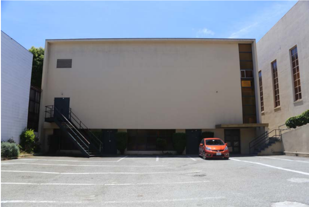
North elevation youth center and fellowship building, view south.
