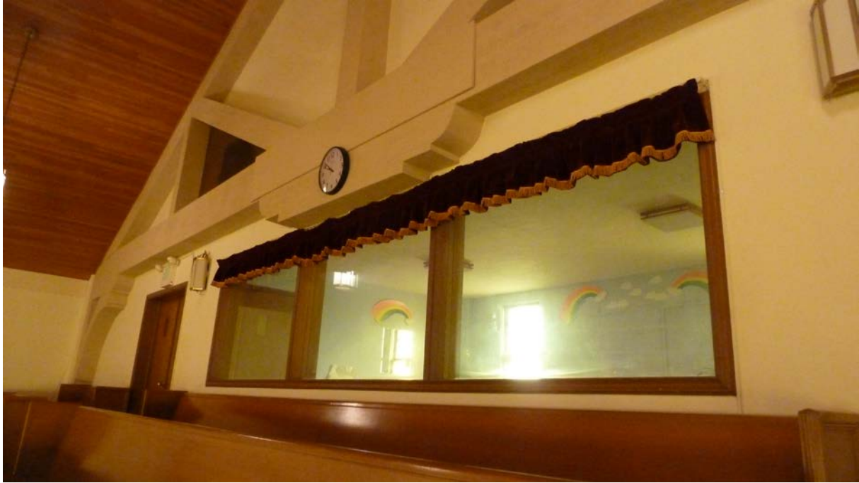
Window into children's room on mezzanine. View northwest.
