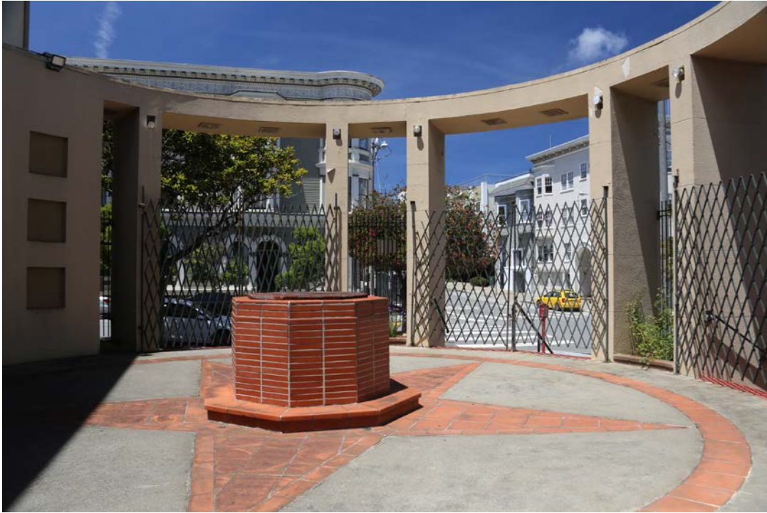
Octagonal baptismal font clad in Roman brick and terracotta star inlaid in concrete platform in the courtyard directly in front of the entrance to the church building. View northwest.
