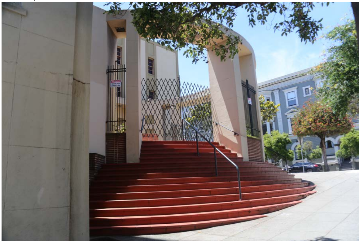
Brick staircase, courtyard, columns, and curvilinear entablature at church entrance. View southwest.
