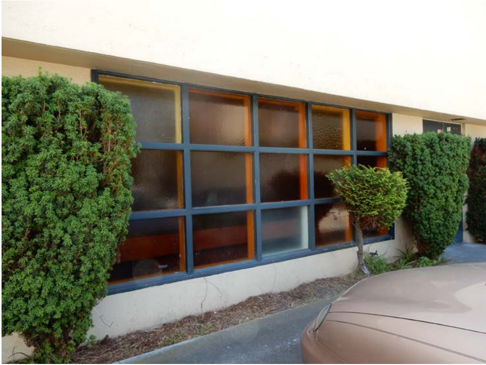
Multi-lite, wood sash windows with textured yellow glass at first floor, near northwest corner of north façade, view southwest.
