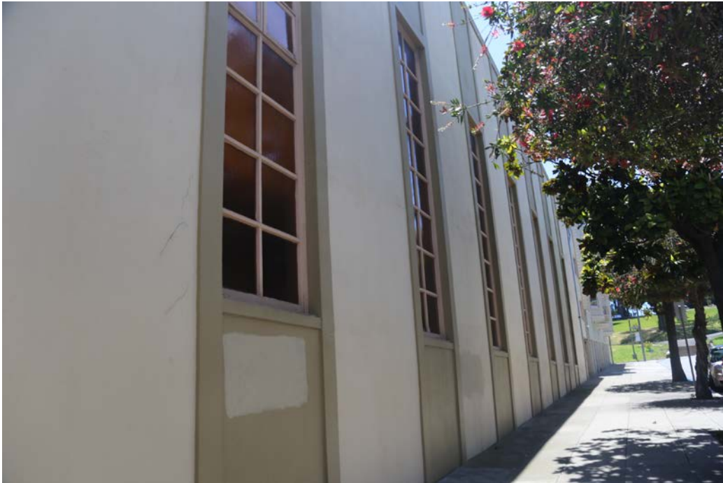
Detail of west façade of main church building. View southeast.
