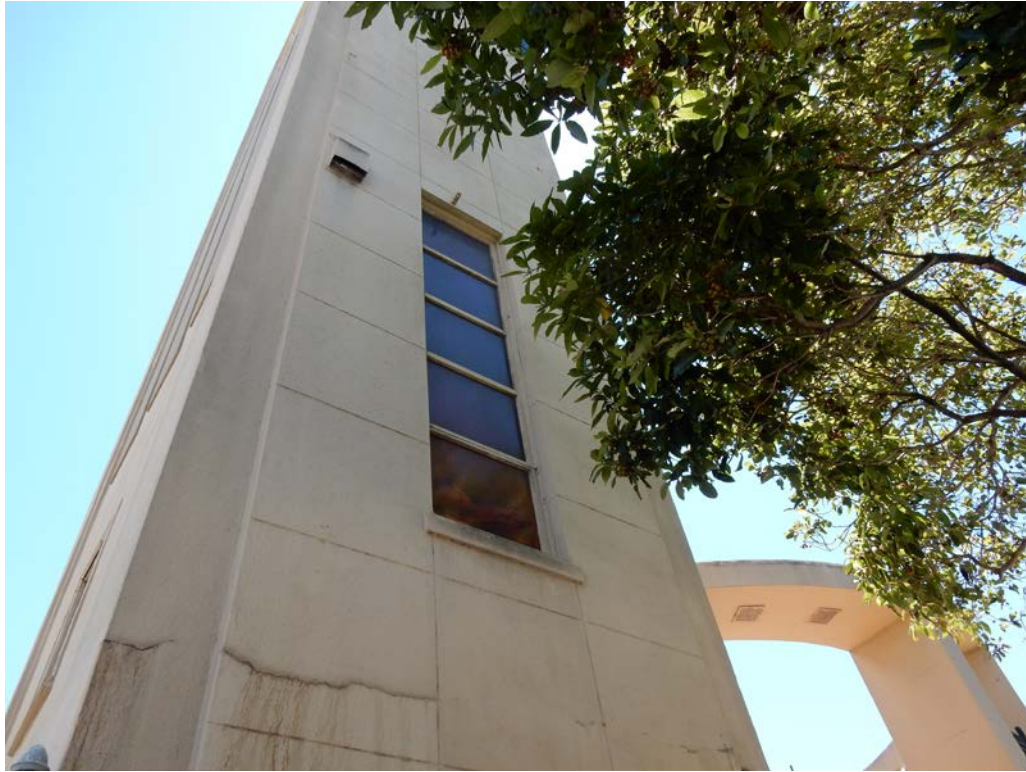
Detail of vertical wooden ribbon windows on bell tower. View southwest.
