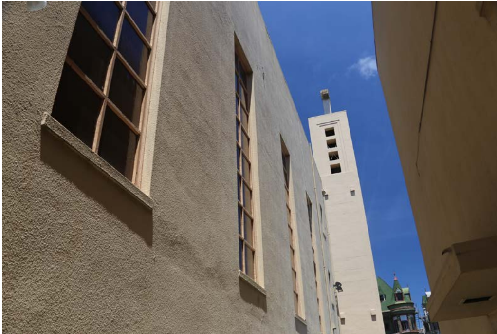
East elevation of church building, vertical wood ribbon windows with divided lites and yellow glass, and south elevation of bell tower. View northwest.
