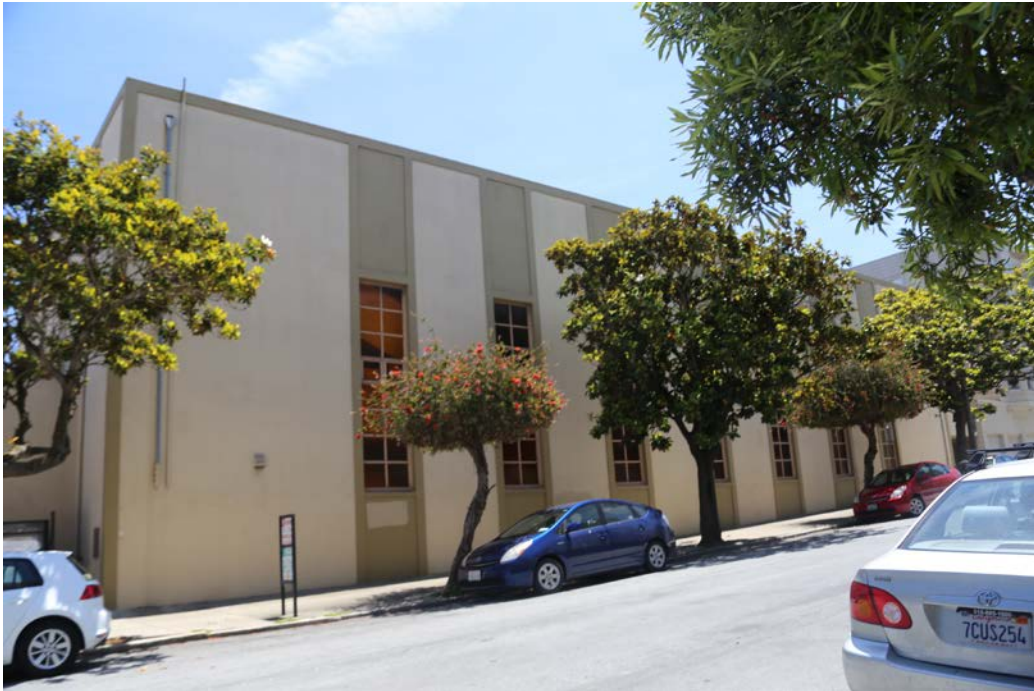
West façade of main church building. View east.
