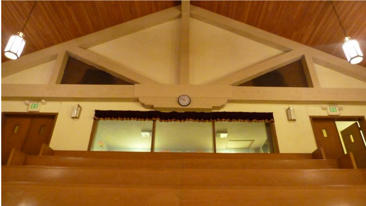
Mezzanine. View north.
