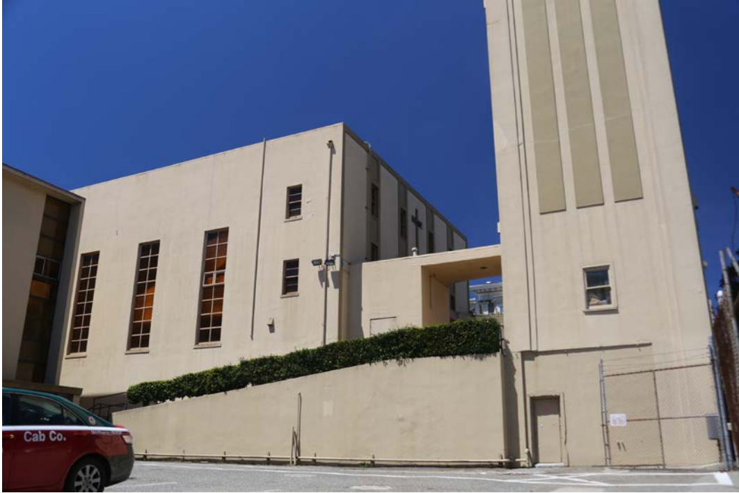
East elevation of church building and bell tower as seen from parking lot located on the church property. View west.
