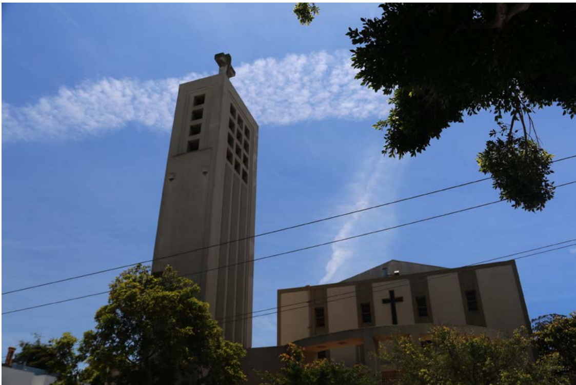
North elevations of bell tower and main church building. View south.
