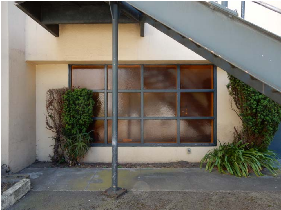
Multi-lite, wood sash windows with textured yellow glass at first floor. Northeast corner of north façade. View south.
