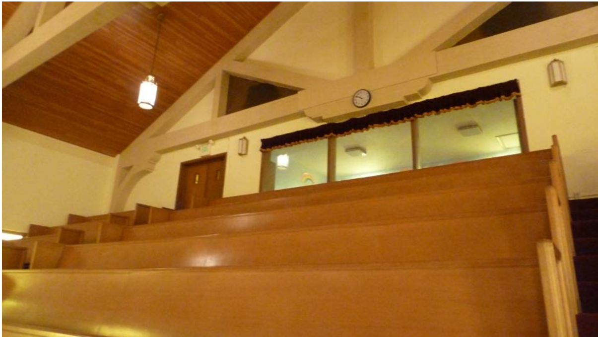
Mezzanine. View northwest.
