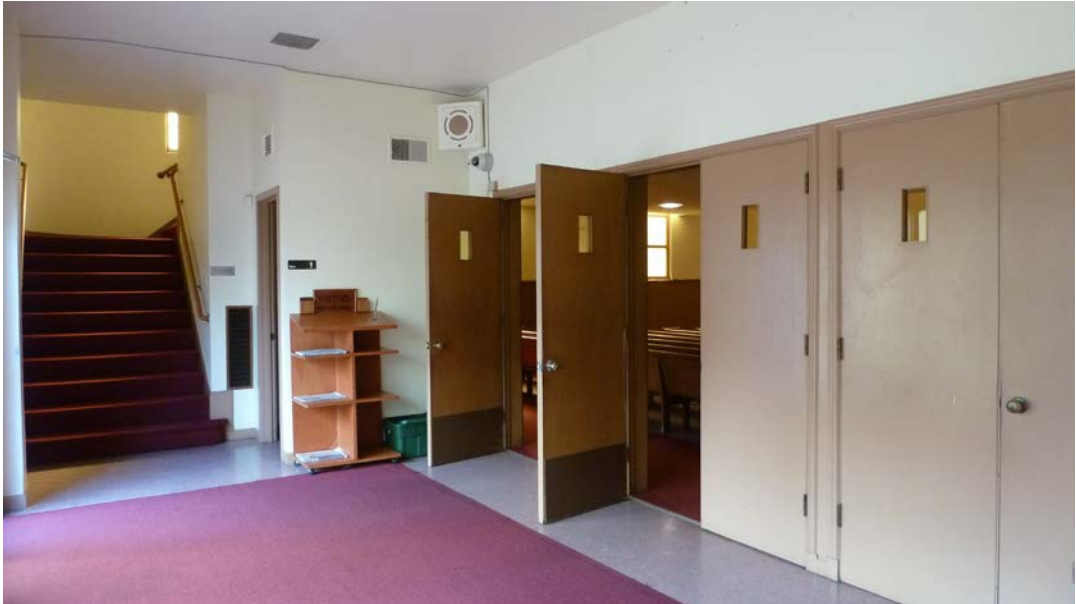
Church lobby and staircase to mezzanine. View southeast.
