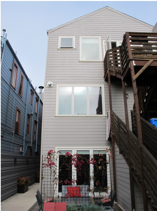
Figure 29: South side fenestration.
