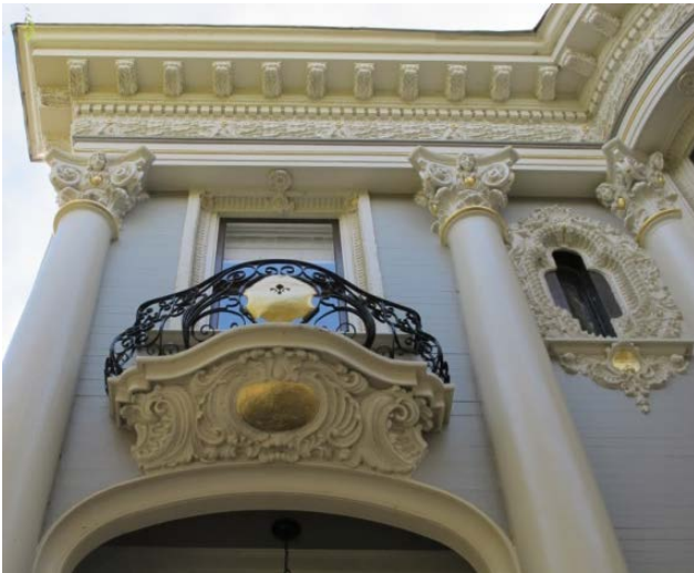
Figure 16: North side of primary façade.
