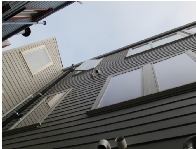
Figure 24: Second and third story fenestration of south façade.
