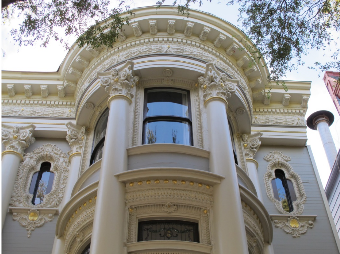
Figure 18: Bay flanked by oval windows in elongated quatrefoil surrounds (south window has a simpler surround).
