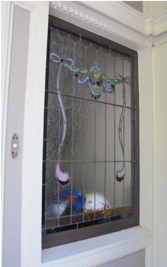
Figure 11: Fixed leaded stained glass window within entry area.
