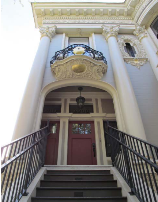
Figure 14: Molded balcony with flanking engaged columns.
