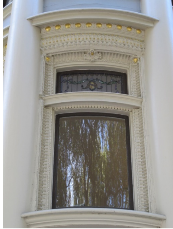
Figure 13: Second story rounded bay window with transom.
