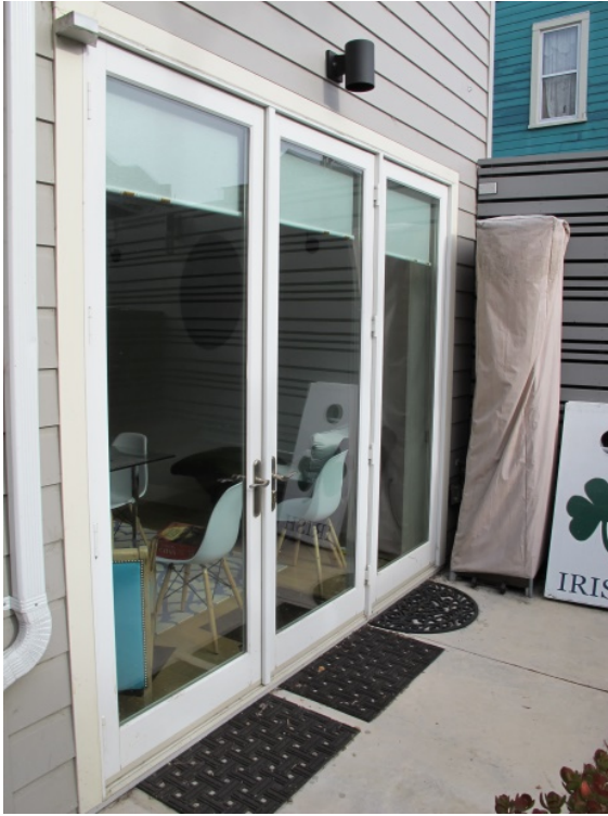
Figure 31: North side ground level.
