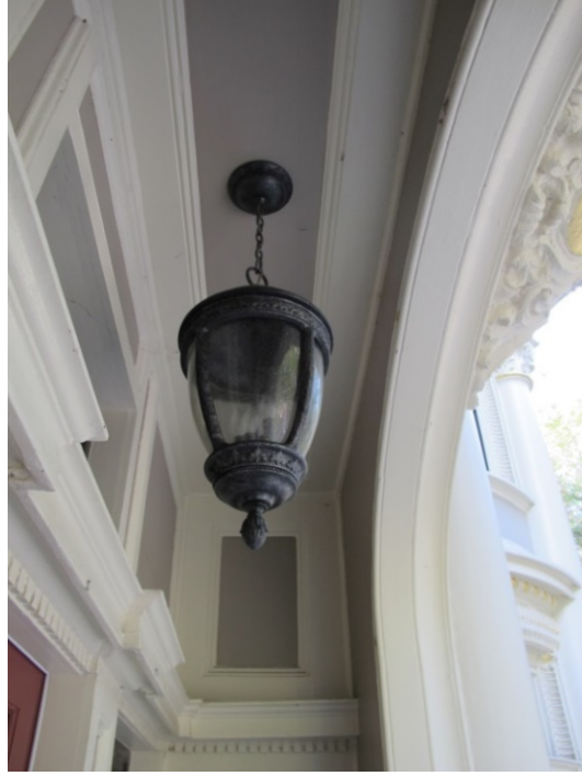
Figure 10: Recessed entry area to Units 2731 and 2733.
