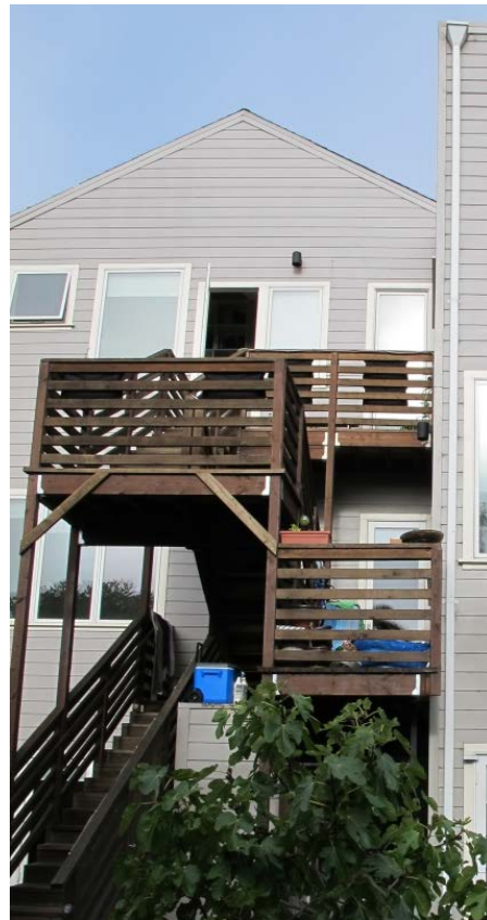
Figure 30: South side fenestration.
