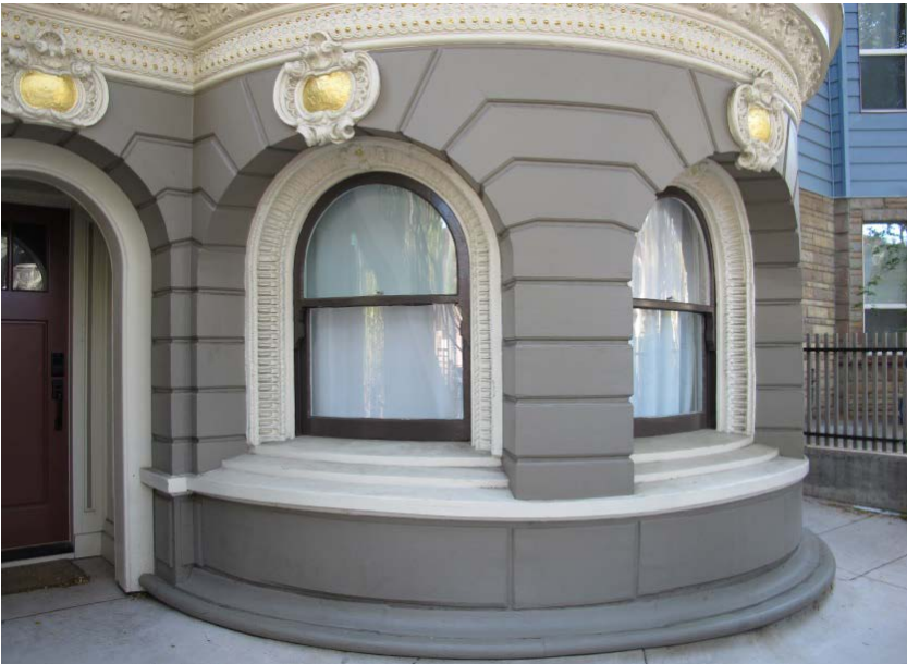
Detail of rusticated base
