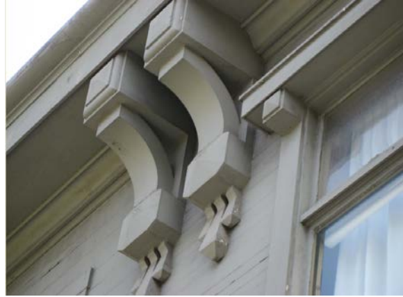
Detail of cornice brackets
