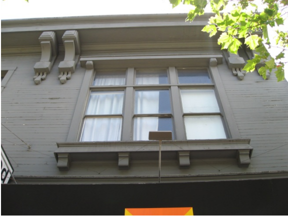
Detail of window and cornice
