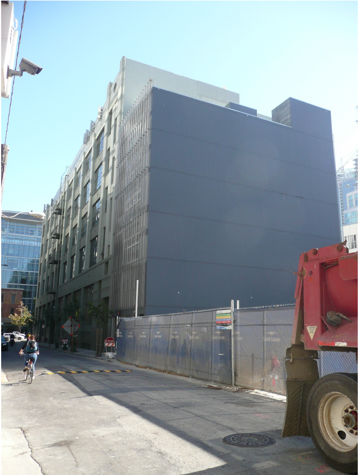
A8. View of west façade, looking east (ARG, October 2015).
