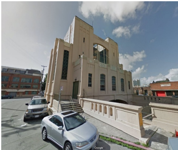
Posey Portal Superstructure, North End (Alameda and Oakland, 1928)
