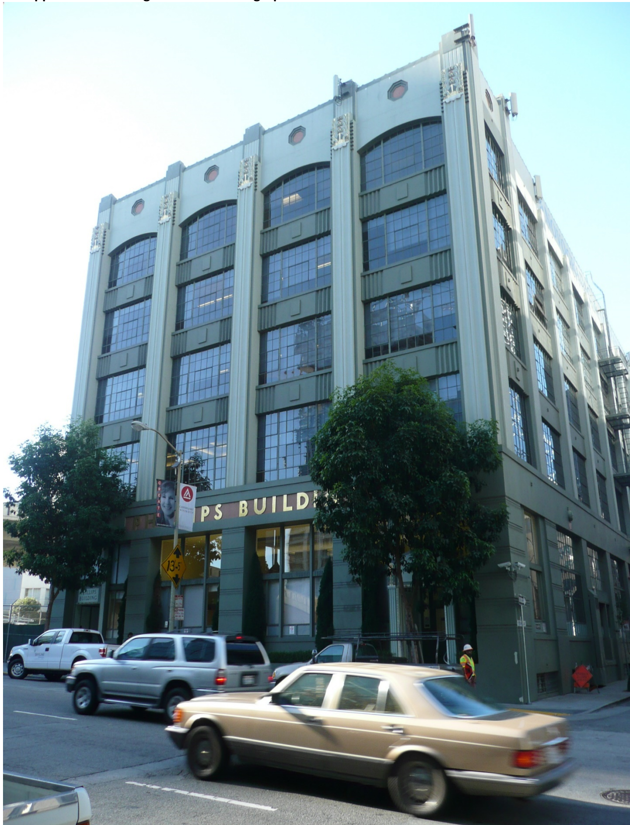
A1. View of front (east) façade, looking south (Architectural Resources Group, October 2015).
