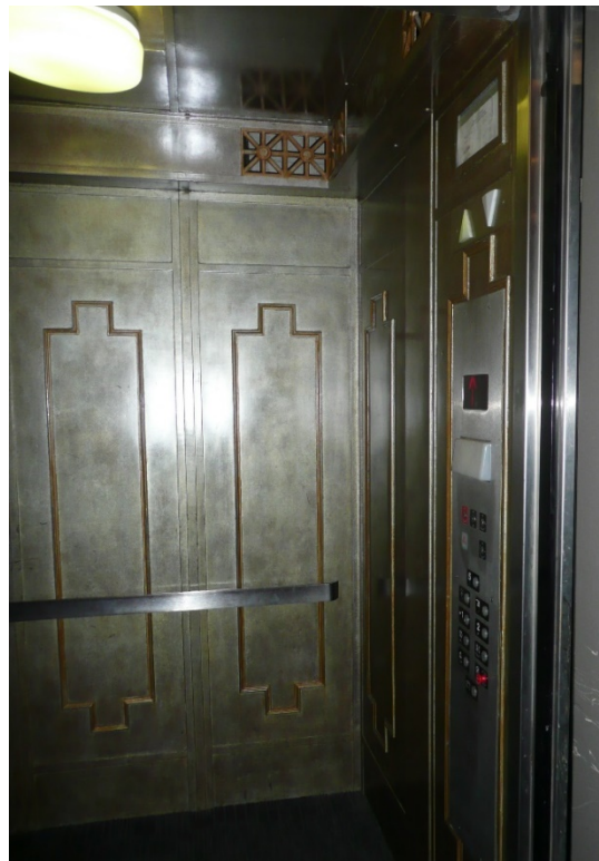
A19. View of interior of elevator cab (ARG, October 2015). Permit research and review of historic drawings did not confirm that the current metal panels are original.
