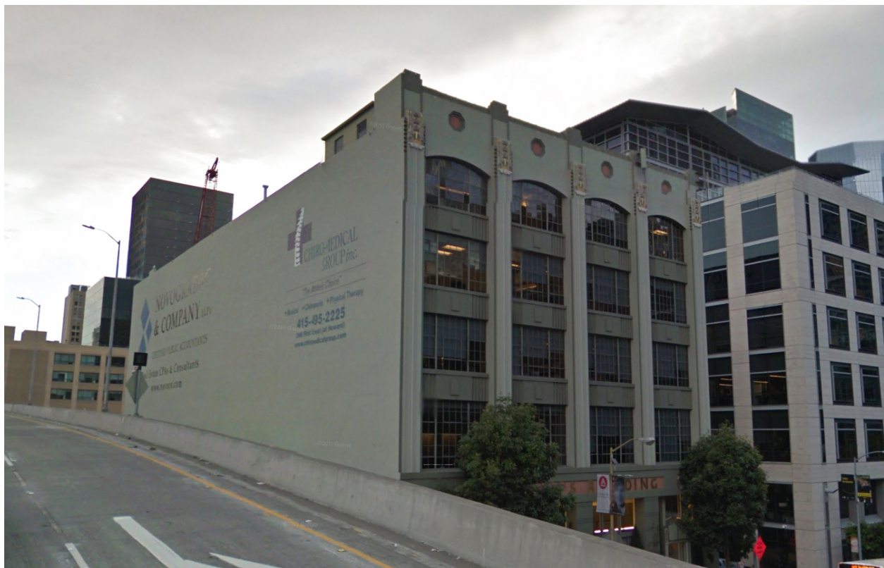
A10. View of south façade, looking west (Google street view, accessed October 2015).
