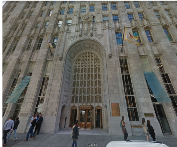
Pacific Telegraph and Telephone Building, Detail (140 Montgomery Street, 1925)
