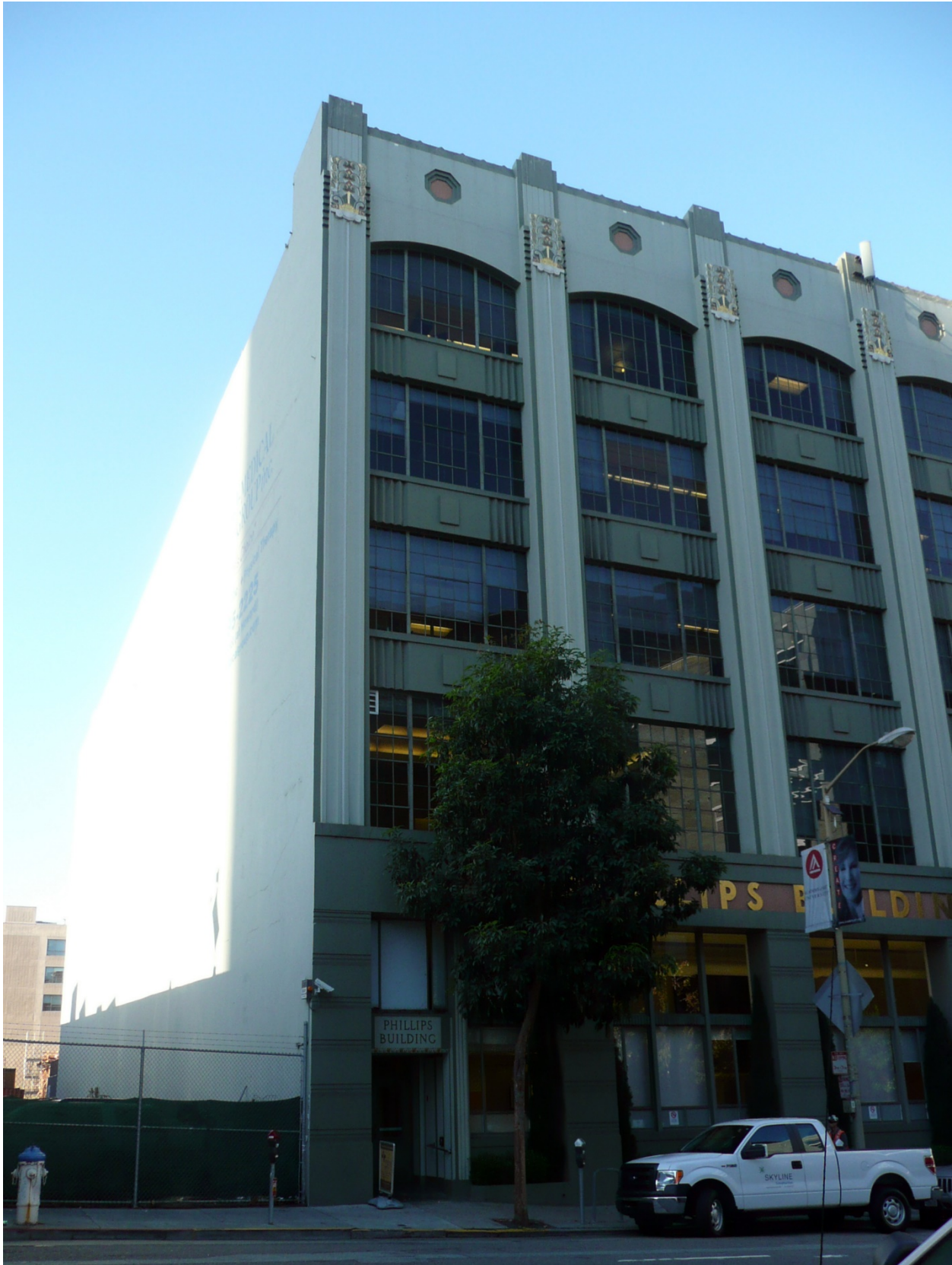
A2. View of front (east) façade, looking west (ARG, October 2015).
