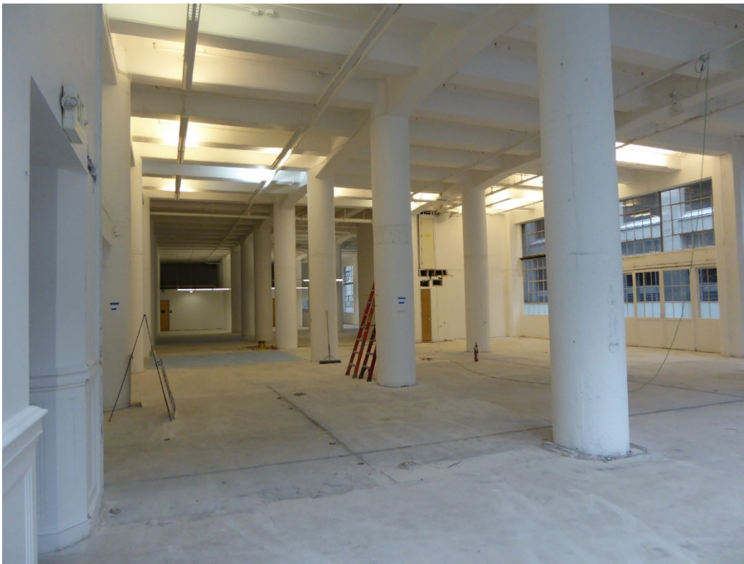
A15. Interior view of first floor, looking west towards the rear of the building (ARG, February 2017).
