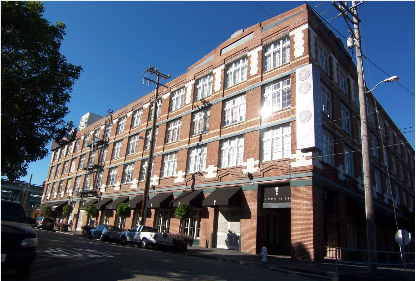
South facade (l), east facade (r)
