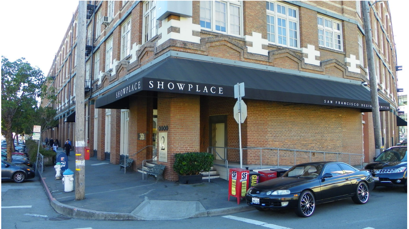
Detail: Triangular arches & ornament dividing base from upper zone
