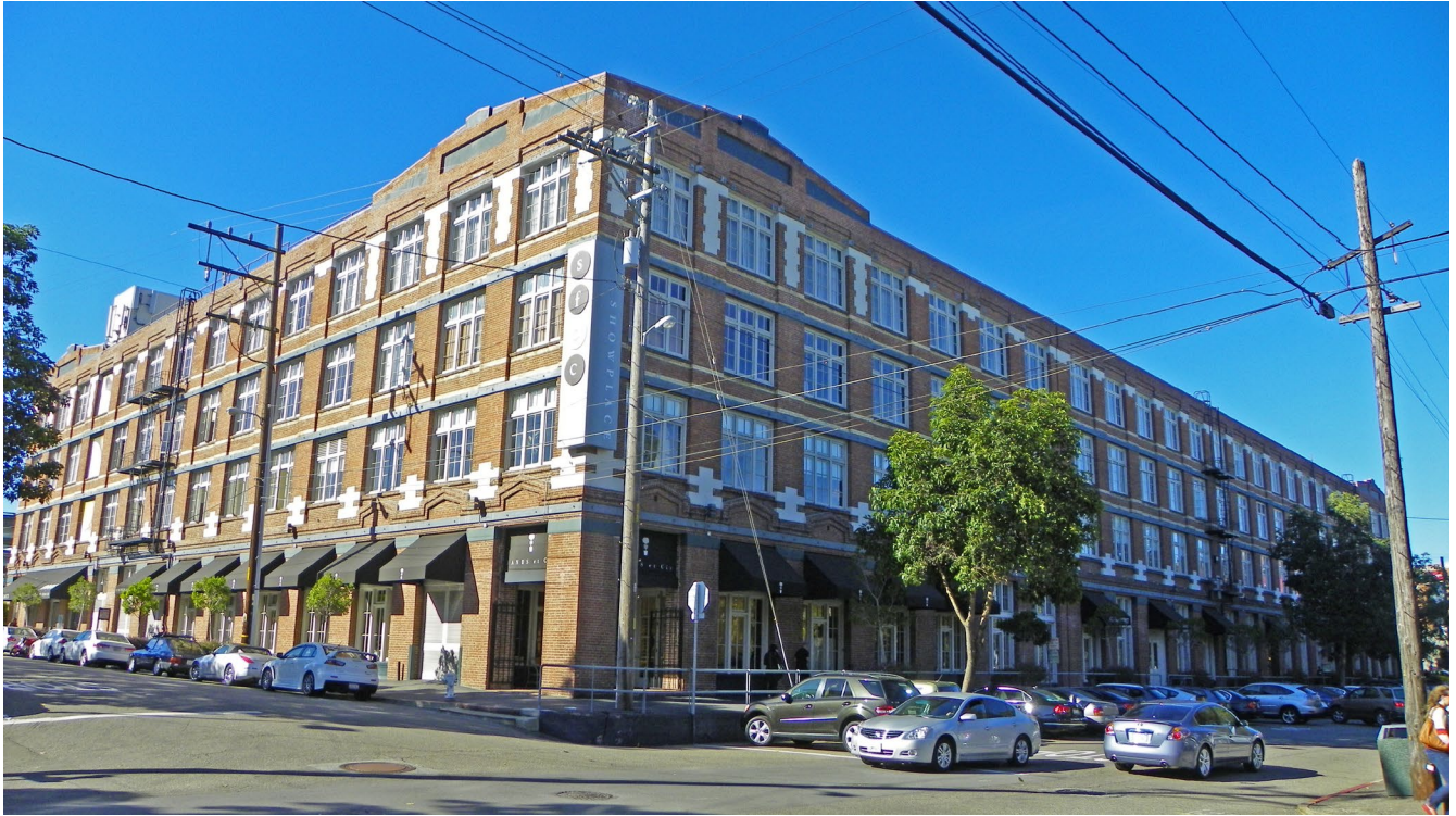
East facade (r), south facade (l)
