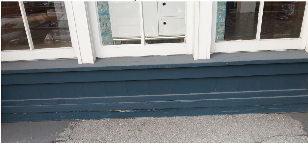
Solid wood bulkhead
