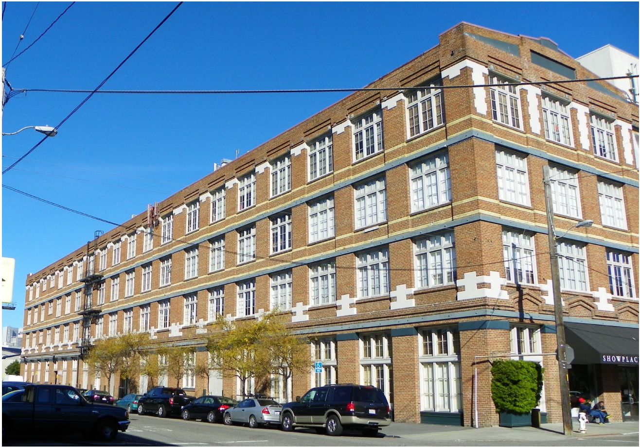
West facade (l), south facade (r)
