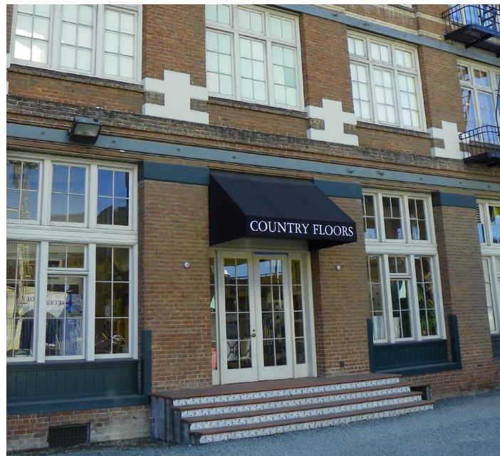
Detail: Contemporary exterior stair, northwest facade
