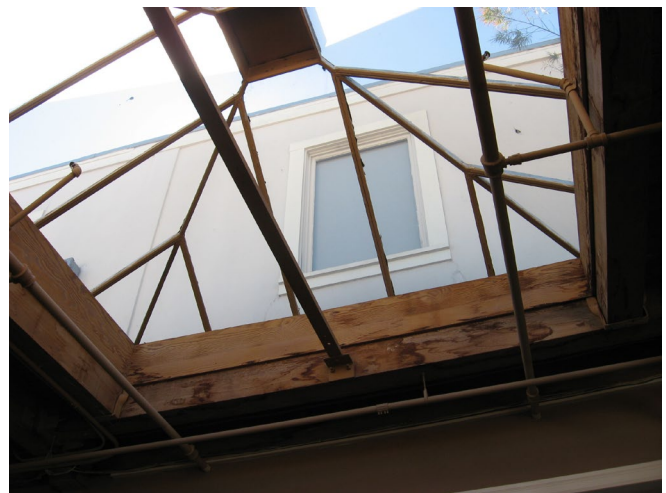
Example of skylight on fourth floor.
