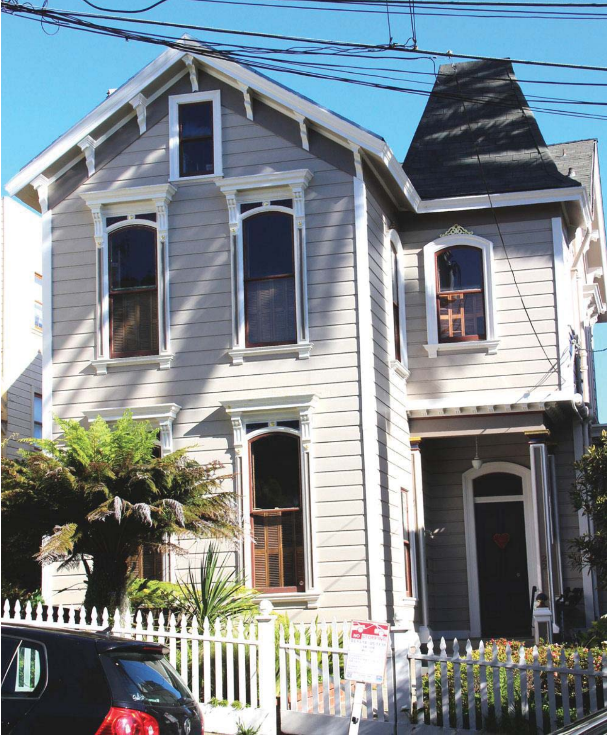
Figure 25. South (primary) façade of the Benedict-Gieling House; view toward north.
