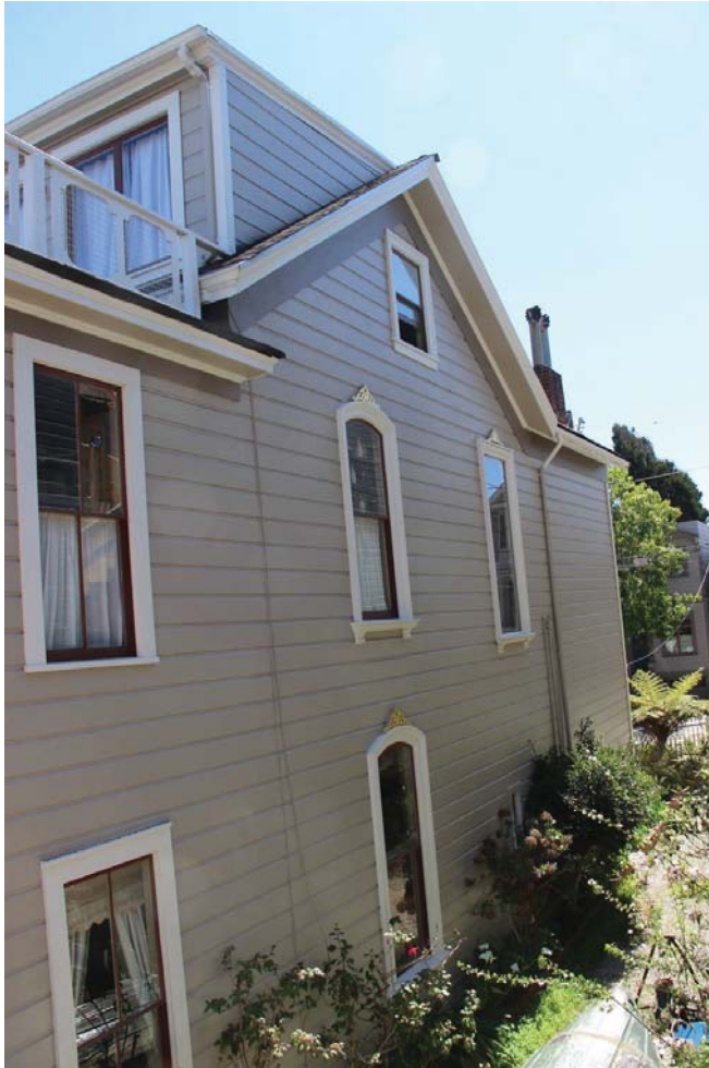
Figure 32. West façade; view toward south.
