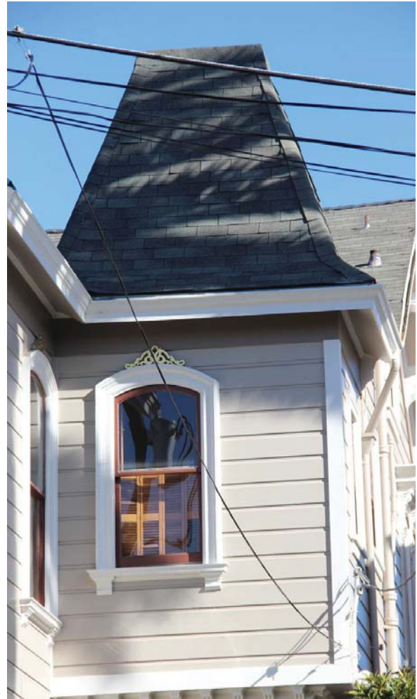
Figure 27. Tower; view toward north.
