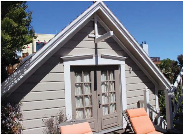
Figure 54. Primary façade of carriage house; view toward northeast.
