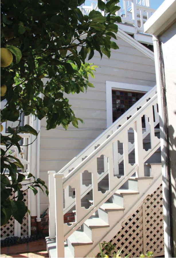
Figure 35. 1933 kitchen addition; view toward south.
