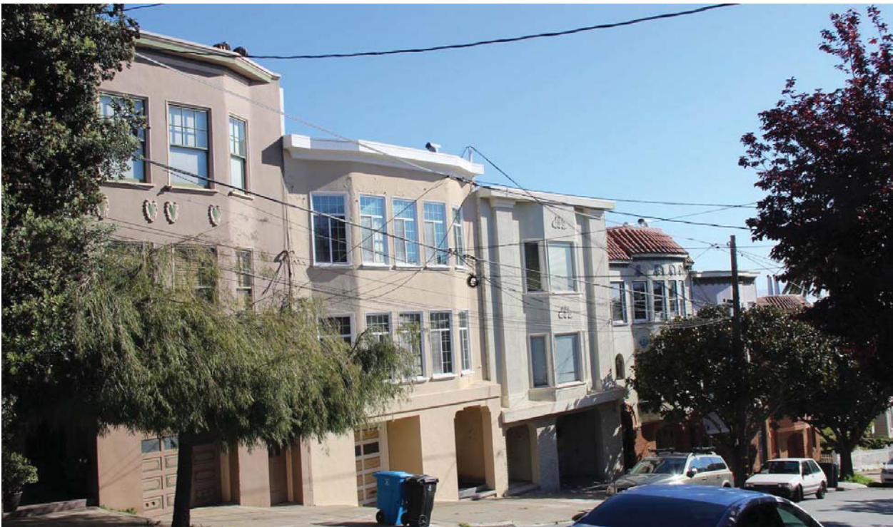
Figure 13. Row of Mediterranean-style flats at 46-48 to 68-70 Beaver Street; view toward northeast.
