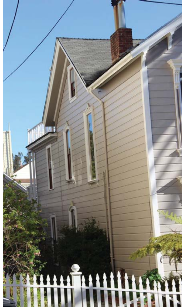
Figure 33. West façade; view toward north.
