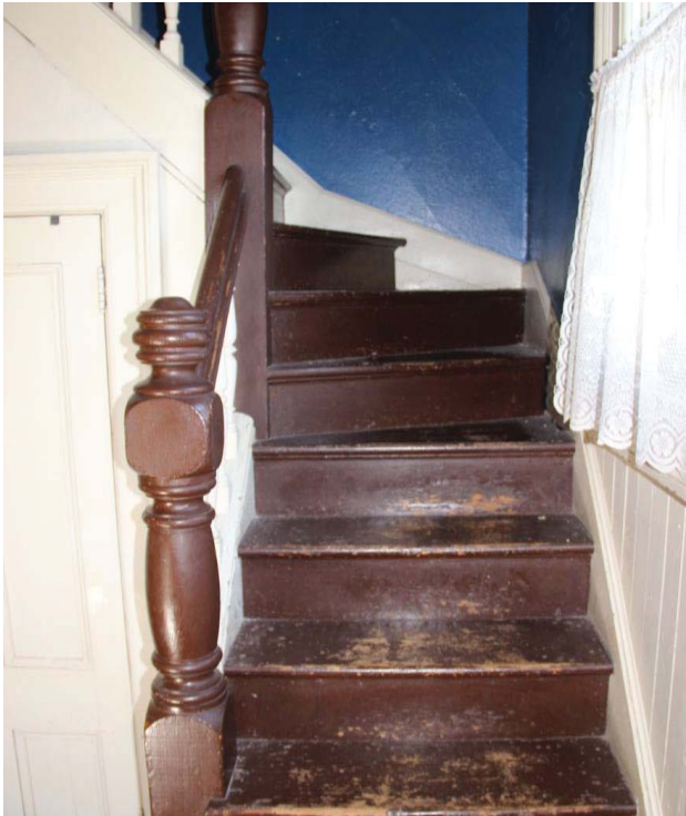
Figure 50. Attic stair; view toward north.
