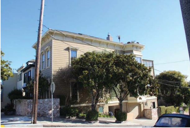
Figure 11. 245 Castro Street; view toward northeast.
