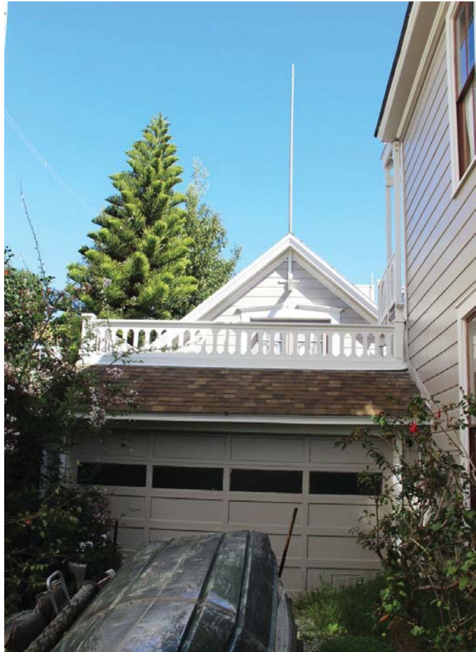
Figure 52. Garage/carriage house; view toward north from driveway.
