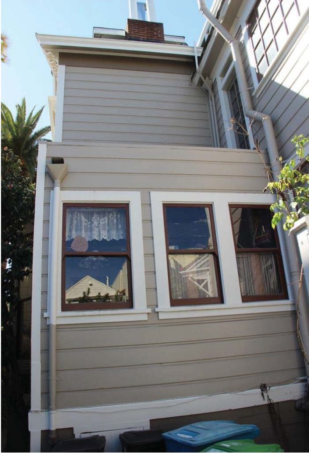
Figure 34. Ca. 1906 bathroom addition; view toward south.
