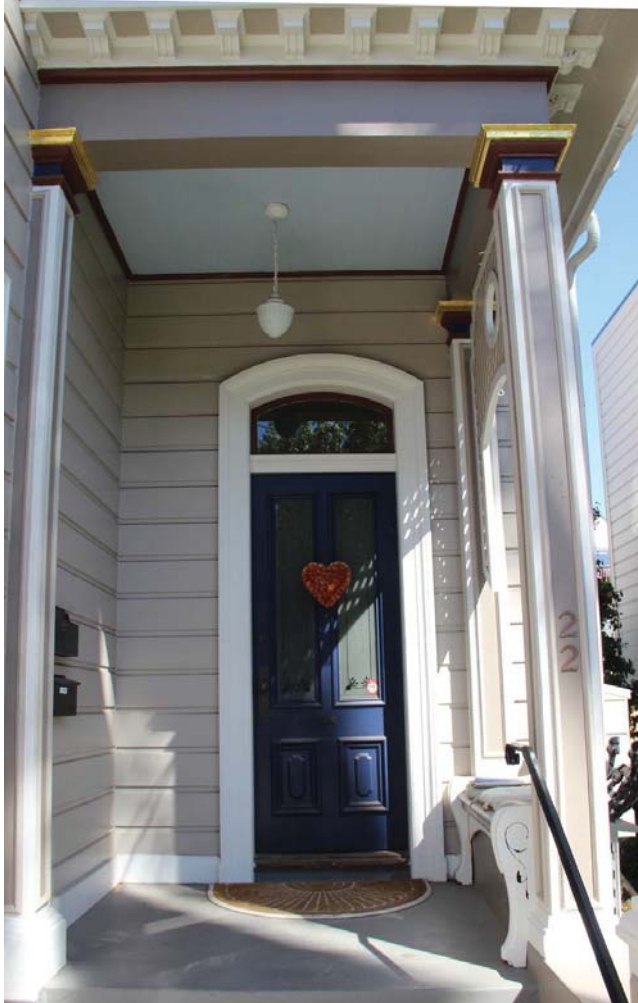
Figure 26. Main entrance; view toward north.
