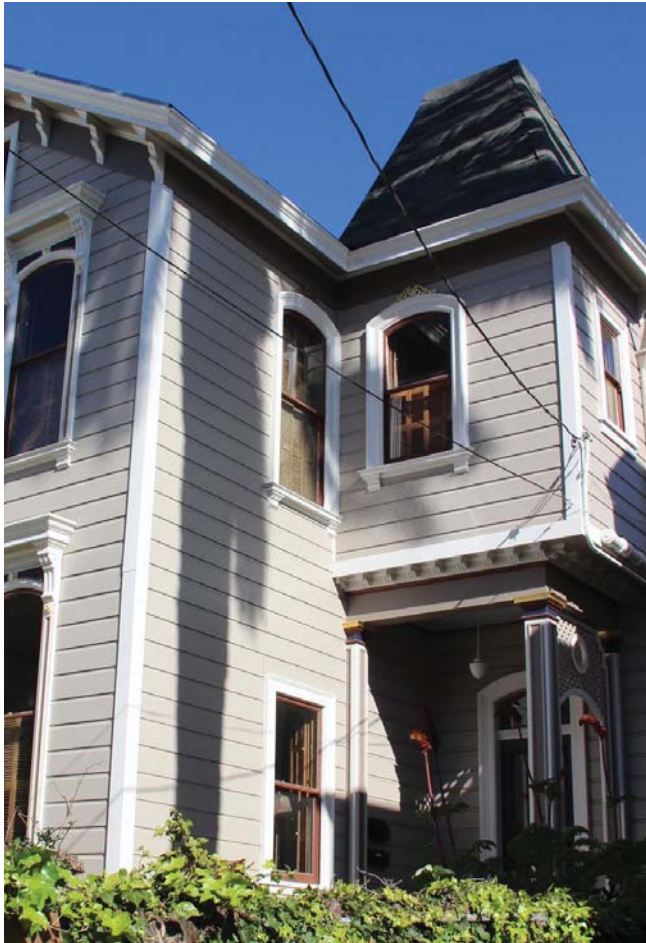
Figure 29. Front part of east façade; view toward northwest.
