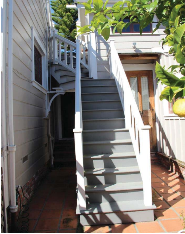
Figure 23. Patio and stair; view toward west.
