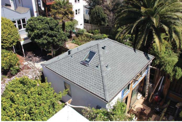
Figure 14. Cottage at rear of 20 Beaver Street.
