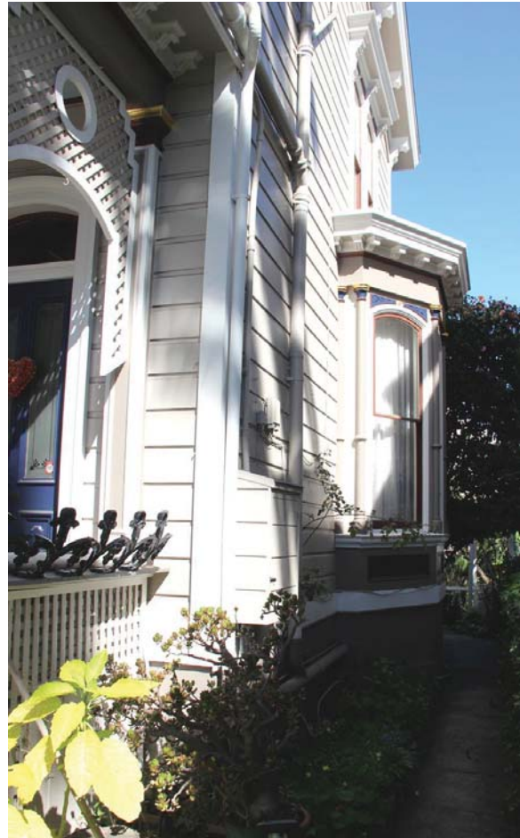
Figure 30. Bay window; view toward north.
