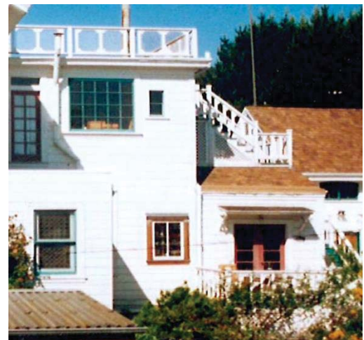
Figure 31. Detail of east façade of service wing; view toward west.
