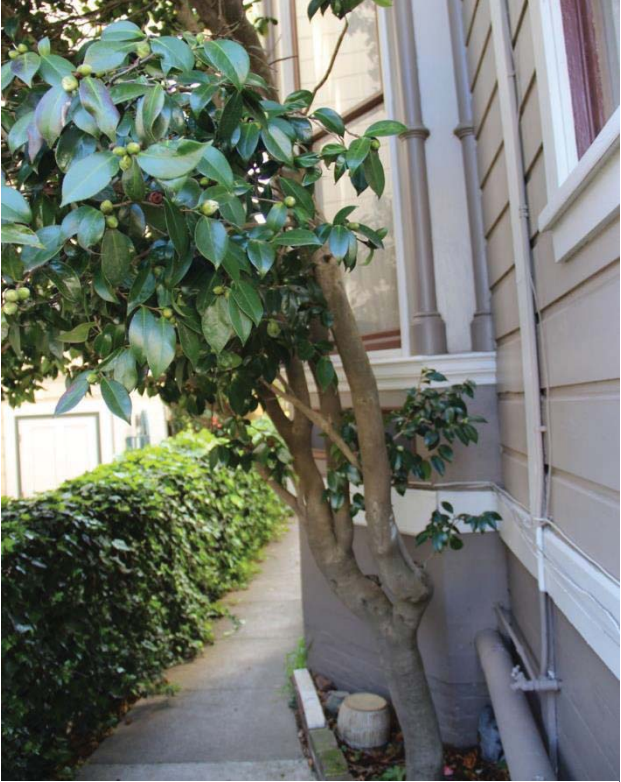
Figure 22. Pedestrian walkway; view toward south.
