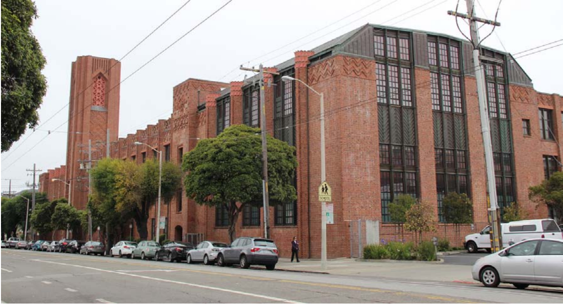
Figure 16. West façade of Theodore Roosevelt Middle School; view toward northeast.
