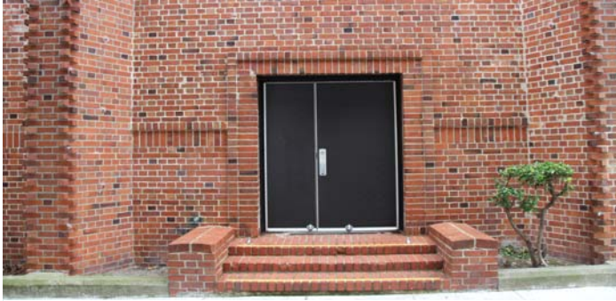
Figure 20. Metal door on primary façade.
