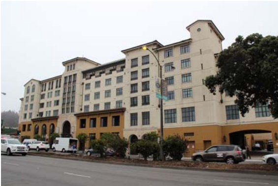
Figure 8. 3575 Geary Boulevard, constructed 2011; view toward southeast.
