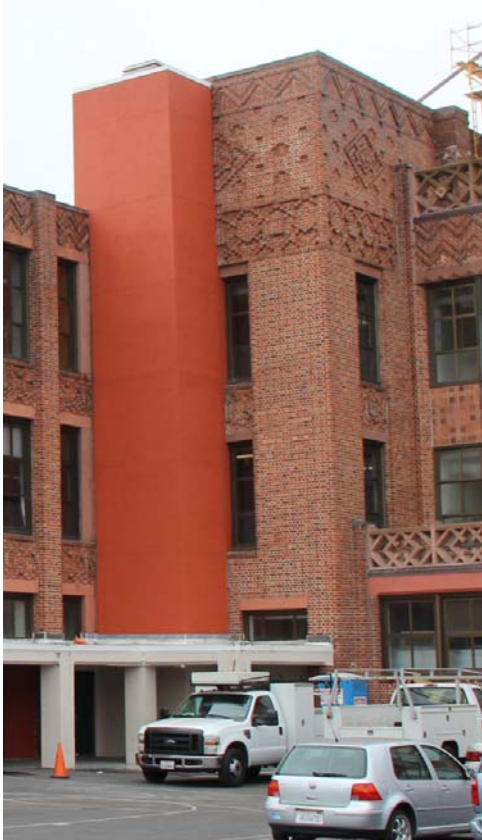
Figure 31. South tower; view toward southwest.
