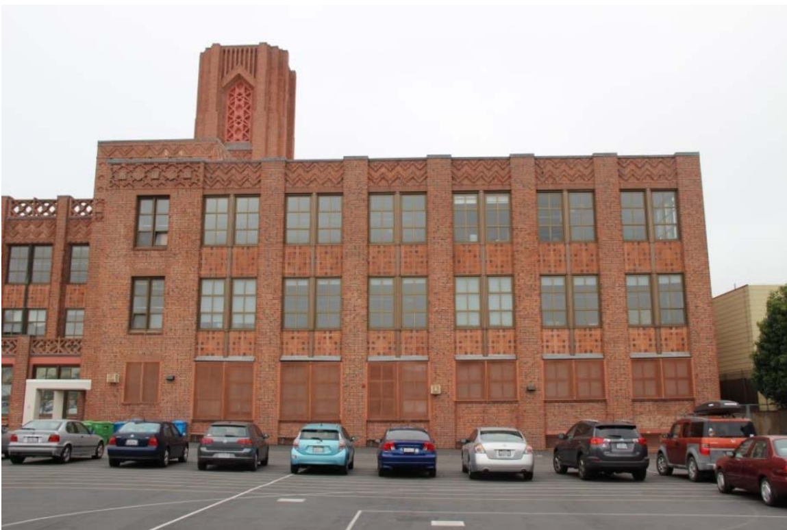
Figure 30. North section of east façade of Theodore Roosevelt Middle School; view toward west.
