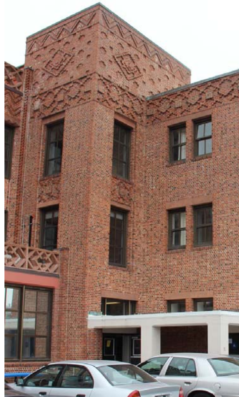
Figure 32. North tower; view toward northwest.
