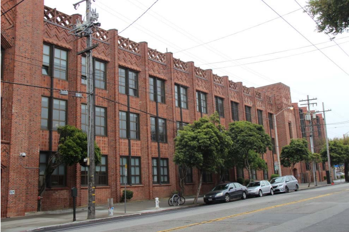
Figure 23. Academic building; view toward southeast.
