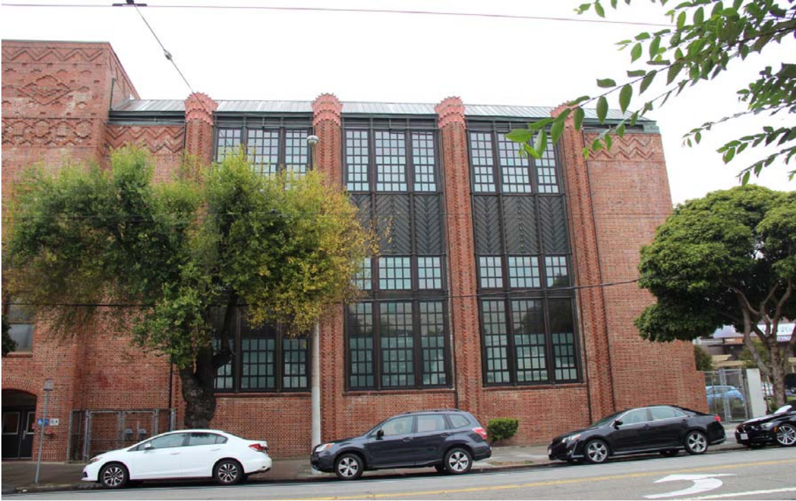
Figure 26. West façade of gymnasium wing.
