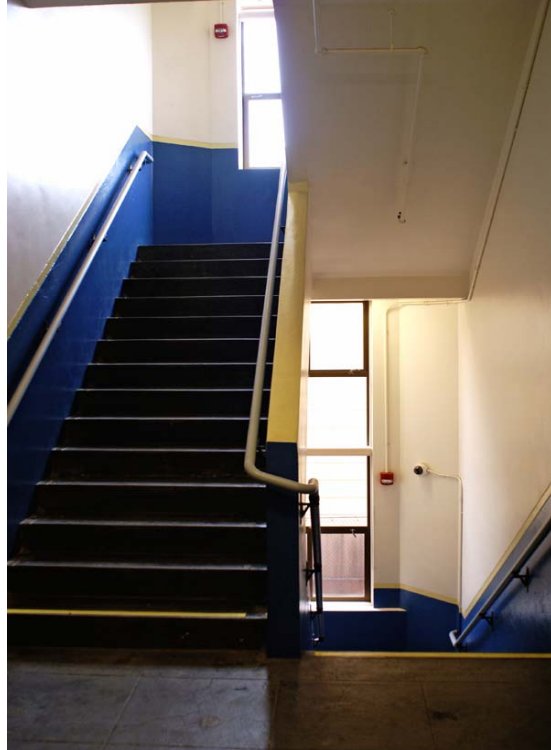
Figure 45. South stair between second and third floor levels.
