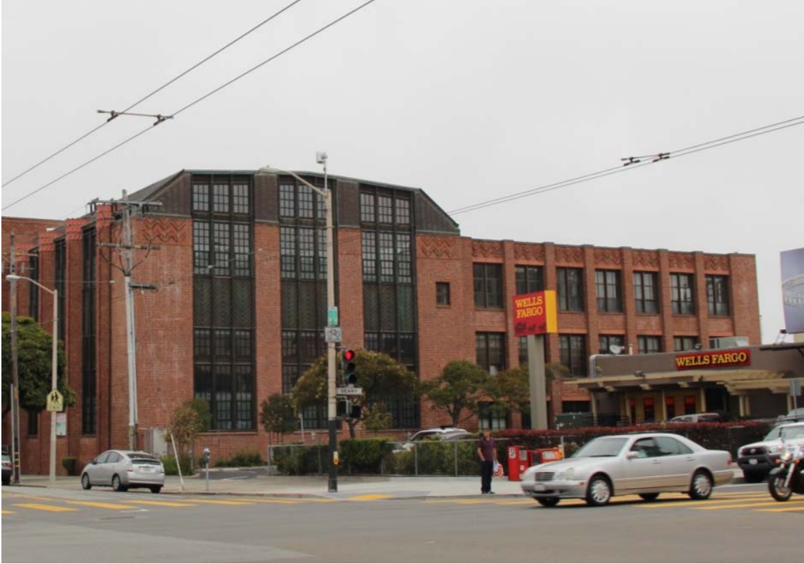
Figure 27. South façade of Theodore Roosevelt Middle School; view toward northeast.
