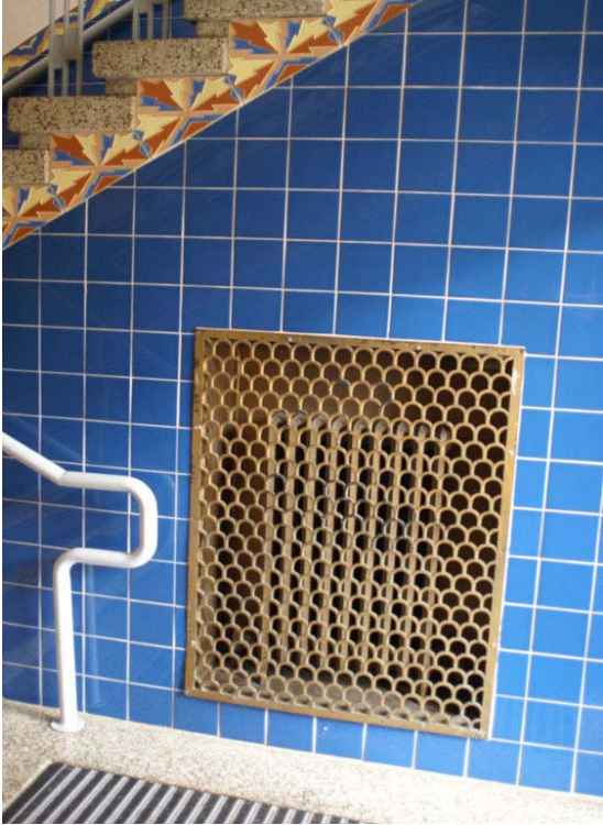
Figure 44. Tiled wainscoting and decorative metal radiator screen.
