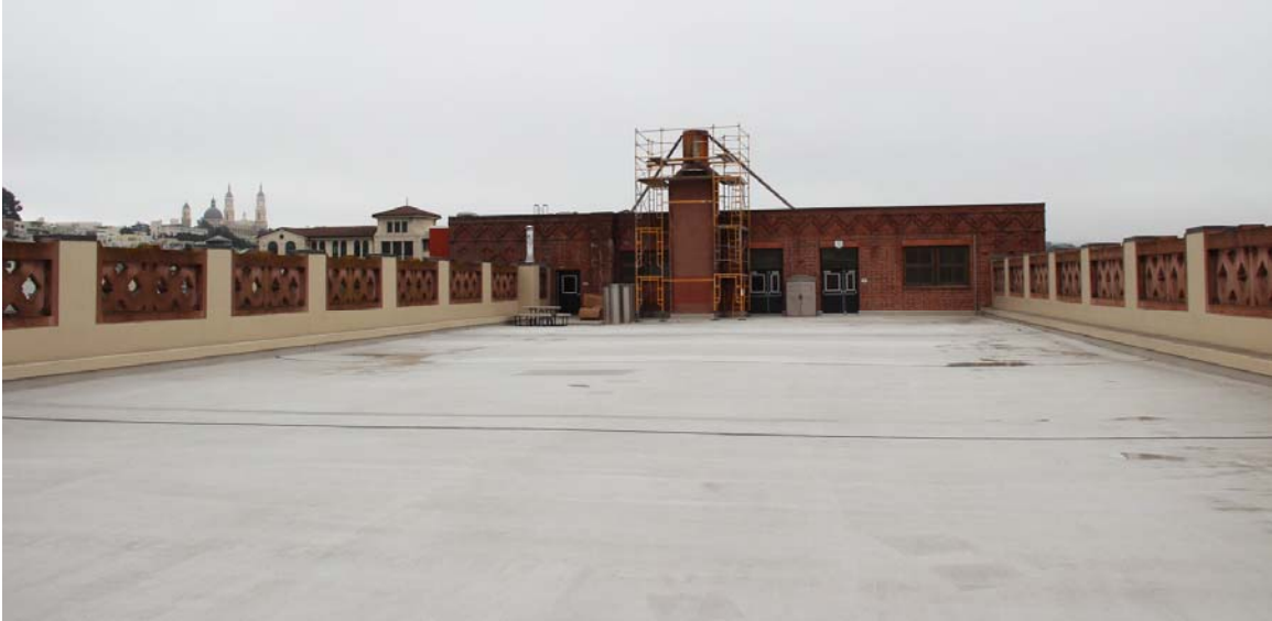
Figure 54. Rooftop play area; view toward north.
