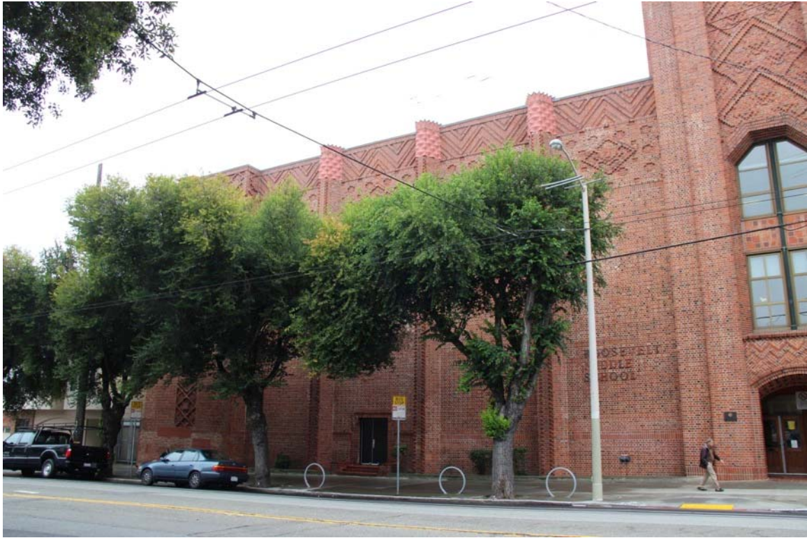
Figure 17. Auditorium wing of west façade; view toward northeast.
