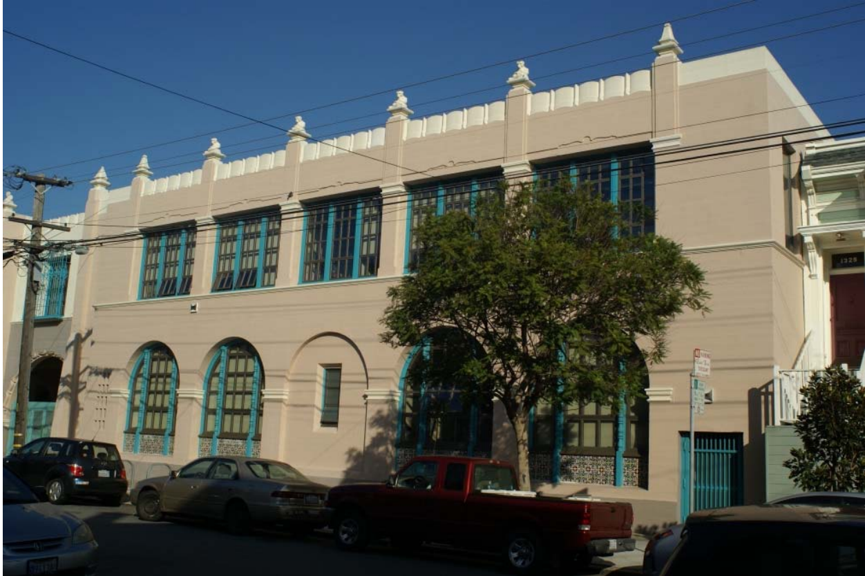
Figure 20. South part of the west façade of the former Sunshine School; view toward northeast.
