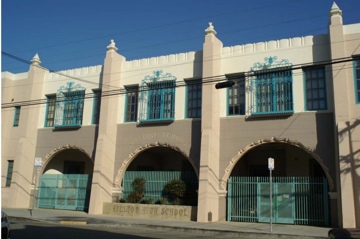
Figure 22. Central section of the west façade of the former Sunshine School; view toward northeast.
