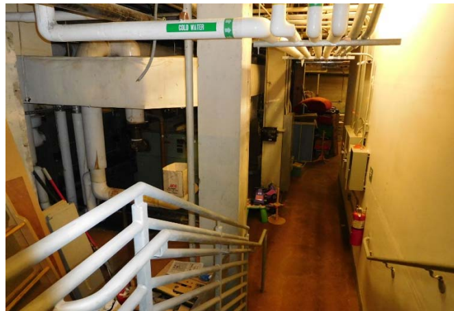
Figure 44. Basement of the former Sunshine School; view toward west.
