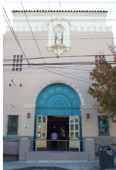
Figure 15. Entrance pavilion on east façade; view toward west.
