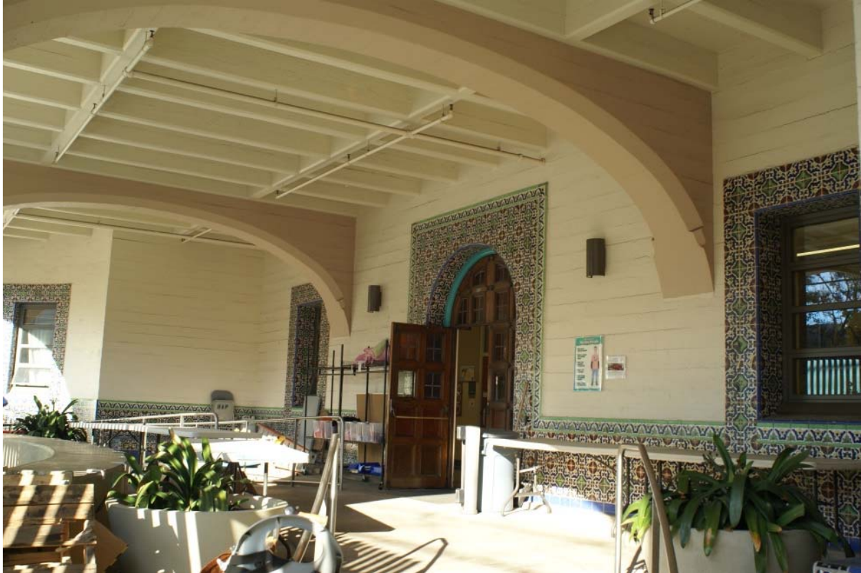
Figure 22. Driveway on west side of the former Sunshine School; view toward northeast.
