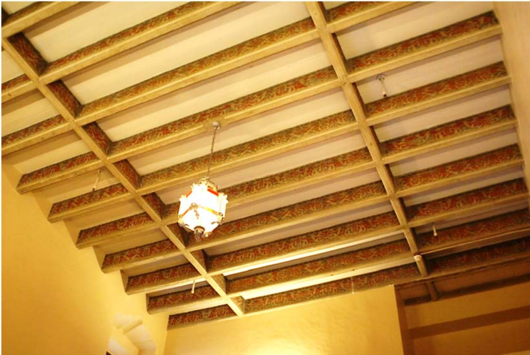
Figure 35. Ceiling of main lobby/stair; view toward north.
