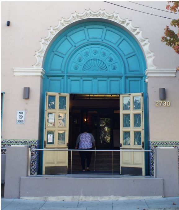
Figure 16. Detail of Bryant Street entrance.
