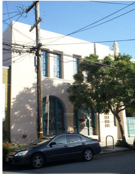
Figure 24. Northernmost part of the west façade of the former Sunshine School; view toward southeast.
