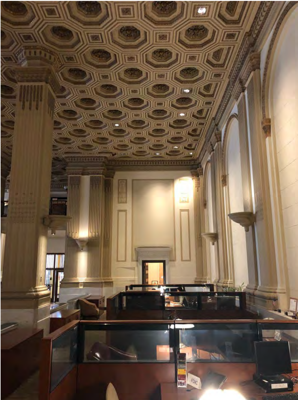
View of the office area at west end of 1920 banking hall, looking south, October 2019. Source: architecture + history, llc. (2020) report
