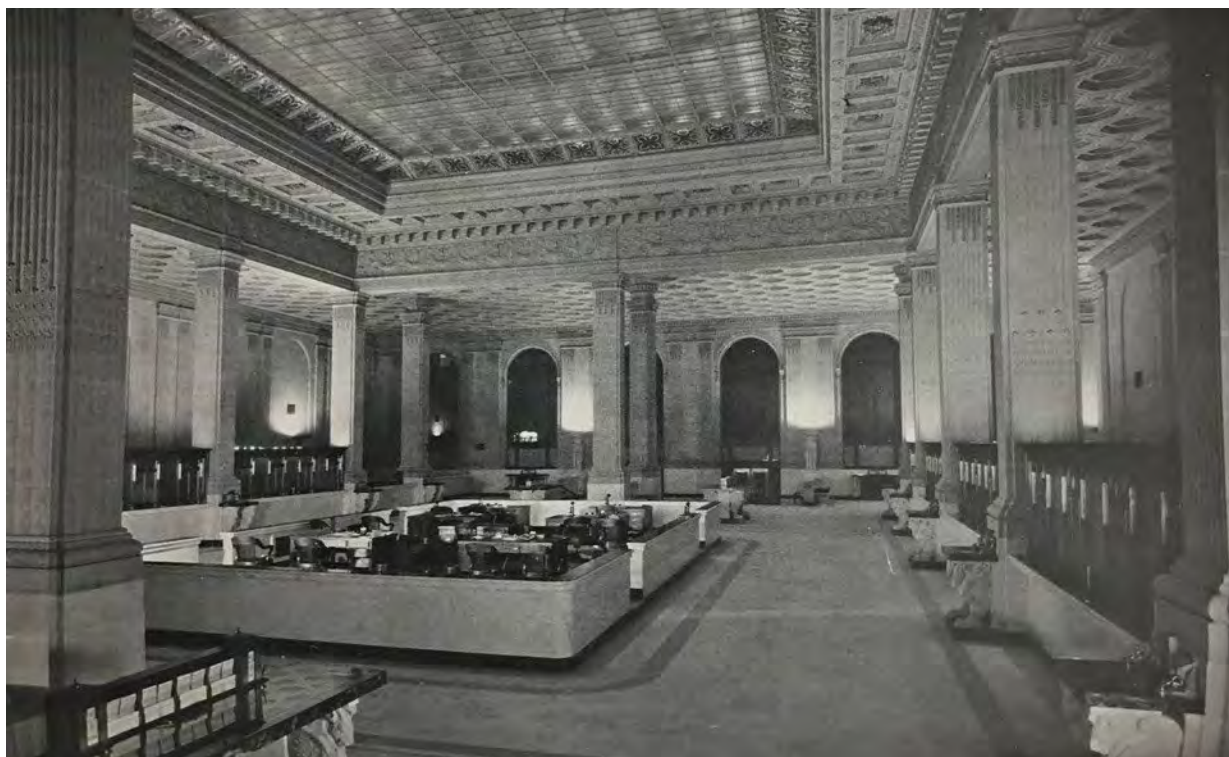
View of the 1920 banking hall, looking east, from The Architect and Engineer , October 1922. Source: architecture + history, llc. (2020) report
