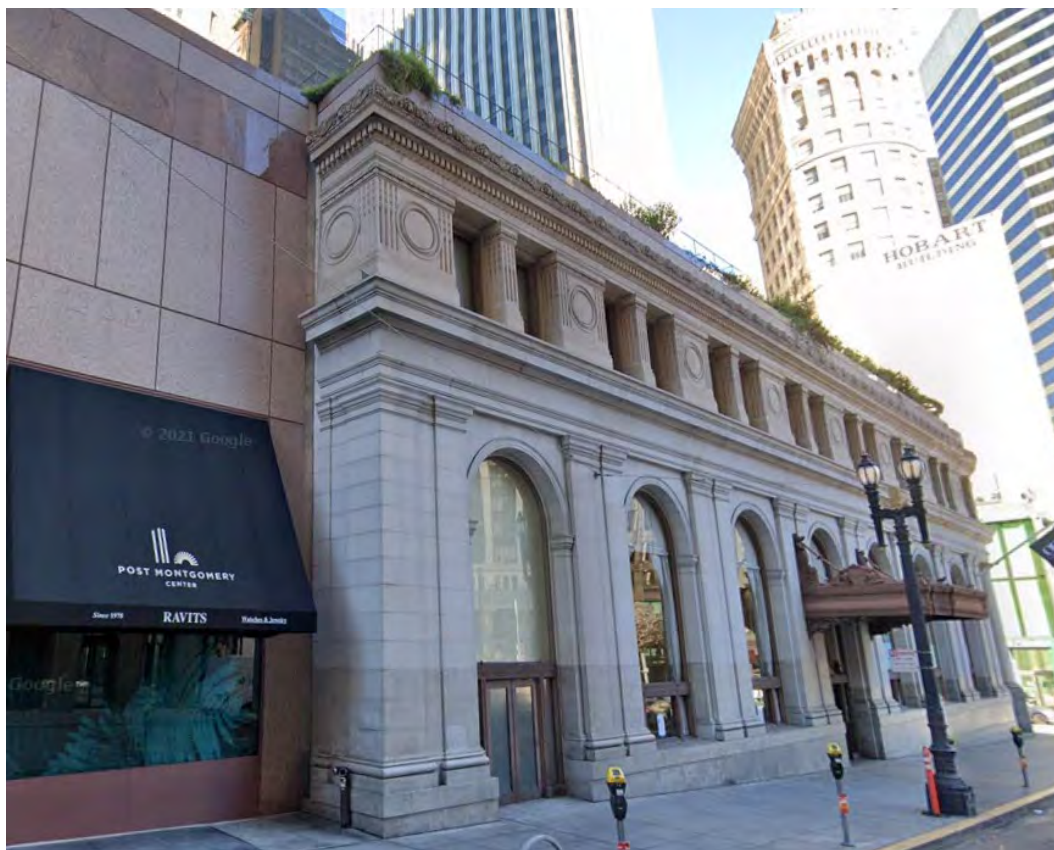
Post Street elevation where building connects to Crocker Galleria, 2020. Source: Google Streetview
