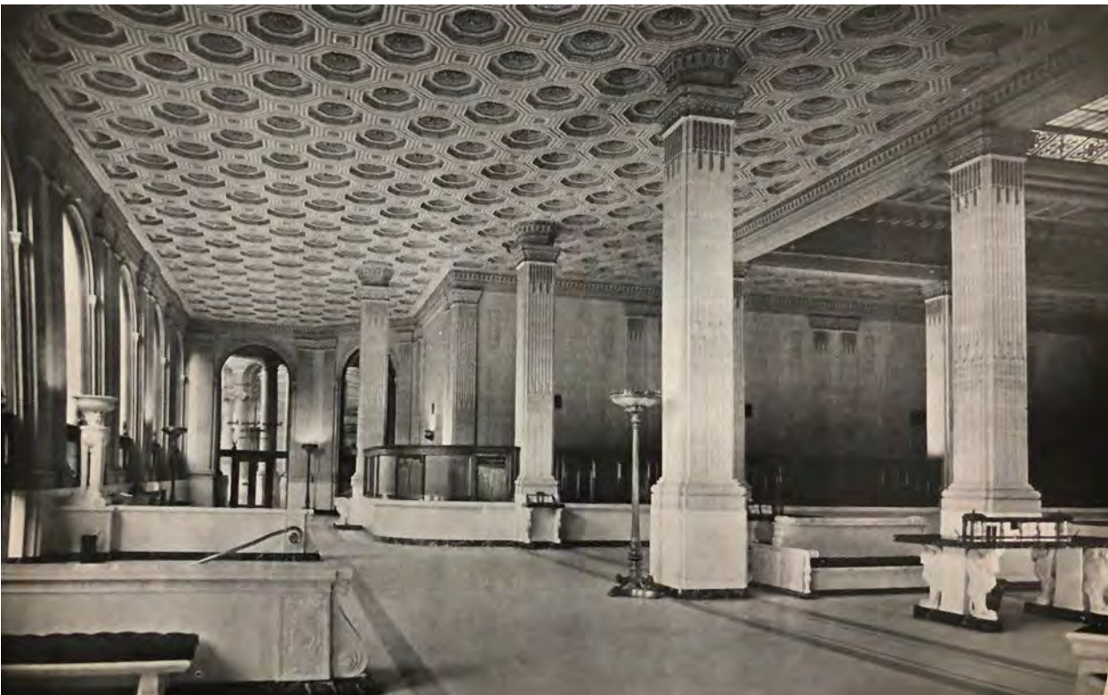
View of interior of 1920 banking hall with stair to Montgomery Street and "teller" windows/counters, looking south, from The Architect and Engineer , October 1922. Source: architecture + history, llc. (2020) report
