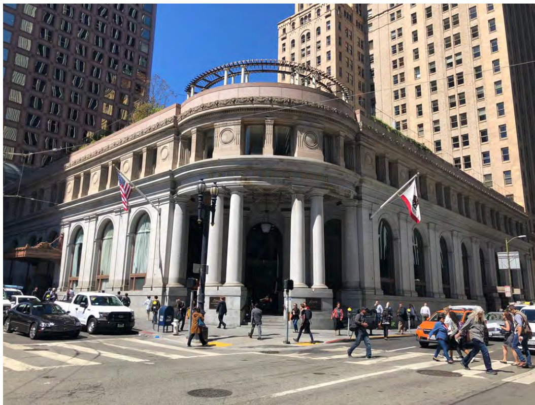
One Montgomery Street, October 2019. Source: architecture + history, llc (2020) report
