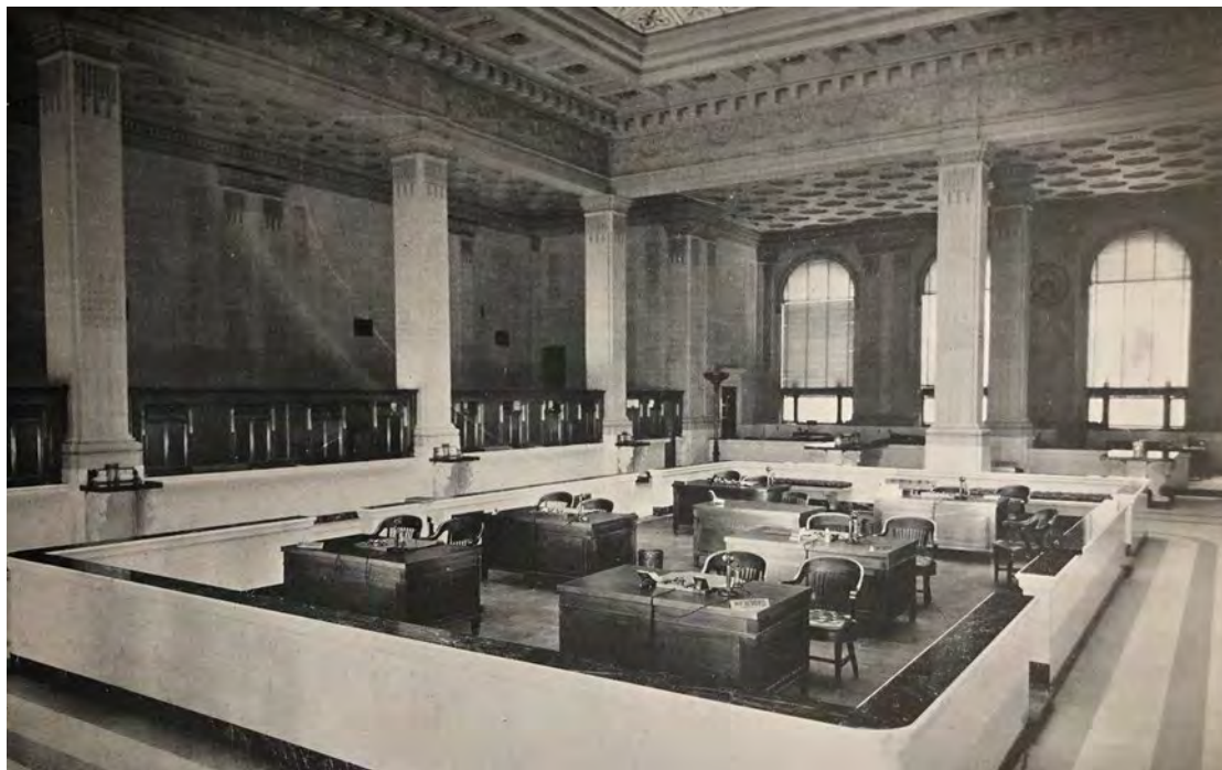
View of 1920 banking hall addition, looking southwest, from The Architect and Engineer , October 1922. Source: architecture + history, llc. (2020) report
