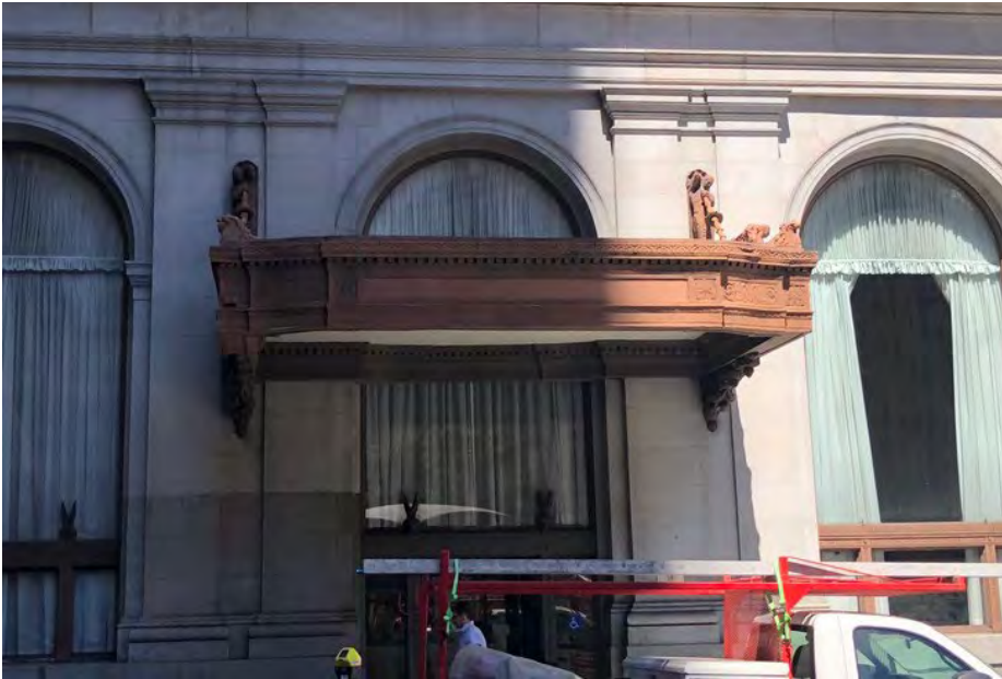
Canopy at Post Street entry, October 2019. Source: architecture + history, llc. (2020) report
