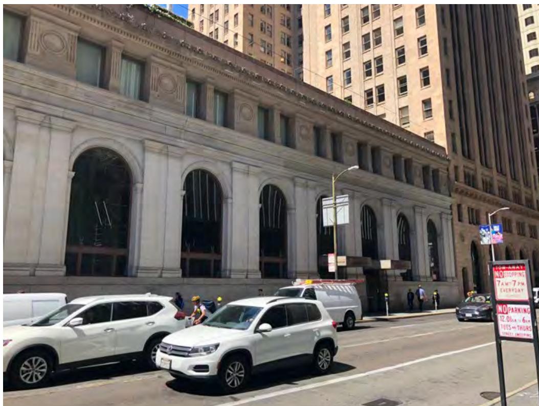
Montgomery Street elevation, view northwest, October 2019. Source: architecture + history, llc (2020) report
