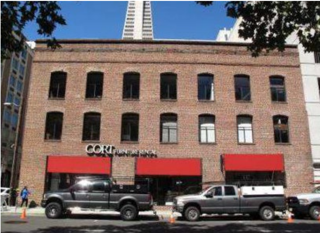
447 Battery Street primary (east) façade, 2017. Source: Page & Turnbull, Inc. (2017) report
