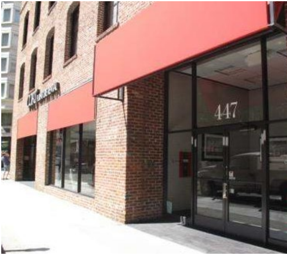
Storefront, east elevation, 2017. Source: Page & Turnbull, Inc. (2017) report
