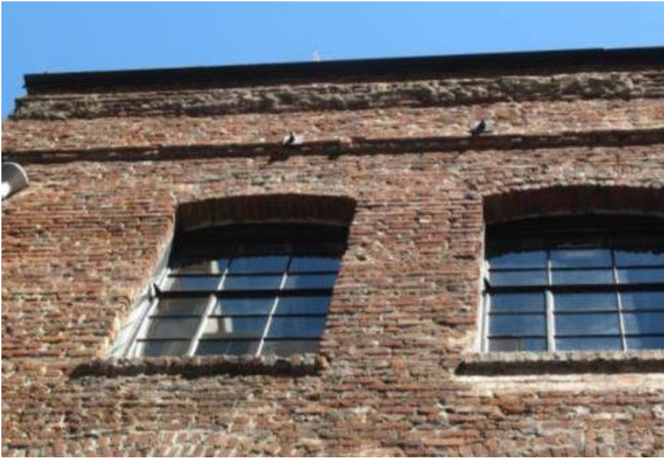
Upper level windows, south elevation, 2017. Source: Page & Turnbull, Inc. (2017) report
