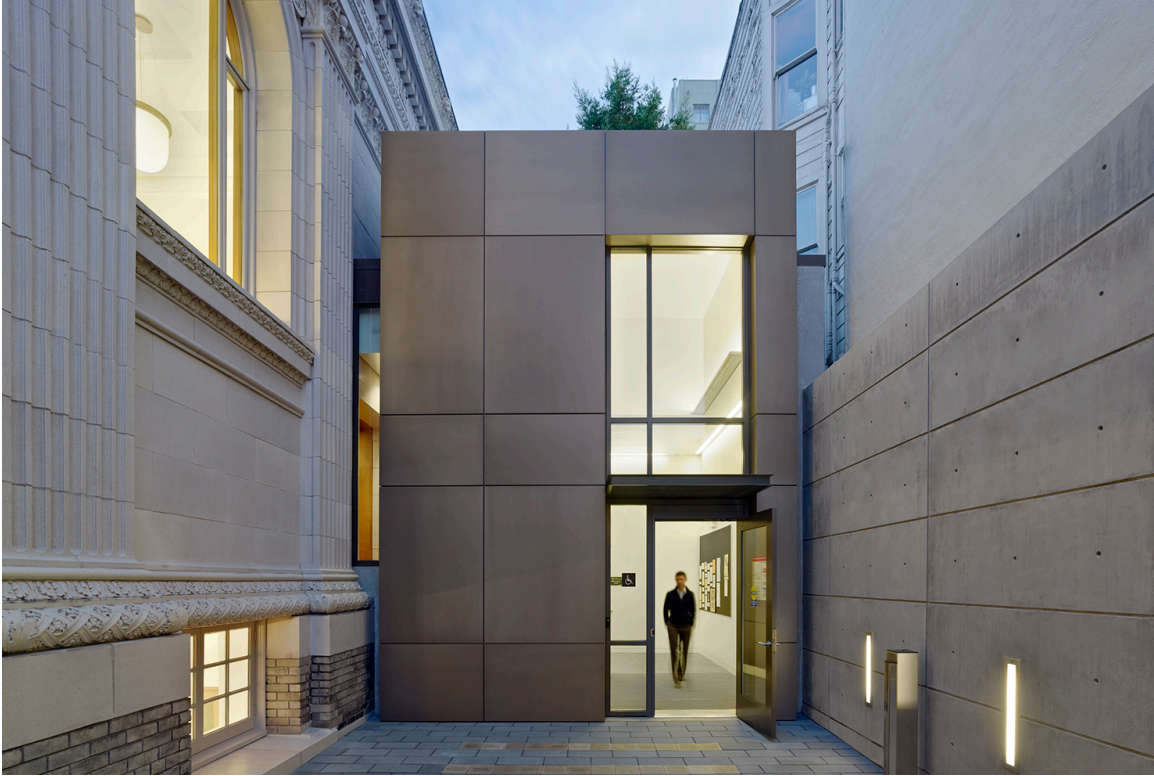
Above: Golden Gate Valley Branch Library, looking south, detail of small addition to the west of original building , 2012 after renovation. (Source: TEF Design).
