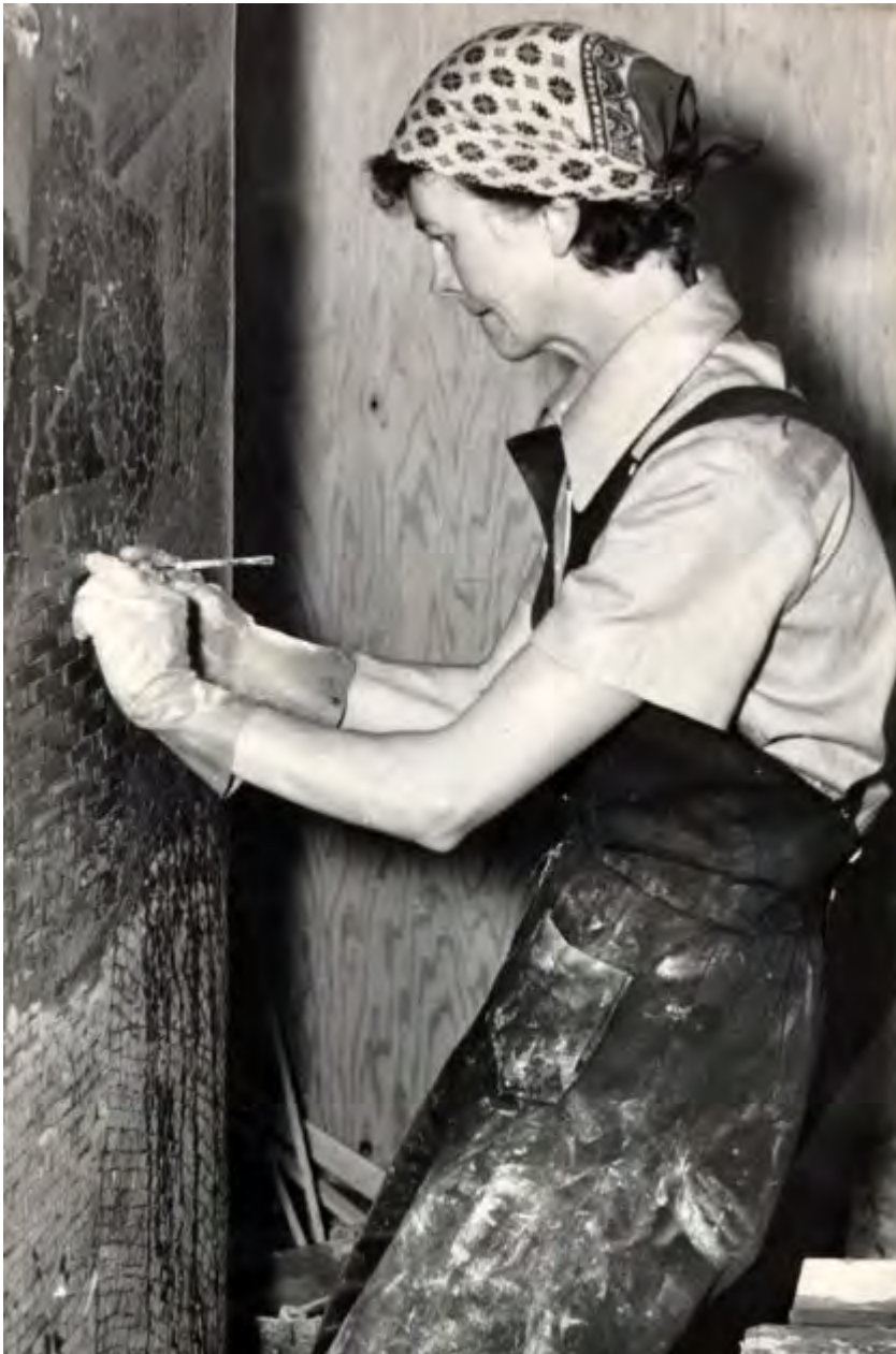
Helen Bruton installing a tile mosaic, May 20, 1937.
