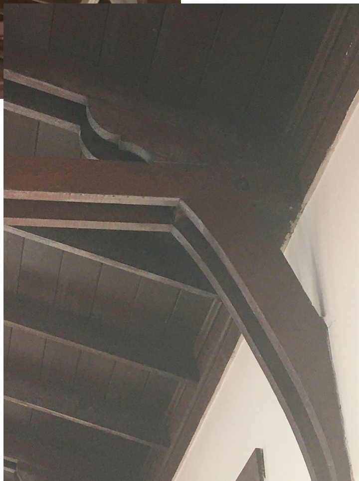
St. James Presbyterian Church, details of ceiling, trusses, and brackets in sanctuary, 2022 Source: San Francisco Planning Department
