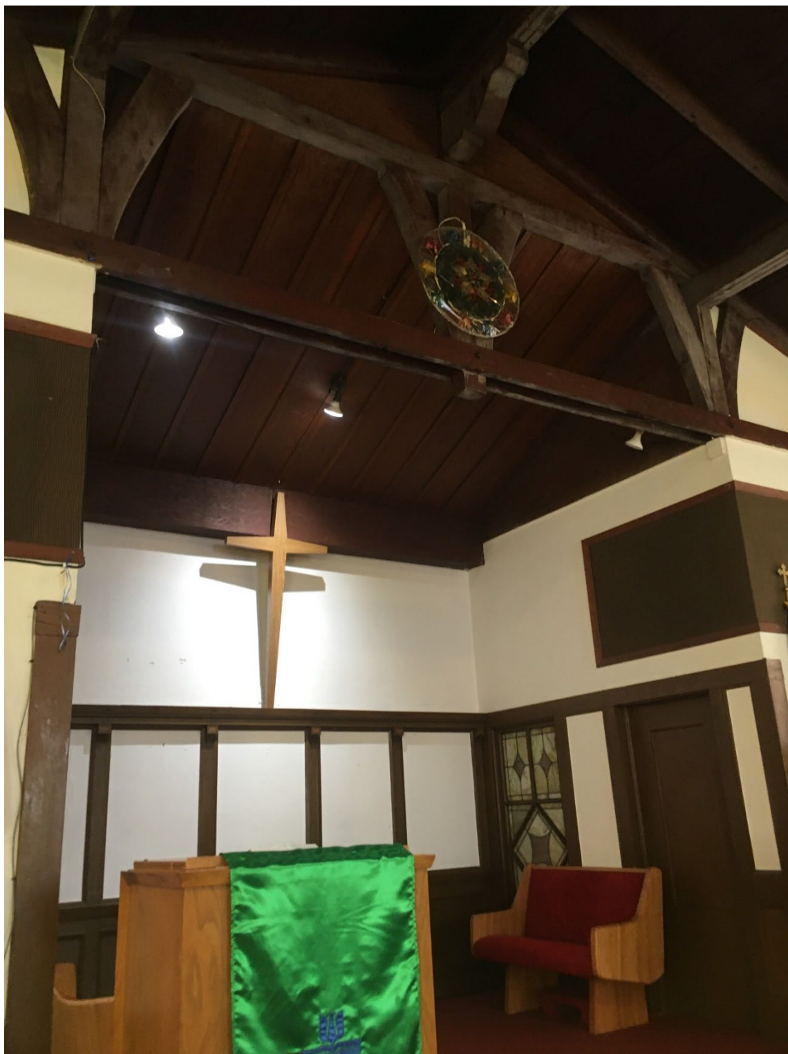
St. James Presbyterian Church, raised platform area at north end of sanctuary, view northeast, 2022 Source: San Francisco Planning Department
