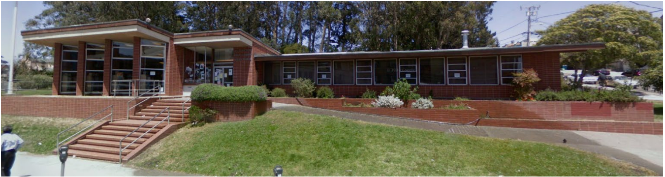
Parkside Branch Library, front façade, view north, 2008.
