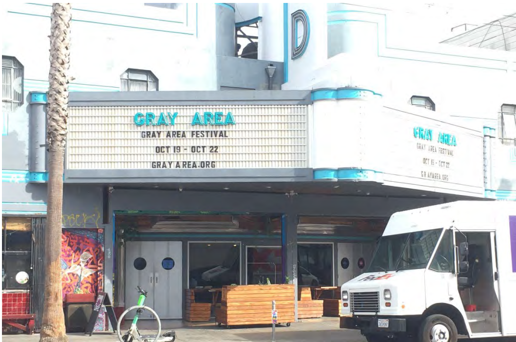
Grand Theater, marquee and entrance vestibule, view east, 2023. Source: SF Planning Department
